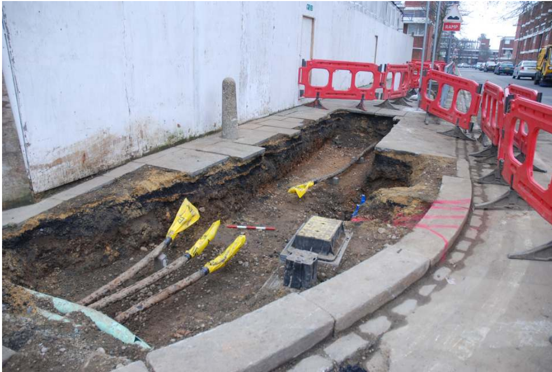
Fig. 9: Photograph of pit 5 on Polthorne Grove.
