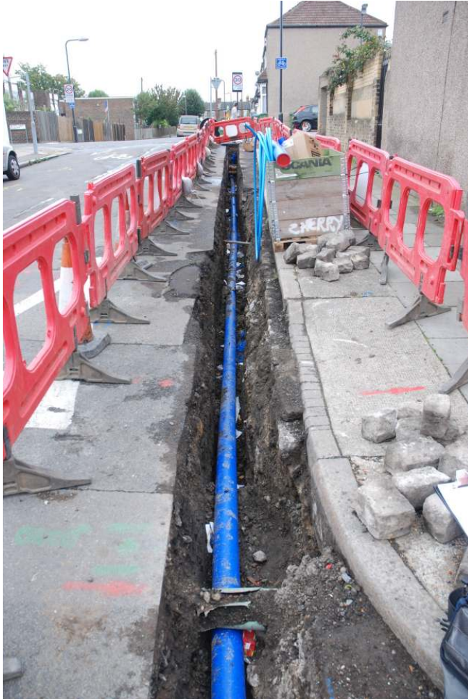
Fig. 11: Photograph of the open-cut trench along Hartville Road, looking west (trench 1).
