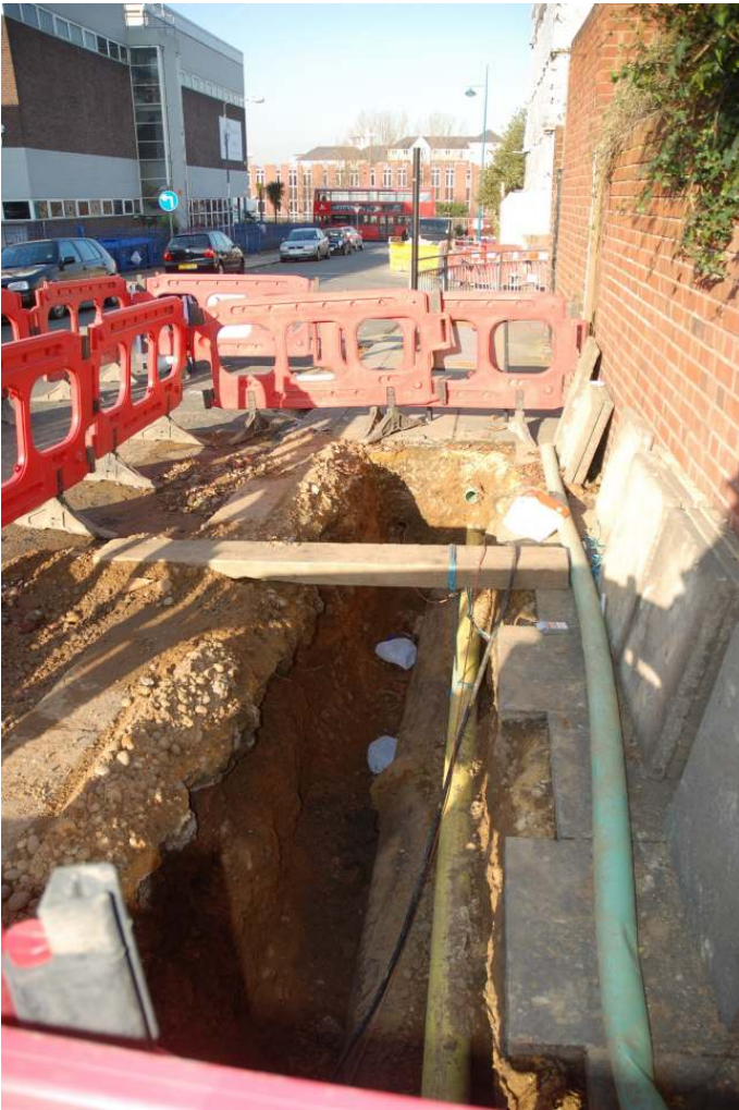
Fig. 7: Photograph of pit 2 on Villas Road, looking north towards Plumstead Road.
