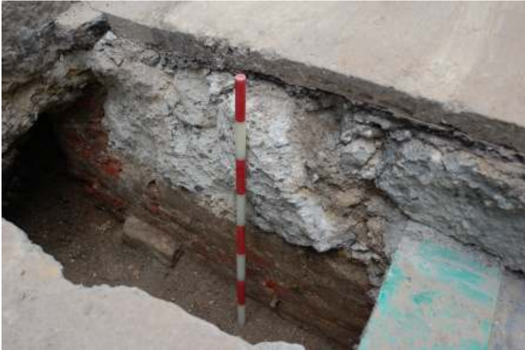
Fig.43: Wall projecting into Leadenhall street on alignment with Hartshorn Alley, facing SW. 4 th October 2011
