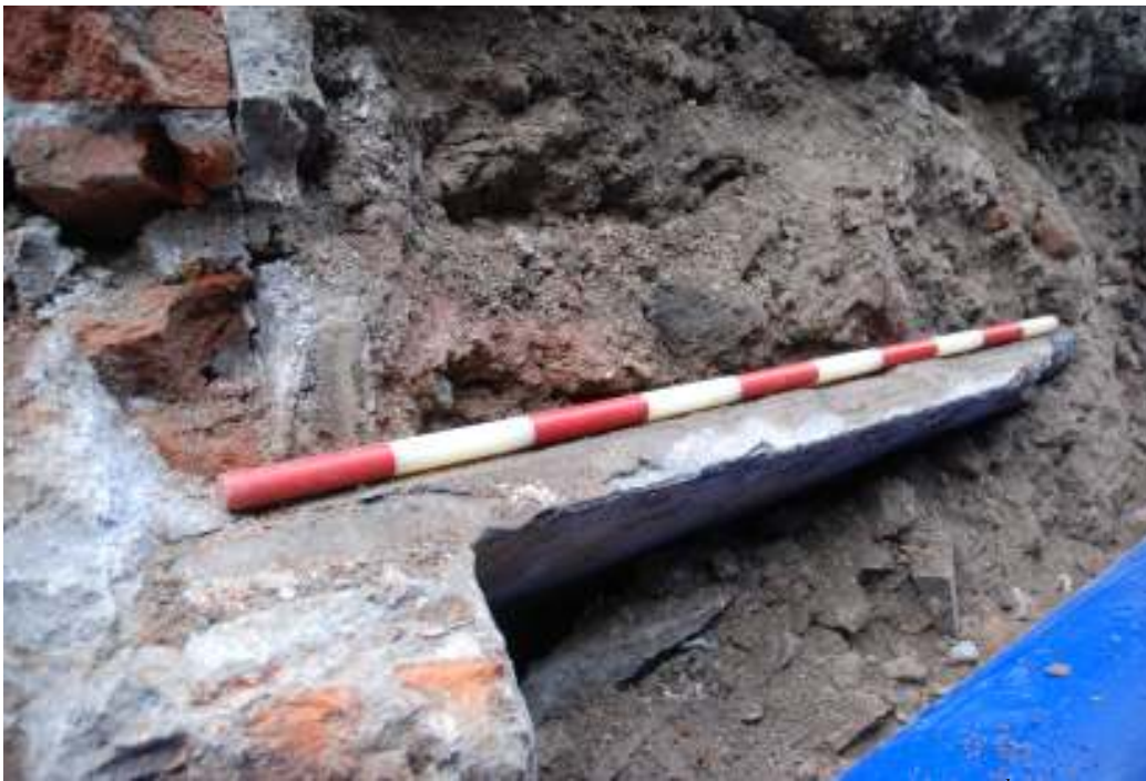
Fig.45: Sloping, concrete roof of cellar, facing SSW. Leadenhall Street 11 th October 2011
