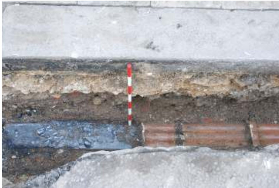
Fig.16: Shot of south section of trench along Aldgate High Street. Facing S
