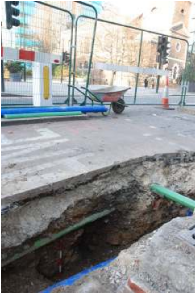
Fig.22: Wall in trenching looking towards St.Botolphs Without, facing NE
