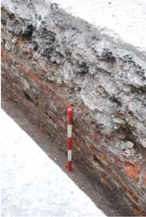
Fig.51: Timber holes in wall, detail of fig.49, facing NE, 13 th July 2011, (0.5m scale)
