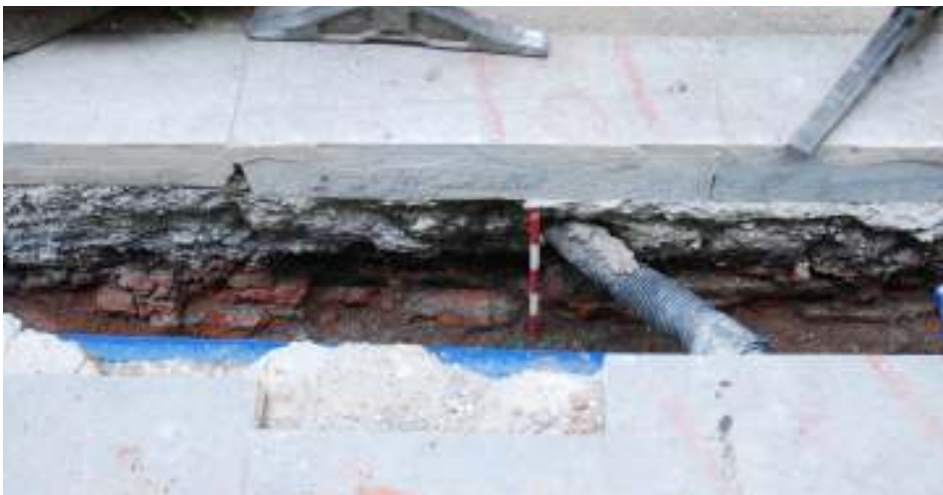
Fig.41: Brickwork in trench along trench, Fenn Court 3 rd November 2010, Facing W
