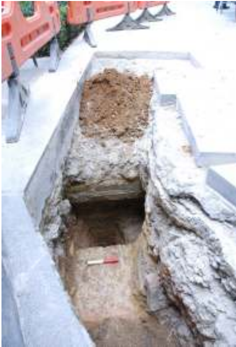
Fig.39: 'Cavity' wall / drain in Fenn Court. Facing NE, (0.2m scale)
