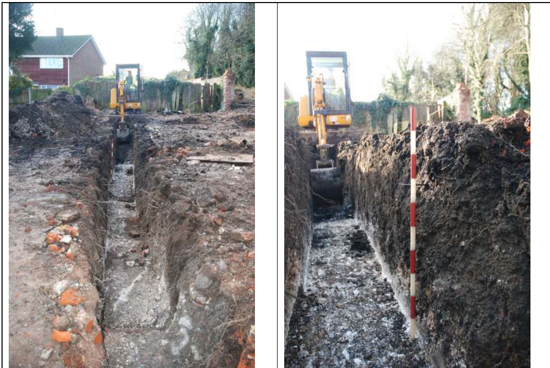
Fig 28 Excavation of the southernmost footing, an extension to Trench 2 running east-west. Only natural hillside accumulated garden soil deposits were encountered in this footing and natural chalk at a depth of -0.6m at the eastern end falling to a maximum depth of -1.2m deep at the far western end of the footing (right).
