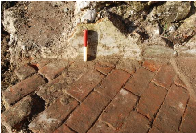
Fig 17 Detail of the dry-laid brick floor, in an on-bed running or stretcher bond. The bricks are noticeably thin, red/brown in colour, with measurements of approximately 215mm (l) x 110mm (w) x 38mm (b). The brick floor has clearly been cut through for the construction of the garden wall (mainly constructed of stone in this area), which is shown behind the 20cm scale, with a plastered face on the interior of the ‘lean-to’ structure. Brick samples from this floor conform to London Fabric Series classification [3047], with a date range of c.1700 to c.1850. The brick samples from the apsidal ended wall are bright orange red in colour and measure 210mm x 112mm x 55mm and are of fabric series [3047], dating to c.1700 to c.1850. The floor clearly abuts the apsidal ended wall to the south and is stratigraphically later than the wall, although both features may be broadly contemporary in date.
