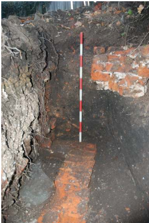
Fig 24. The small brick building at the westernmost end of footing Trench 1 (to the left of 1m scale), just below and to the south of the brick foundation for the garden wall (to the right of the scale and constructed in bright red brick with a concreted greyish white thick lime mortar in this location). Image looking west, scale 1m, the base of the structure is at +87.8m AOD.
