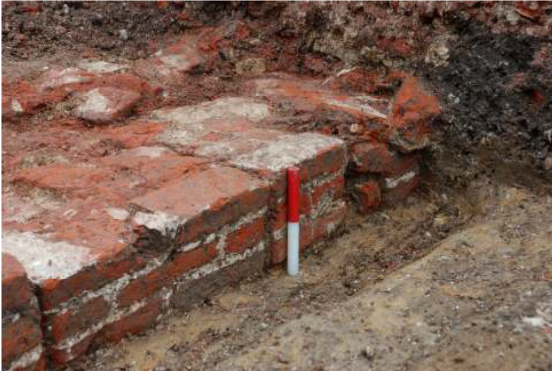
Fig. 67: Close-up photograph of the northern end of wall (43). This shows that the wall was made up of chunks of re-used brickwork.
