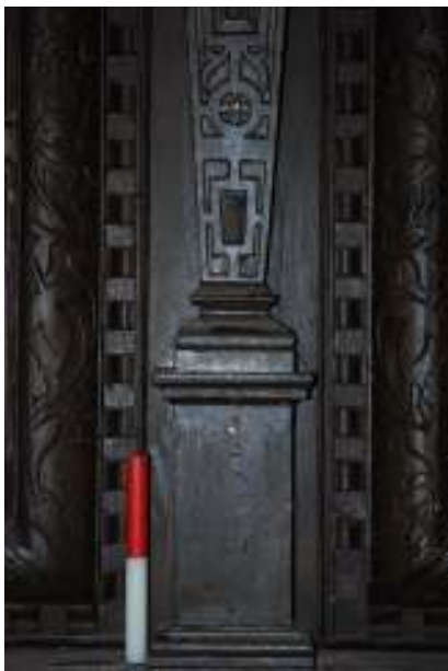
Fig. 174: Photograph of the Roman Doric columns, on pedestals, on the entrance hall fireplace.
