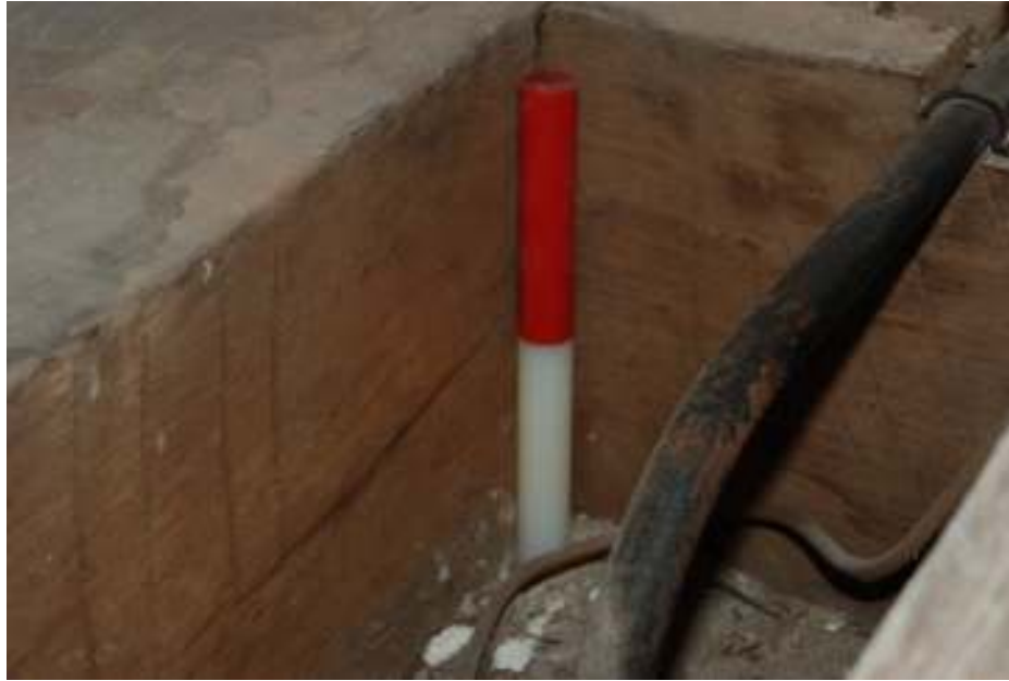
Fig. 147: Carpenter's marks in Room F21.
