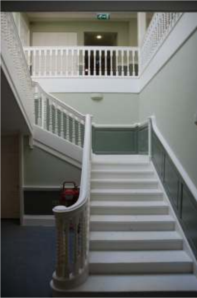
Fig. 179: Photograph of the staircase, after restoration. The new balusters along the western side of the first floor, inserted by Clancy, can clearly be seen.
