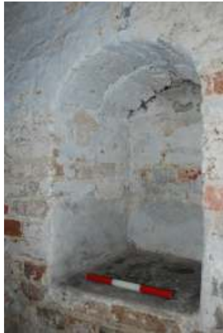
Fig. 105: Photograph of the open niche on the southern wall of the passageway through into the main part of the cellar.
