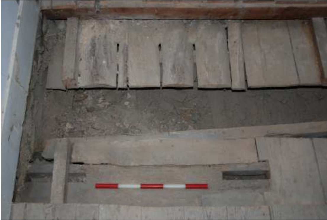
Fig. 134: Pine skins in room S7, timber 1 in lower half of shot with empty mortise joints. Facing west (0.5m scale).
