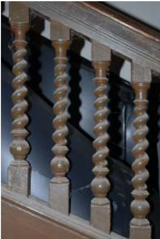
Fig. 180: Close-up photograph of the barley-twist balusters.
