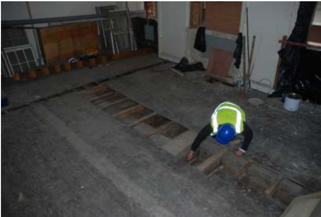
Fig. 122: Inspecting timbers in room F7.
