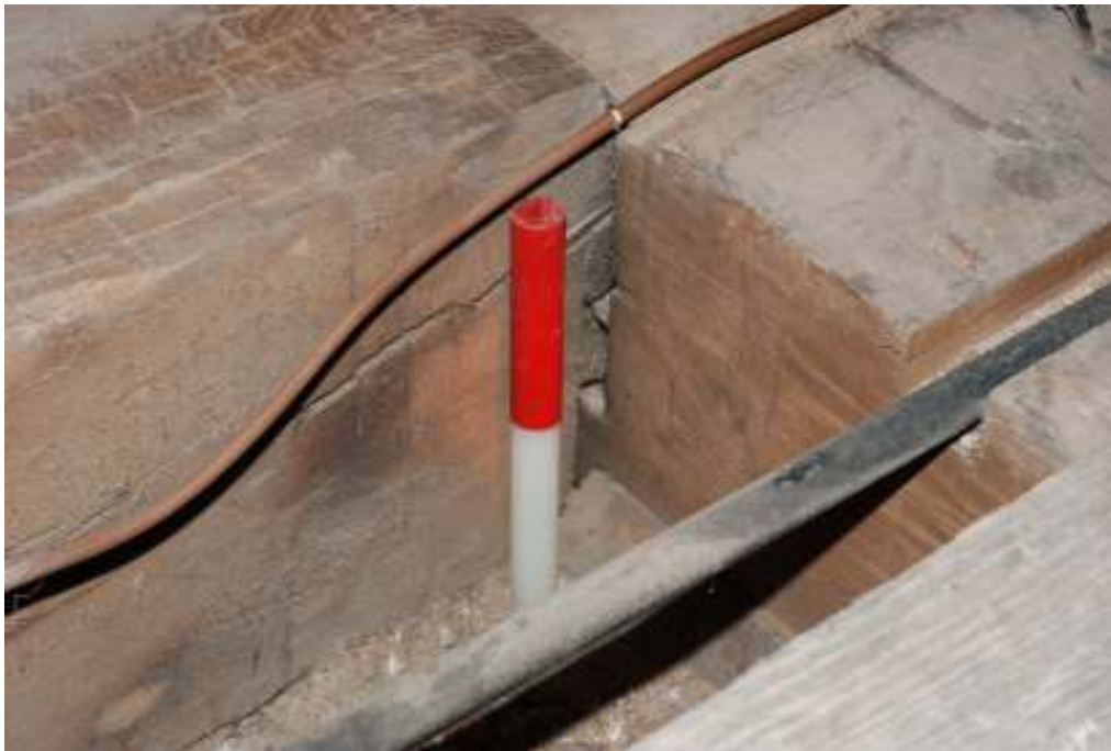
Fig. 146: Photograph of timber 5 and the adjacent beam to the left (room S20), looking south-west and showing carpenter's marks (0.2m scale).
