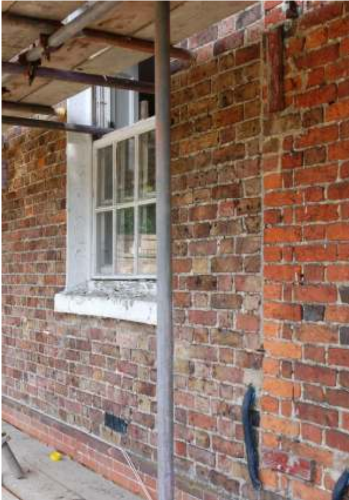
Fig. 32: Close-up photograph of the abutting line of brickwork on the southern frontage, representing the original south-western corner of the earlier 17 th Century house.
