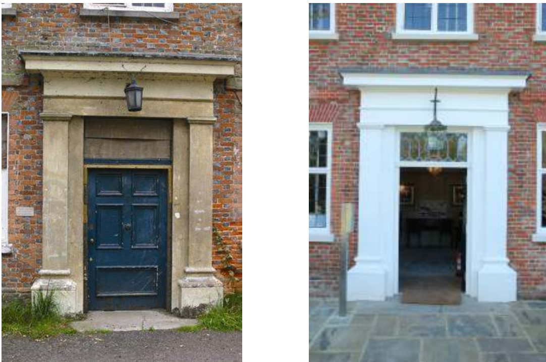
Fig. 25: Photographs of the door today – taken before and after restoration.
