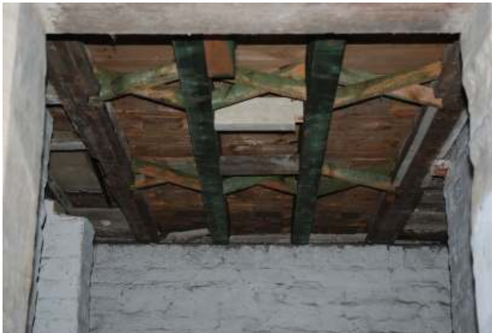
Fig. 120: Photograph of the ceiling of the cellars.
