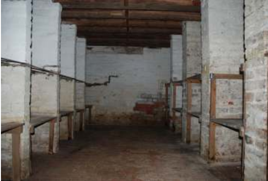
Fig. 114: Photograph of the southern-most room of the cellars. The different bays / shelves on either side can clearly be seen.
