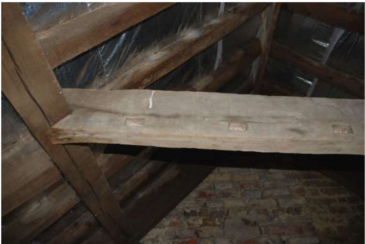
Fig. 69: Re-used timber above north-eastern part of room S13. The earlier mortices are visible.
