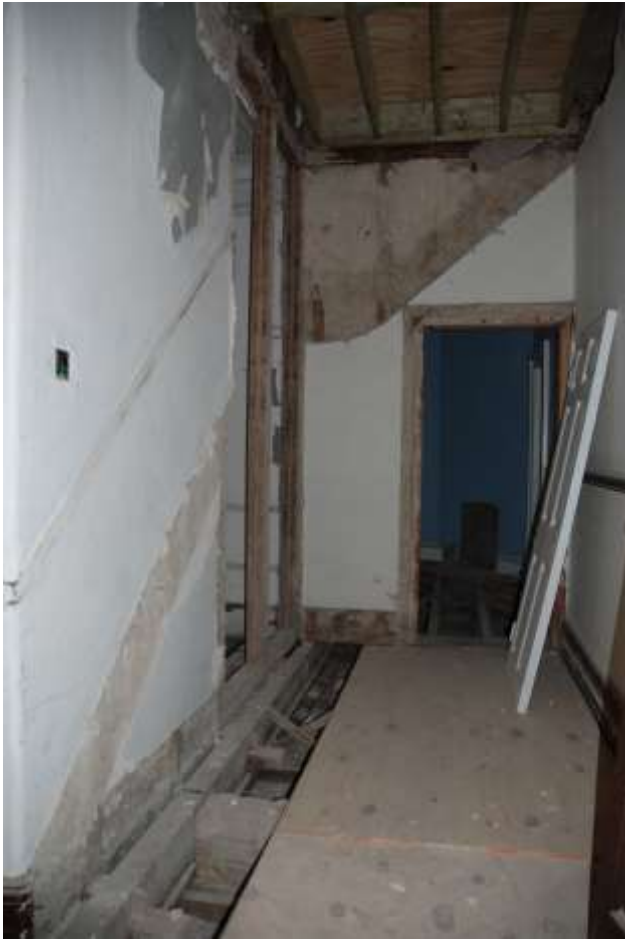
Fig. 219: Outline of the staircase from first to second floor in the area of Captain Tarleton's eastern extension (now removed).
