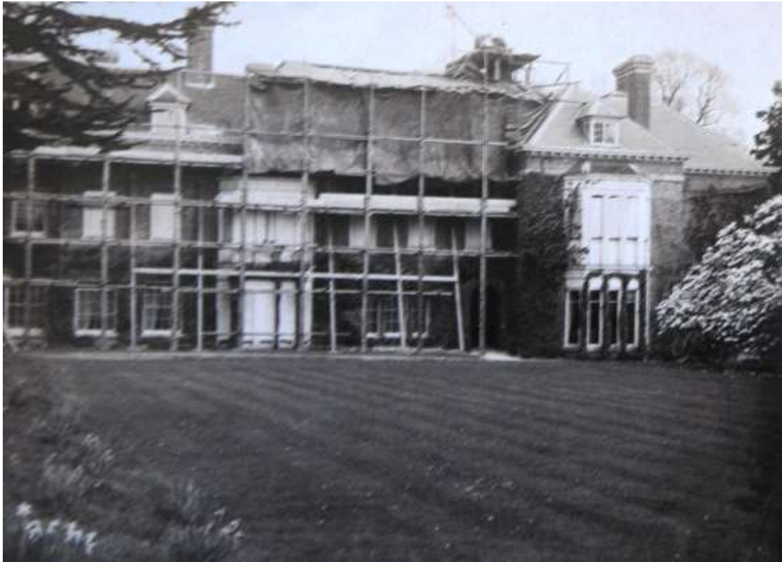
Fig. 251: Photograph of the repair works undertaken in 1924-25, southern frontage. © Christopher Fagan.
