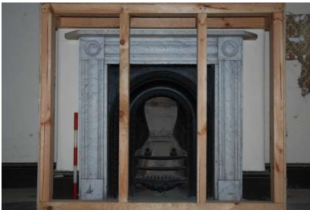
Fig. 224: Fireplace in room S5.
