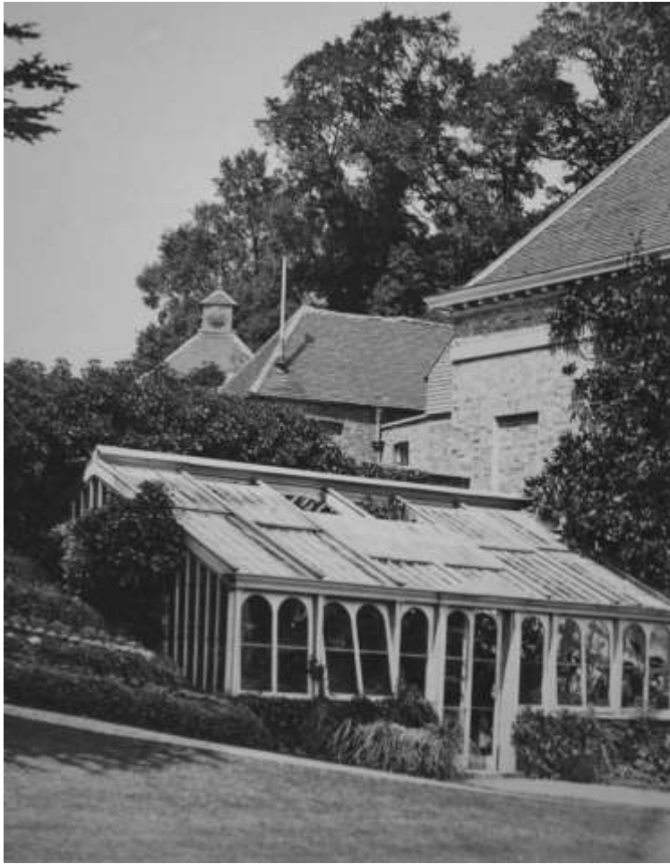
Fig. 137: c.1900 photograph with the roofs of the stables visible between the main house and the dovecote. © Christopher Fagan.
