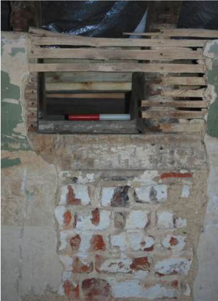
Fig. 96: Close-up photograph of some of the original lime-washed brickwork of the engine room, below later lath and plaster and rendering.
