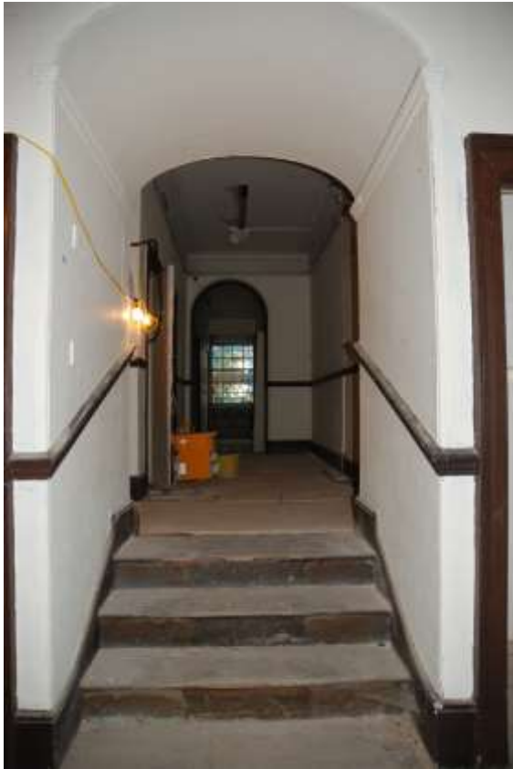
Fig. 227: Stairs on the first-floor, leading up into the area of the eastern extension, and reflecting the raised floor / ceiling level in this area.
