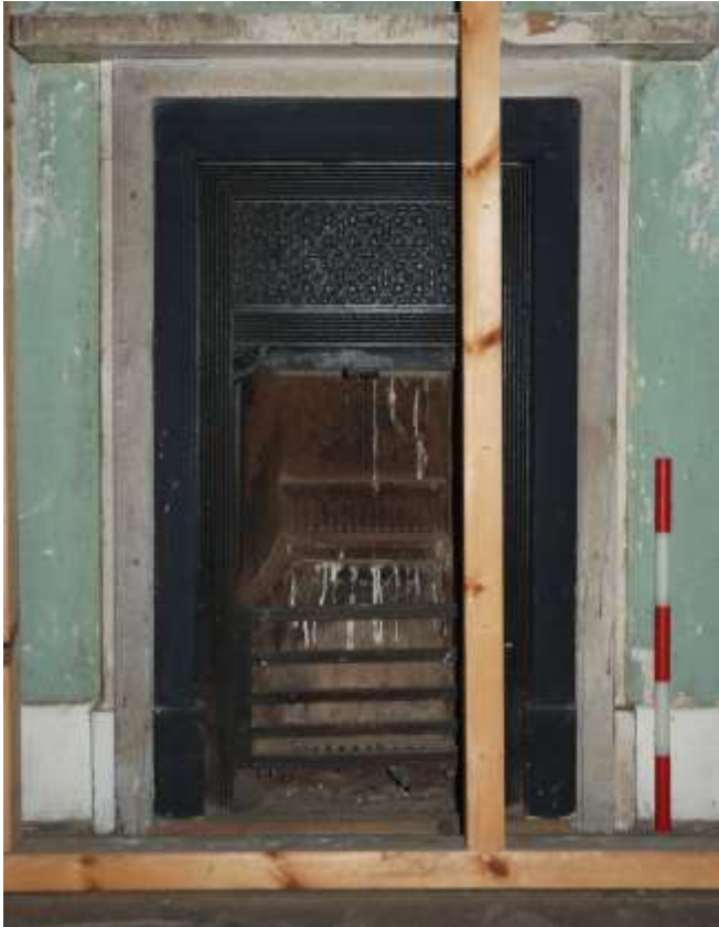
Fig. 131: Fireplace in room S9.
