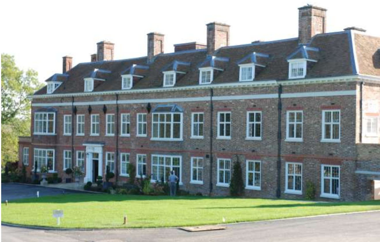
Fig. 42: Northern frontage of Breakspears. The later (greyer) brickwork of Partridge's rebuild can be seen the whole way along, above the top of the first-floor windows.
