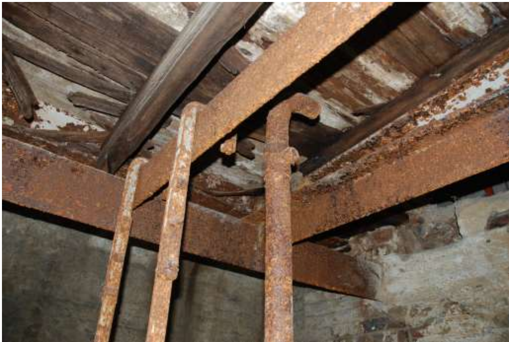
Fig. 115: Photograph of the ladder hooked over the lower-level girders.
