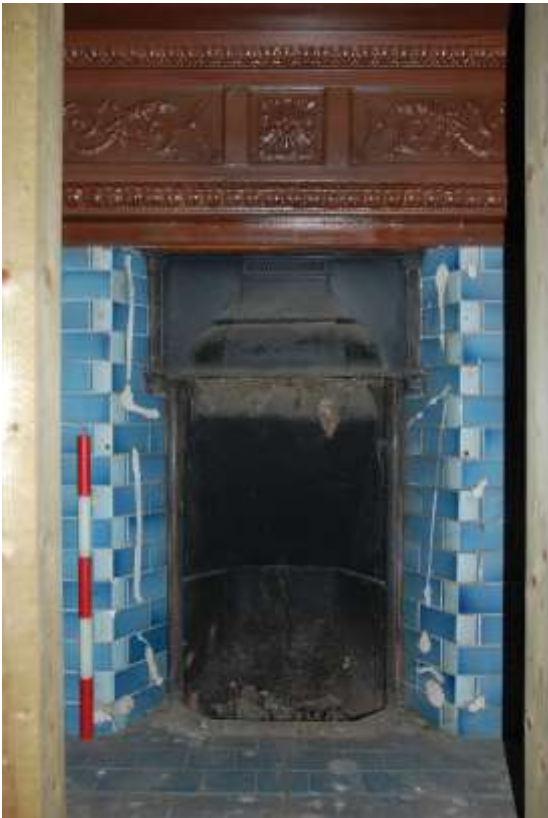
Fig. 180: Detail of the grate of the eastern fireplace in the Drawing Room.
