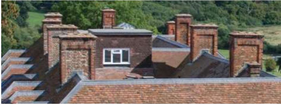
Fig. 46: Photograph of some of the chimneys, looking east.
