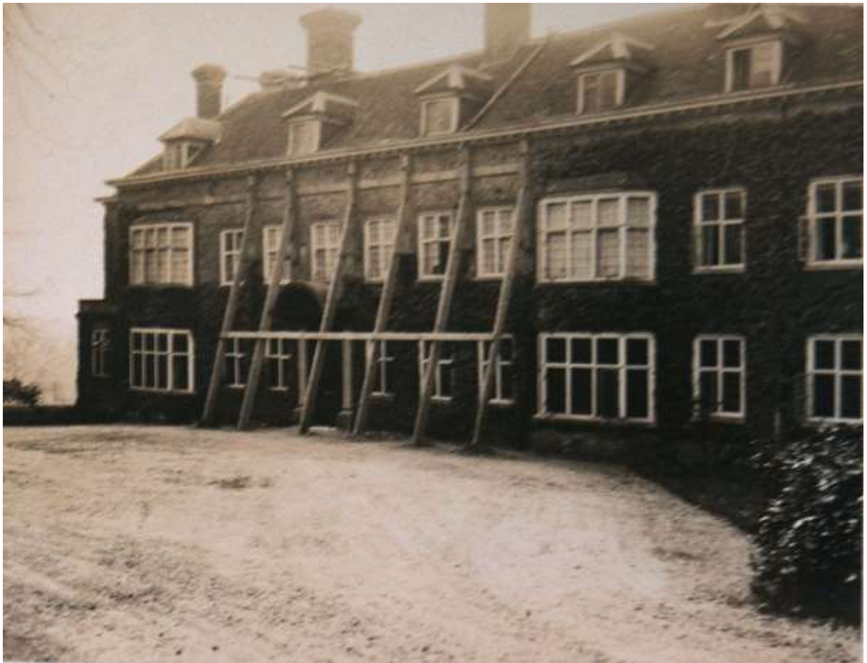
Fig. 250: Photograph of the repair works undertaken in 1924-25, northern frontage. © Christopher Fagan.
