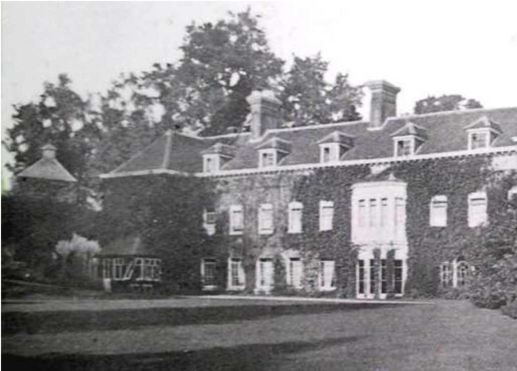
Fig. 232: 1911 photograph depicting the smaller conservatory / garden house.
