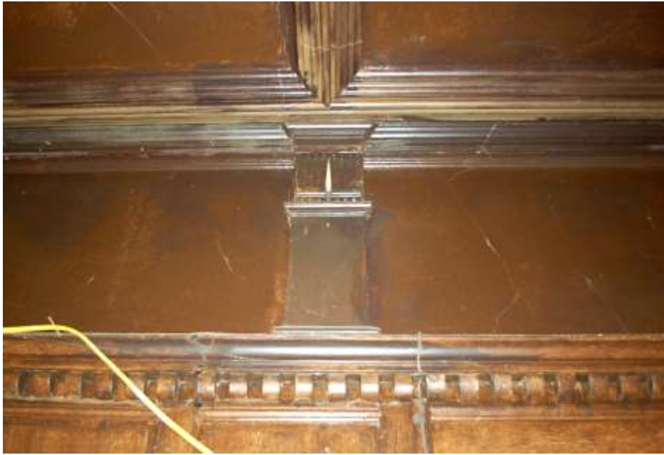
Fig. 125: Entrance Hall – wall above panelling (G22).
