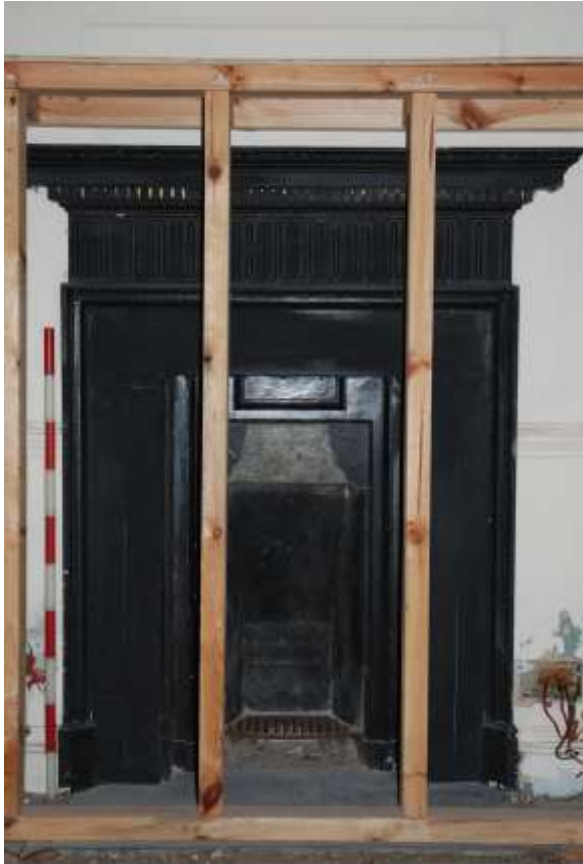
Fig. 214: Fireplace in the Blue Bedroom Dressing Room (F3).
