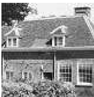
Fig. 269: Extract from 1974 photograph, depicting the demolished chimney (between the two dormer windows).
