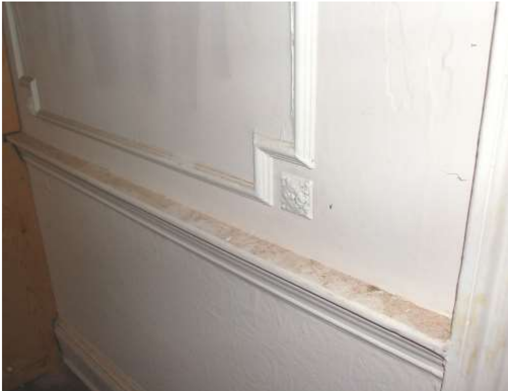
Fig. 297: Beading and plastic corner moulding forming one of a number of wall panels in the drawing room (G1).
