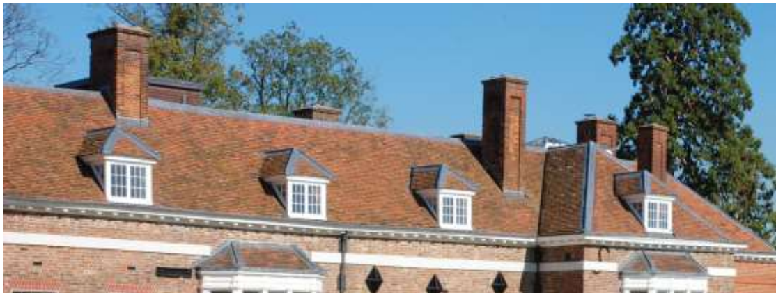
Fig. 258: Photograph of the chimneys today, without their ‘capped’ tops.
