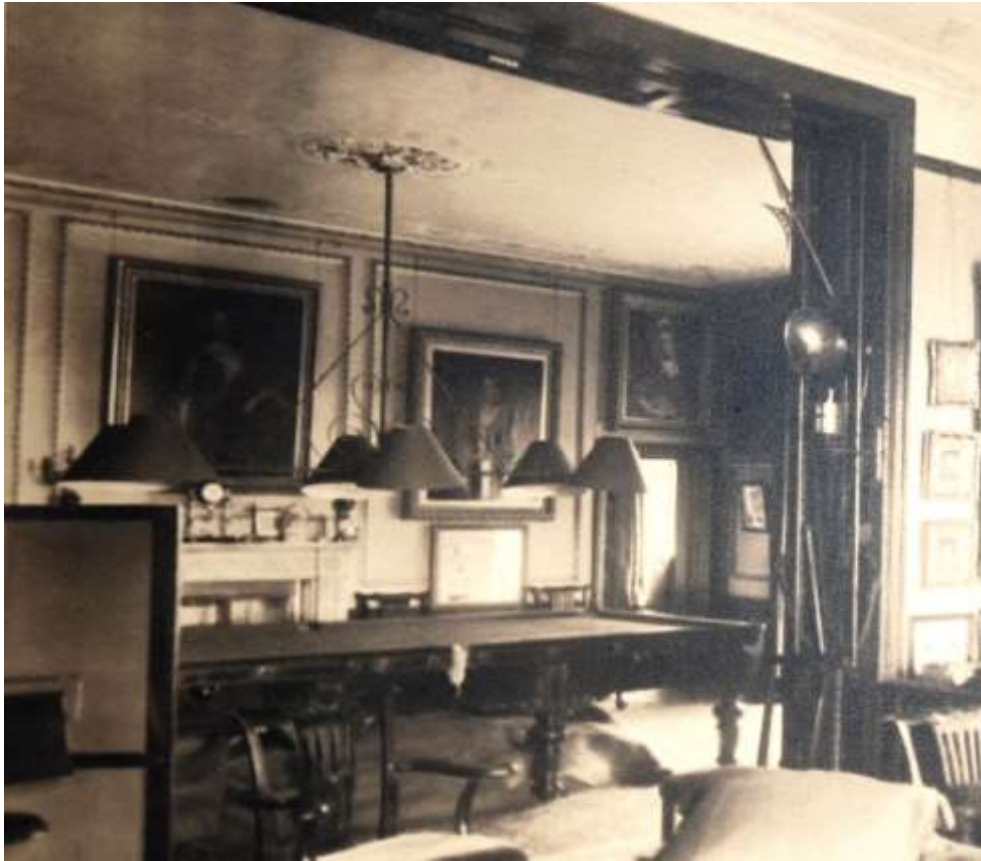
Fig. 181: c.1900 photograph of the billiard room, showing the fireplace.
