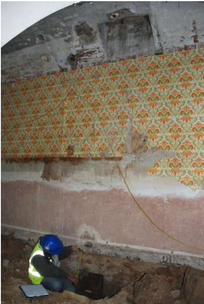
Fig. 106: Photograph of the shaft leading through to the pump room from the beer cellar. Just visible behind the scale is a bracket with two upstanding bolts, apparently identical to (but much more heavily corroded than) that recorded in the pump room (see fig. 111)
