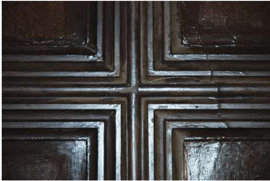
Fig. 123: Entrance Hall Ceiling.
