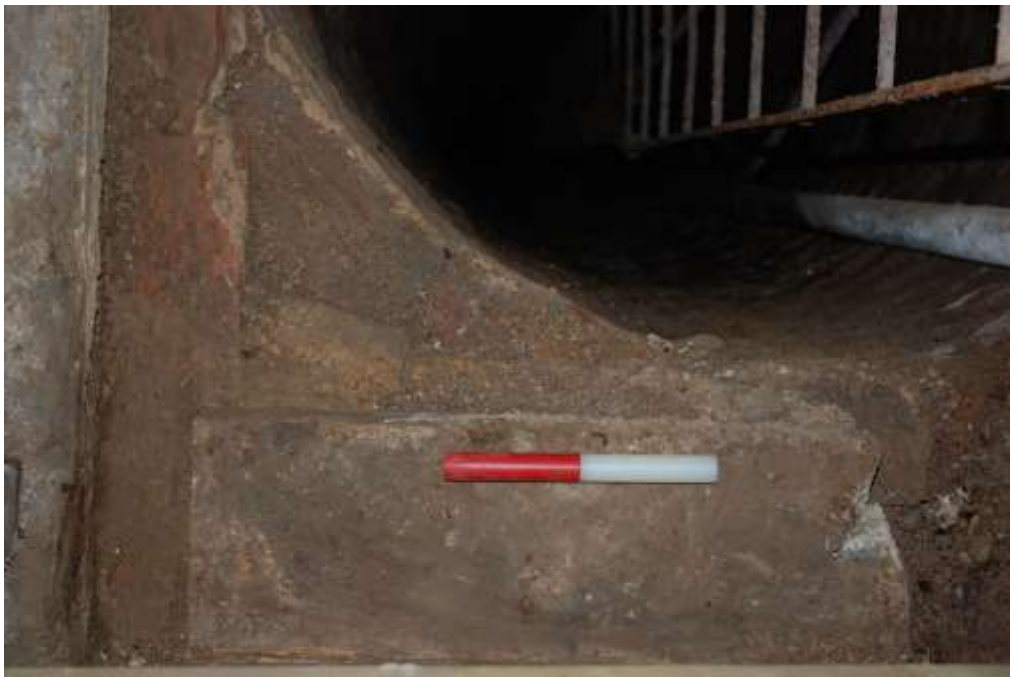
g raph of the north-east corner of the impression of the well-cover.
