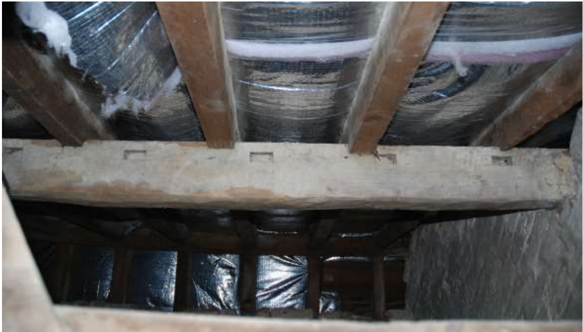
Fig. 69: Re-used timber above north-eastern part of room S13. The earlier mortices are visible.
