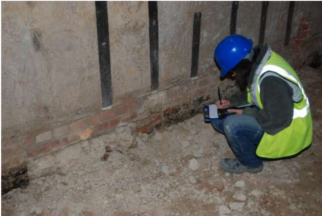
Fig. 90: Photograph of the blocked door on the western wall.
