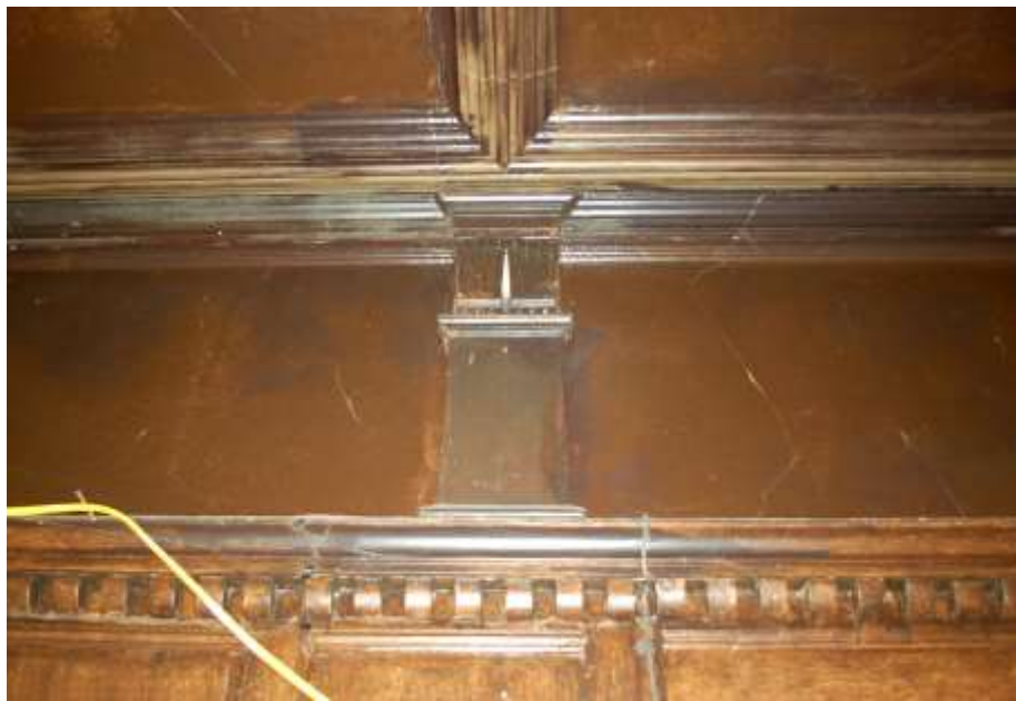
Fig. 301: Detailed photograph of the coving in the entrance hall, showing its re-painting (probably undertaken when Breakspears was used as a film-set).
