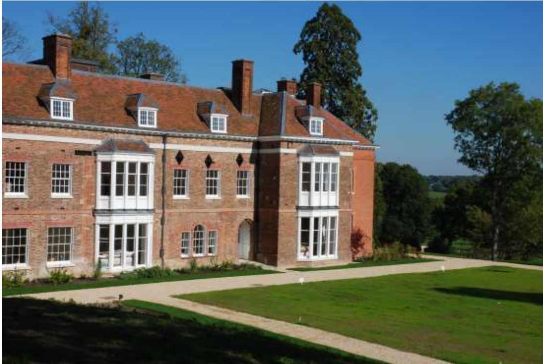
Fig. 30: Southern frontage. The brickwork of the 'earlier' house is visible in the central part of the photo (around the doorway and Venetian window), and that of the 'later' house in the western part (i.e. to the left of the closest bay-window).
