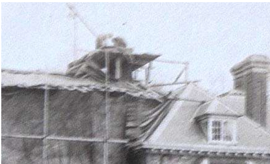
Fig. 256: 1925 photograph of the repair works, southern frontage, showing two men working on the chimney.
