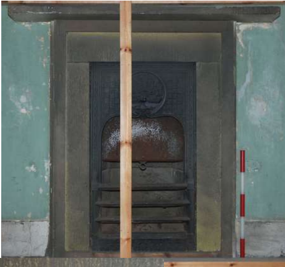
Fig. 76: Fireplace in room S10.
