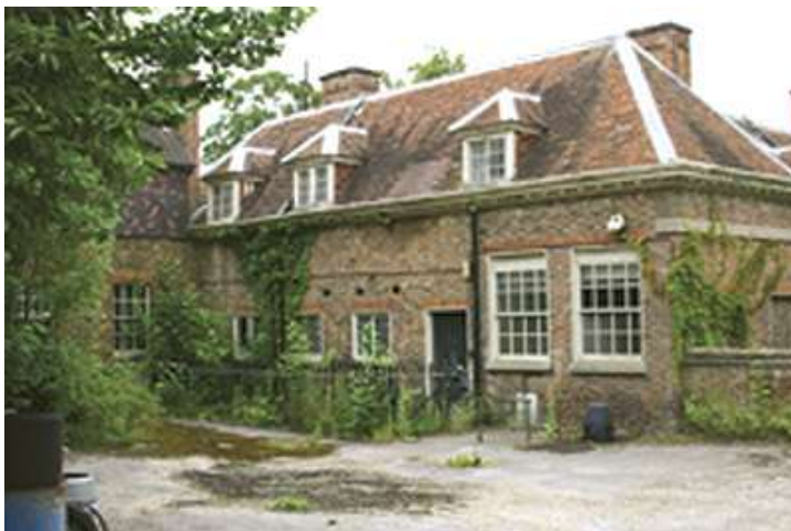
Fig. 152: Photograph of the water-tower prior to Clancy redevelopment works (provided by Clancy).
