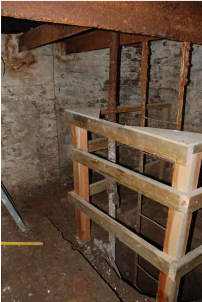
Fig. 112: Photograph of the pump room, with the well in the centre.
