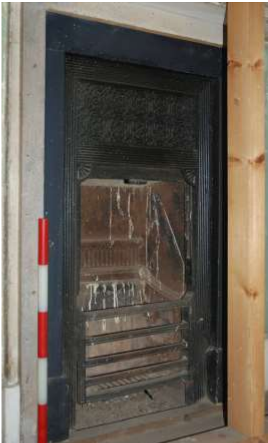
Fig. 132: Close-up of fireplace in room S9.
