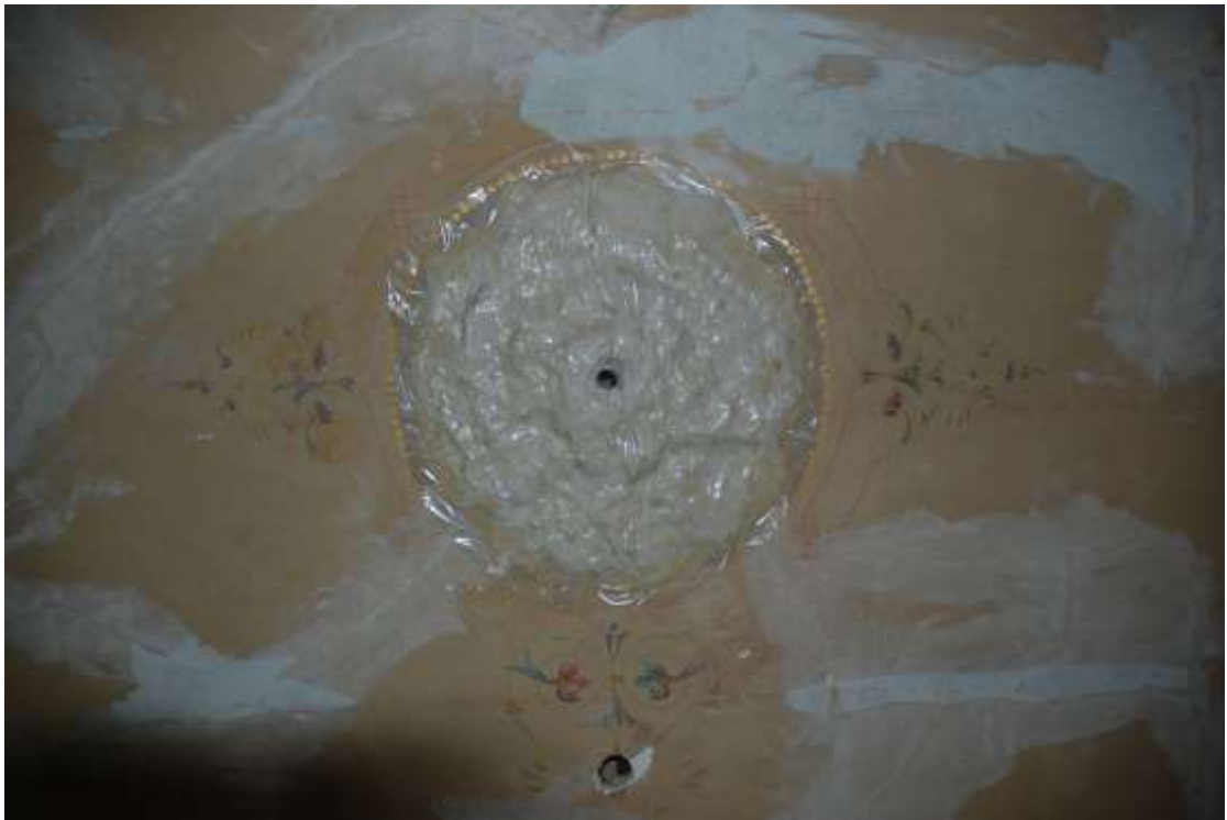
Fig. 191: Photograph of whole centre of the ceiling.
