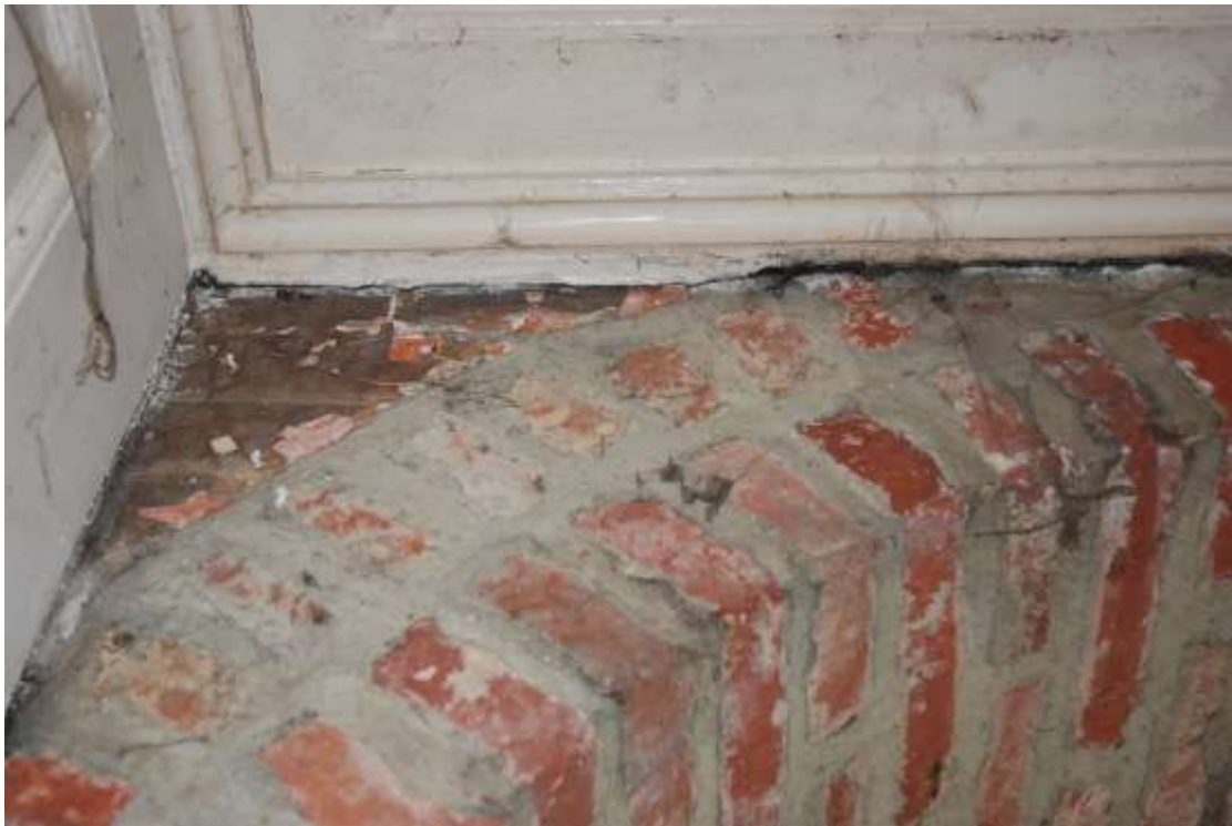
Fig. 146: Interior arch of the door, cutting through an earlier painted wall-face.
