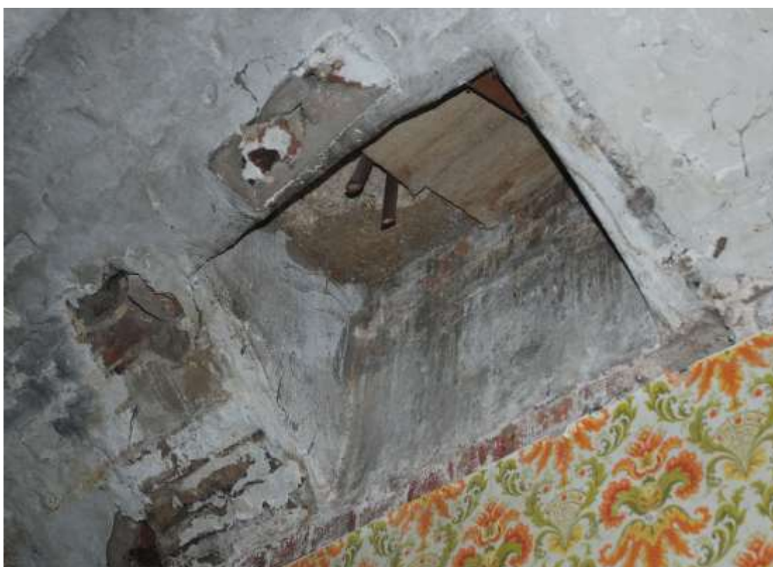
Fig. 105: Photograph of the (now-blocked) shaft in the ceiling of the beer cellar, through which the actuating rods would have run.
