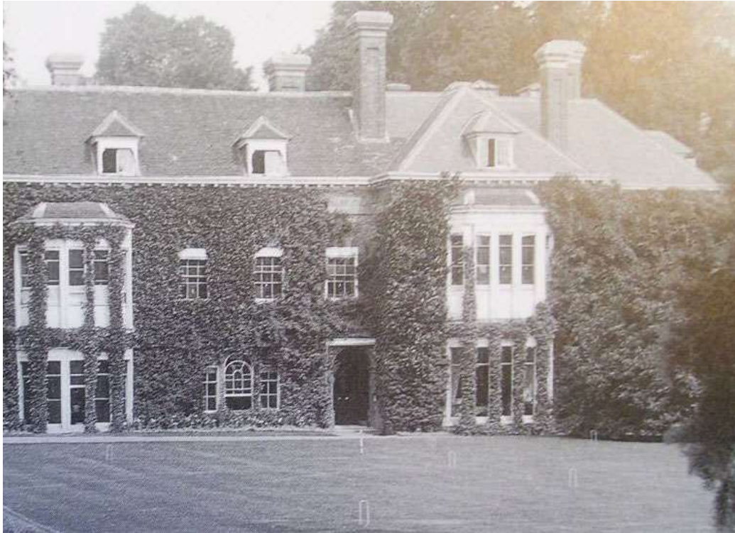
Fig. 166: Early 1900s photograph, clearly showing the new tiled roof over the eastern end of the house.
