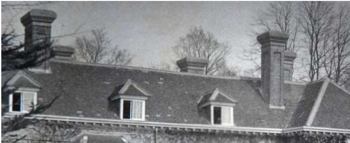
Fig. 257: 1890s photograph, depicting the ‘older’ type of chimney, with the capped tops.
