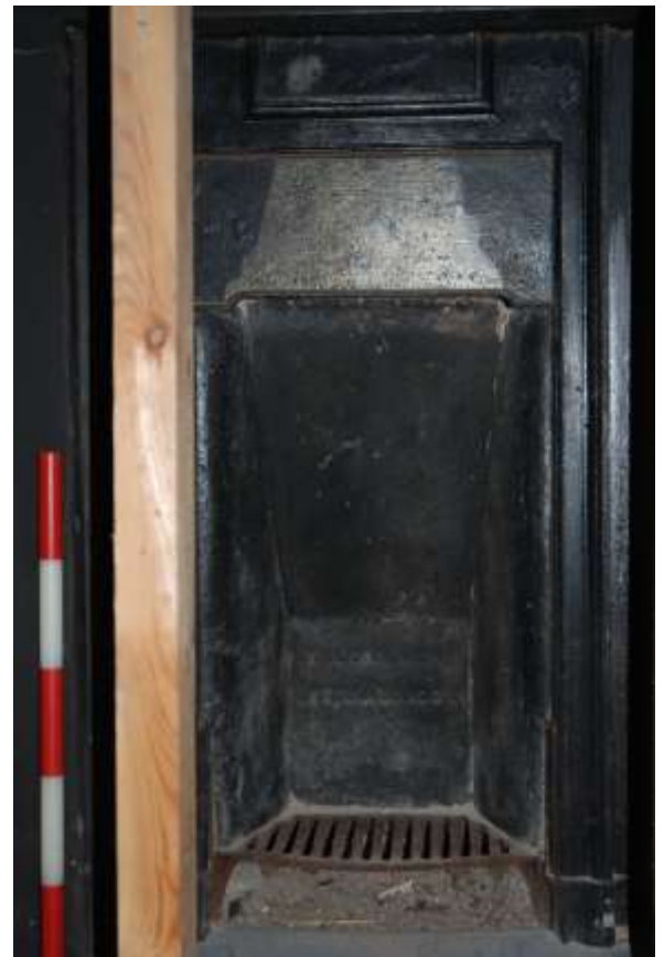
Fig. 215: Close-up of fireplace in the Blue Bedroom Dressing Room (F3).
