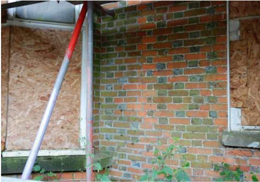
Fig. 144: Billiard room bay-window (background of shot), with earlier window half blocked by insertion of bay-window.
