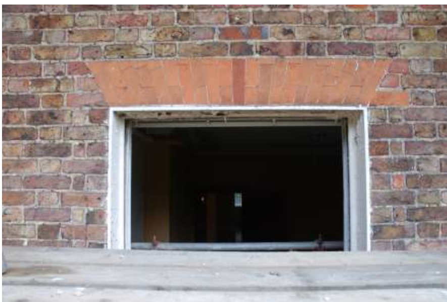
Fig. 34: Gauged brickwork above new windows.
