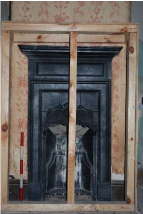
Fig. 222: Fireplace in room S1.
