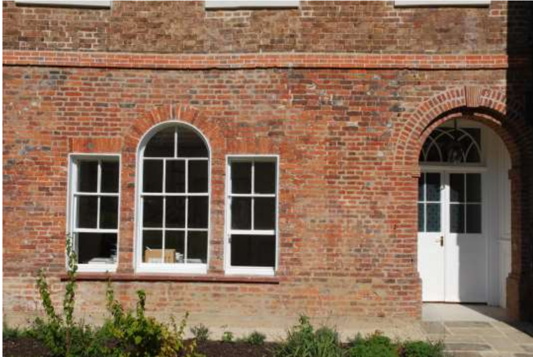
Fig. 255: Patching of the southern wall, around the Venetian window and door.
