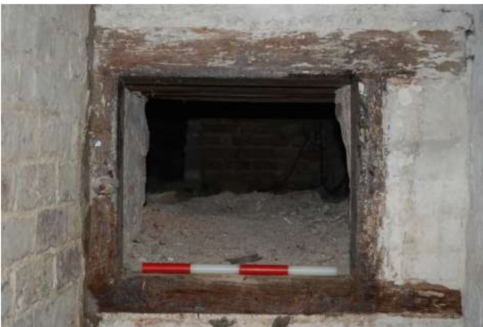
Fig. 174: Photograph of small timber-hatch in southwest corner of cellars.
