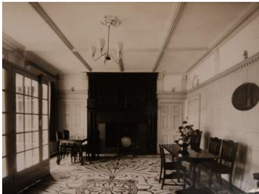
Fig. 283: 1960s photograph of the entrance hall, with the panelling having been painted over.
