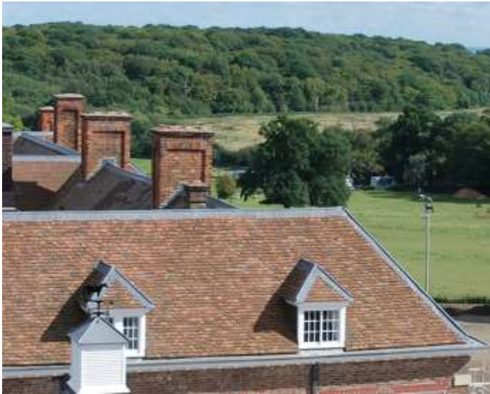
Fig. 248: Photograph of the small chimney (just in front of the larger one) which was attached to the later fireplaces in room F16 (and possibly F15).
