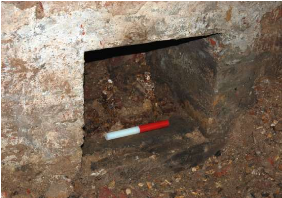
Fig. 106: Photograph of the shaft leading through to the pump room from the beer cellar. Just visible behind the scale is a bracket with two upstanding bolts, apparently identical to (but much more heavily corroded than) that recorded in the pump room (see fig. 111)
