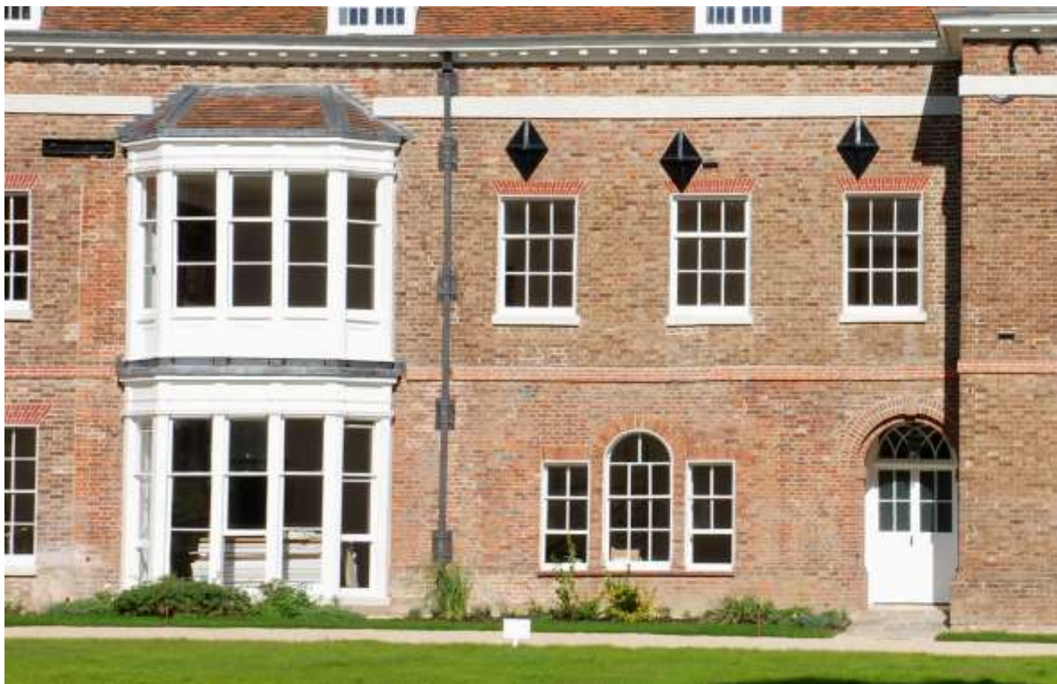
Fig. 254: Photograph of the four tie-rods (southern frontage).
