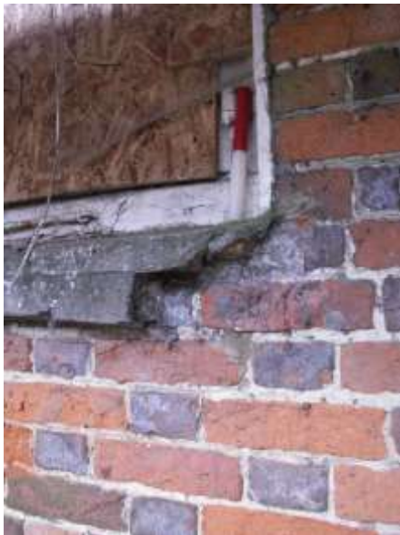
Fig. 33: New concrete window-sill.
