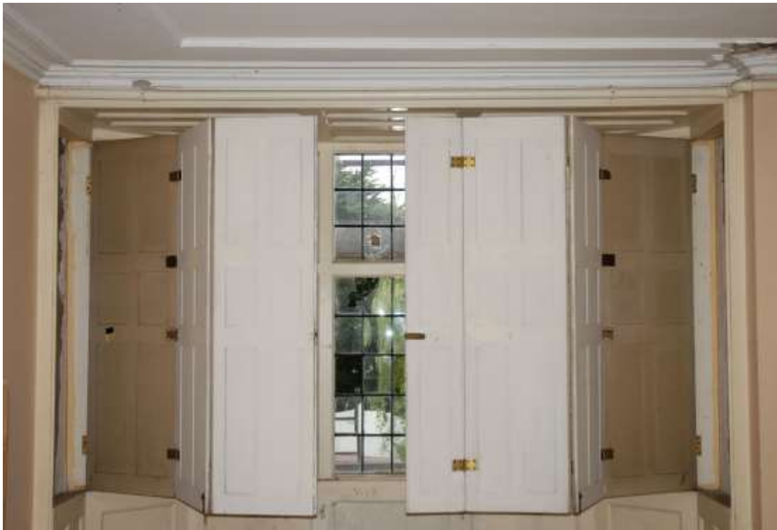
Fig. 41: Horizontal shutters in room F22.
