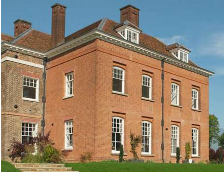
Fig. 169: Photograph of the eastern end of the house, showing the sash windows, decorative gauged brickwork above this, and new dormer windows.
