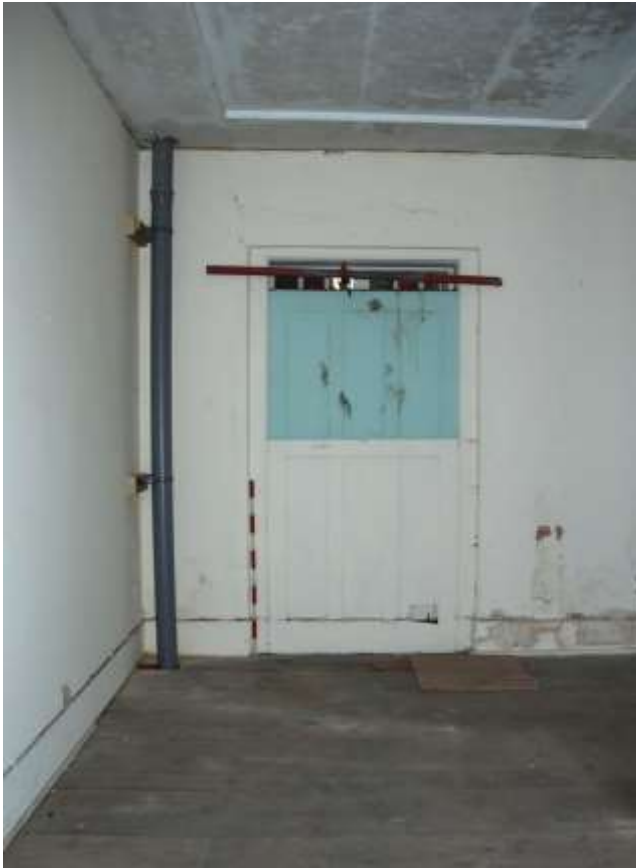
Fig. 40: Unusual window in room F18 with shutters which move up and down.
