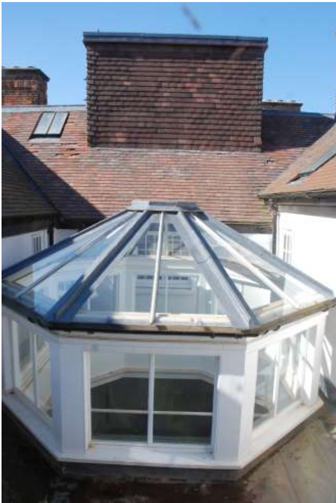
Fig. 50: Photograph of the lantern from the east.
