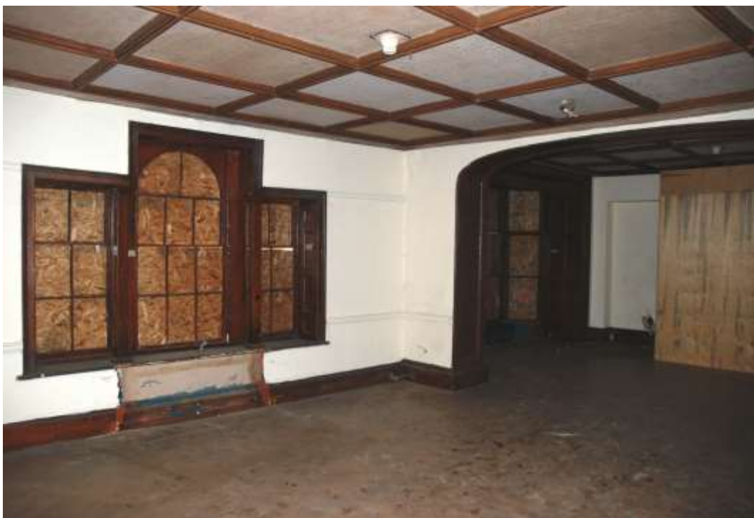
Fig. 299: Photograph of the library ceiling (film-set addition).
