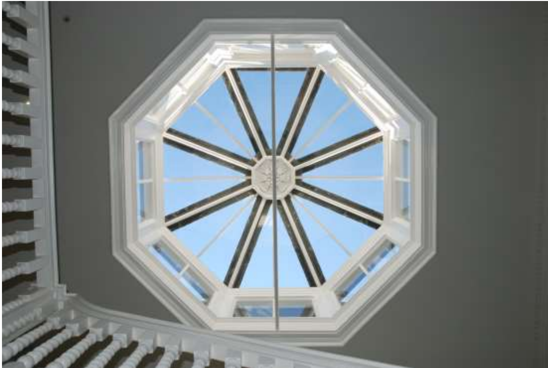
Fig. 49: Photograph of the lantern, looking directly up at it.
