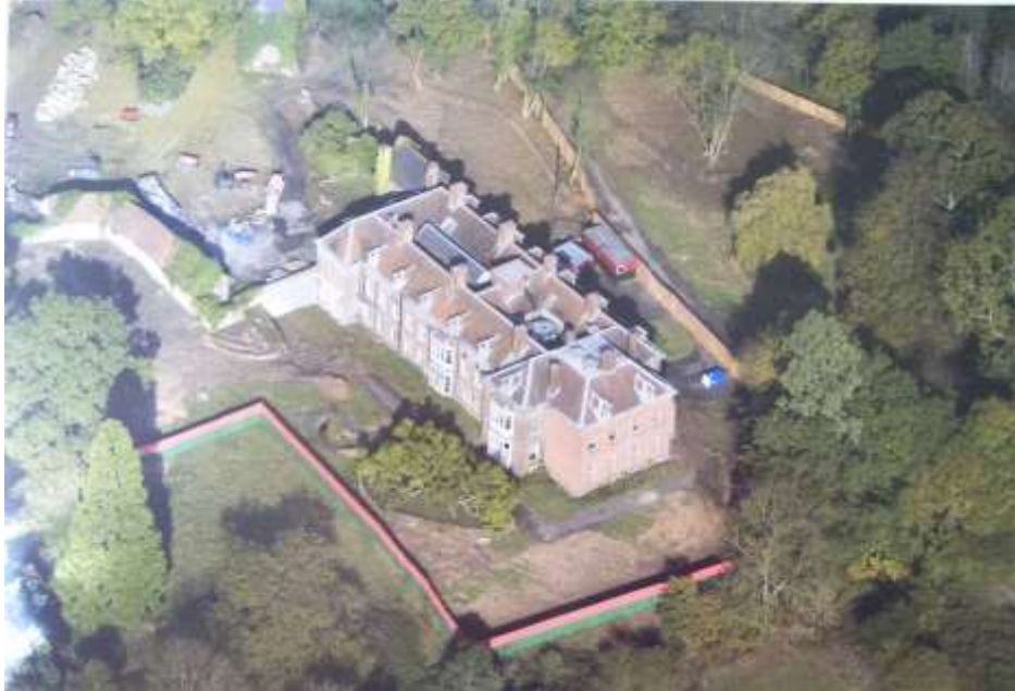
Fig. 45: Aerial photograph of Breakspears, looking north-west, immediately before building works. The nature of the roof can clearly be seen from this angle.
