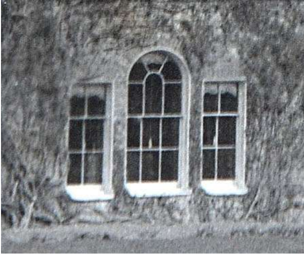
Fig. 260: c.1900 photograph of the Venetian window, showing its earlier splayed form.
