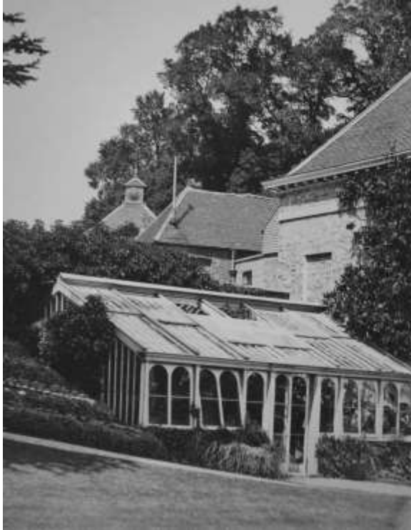
Fig. 153: c.1900 photograph, with tile-hung southern gable of the stores, and adjacent flat-roofed harness room, seen between the main house and stable roof.
