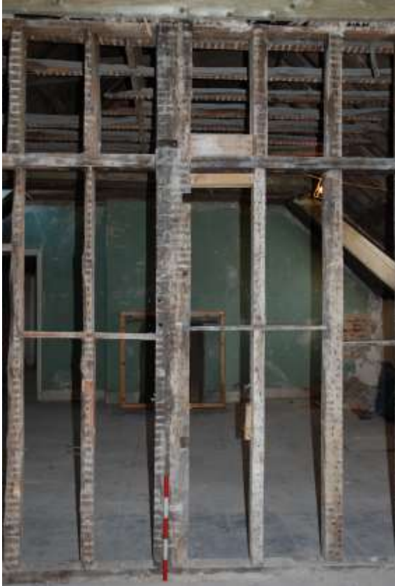
Fig. 70: Re-used timber above room S12. The earlier mortises are visible.
