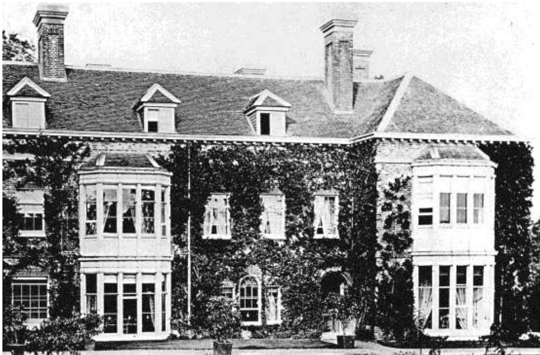
Fig. 38: 1860 photograph of the two bay-windows on the southern frontage.
