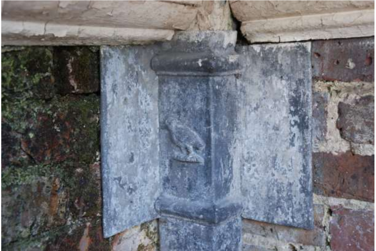
Fig. 61: The partridge emblem on the drain-pipe between rooms S3 and S6.
