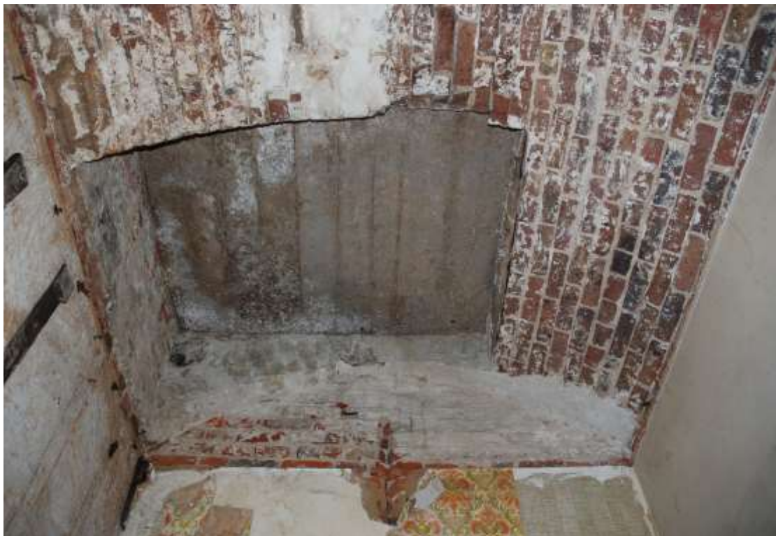
Fig. 89: Photograph of the access hatch (now blocked).
