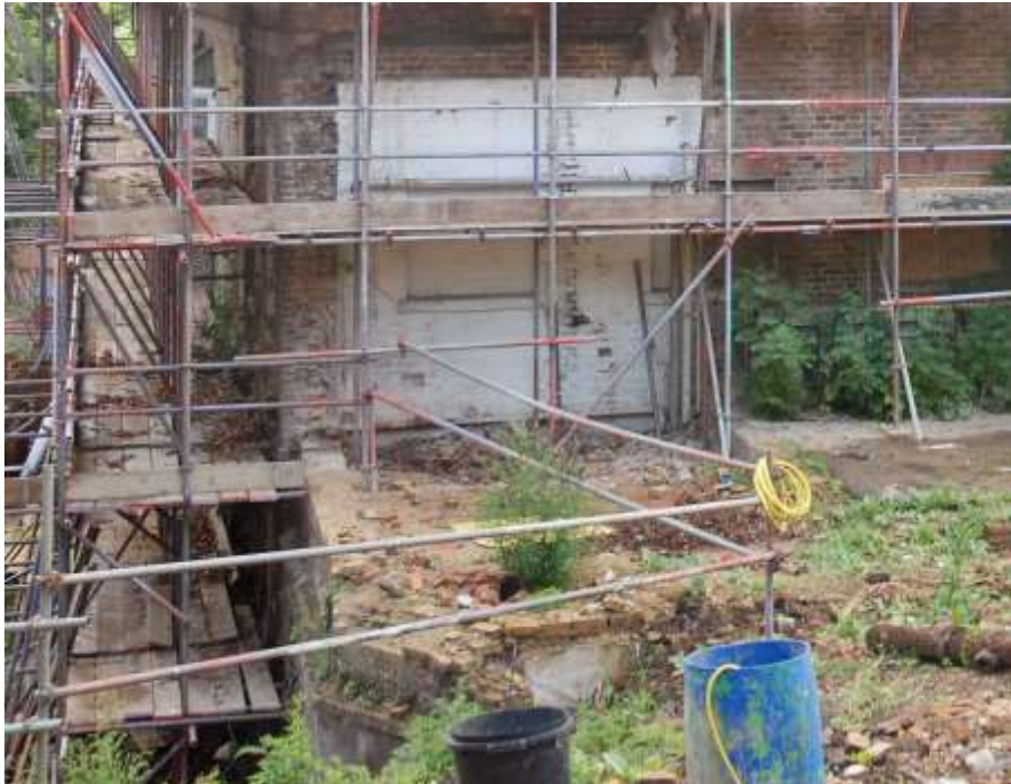
Fig. 149: Photograph of the two blocked-up windows in F18 – blocked up because of the construction of the western structure.
