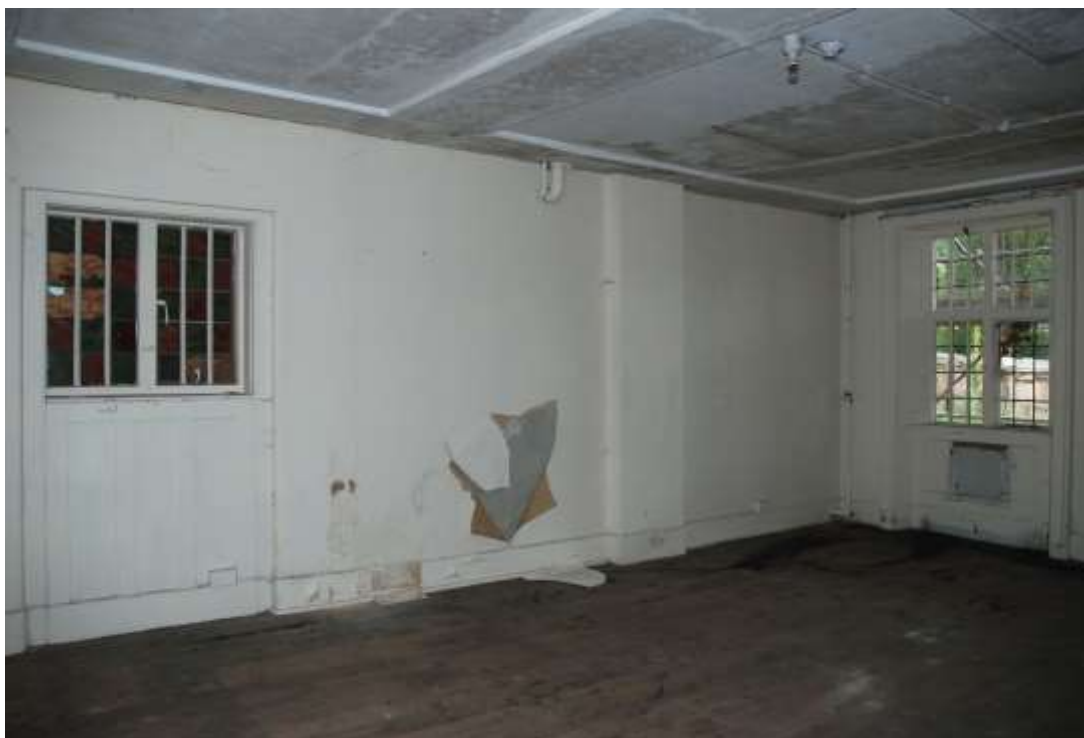
Fig. 53: Chimney-breast on the western wall of room F18.
