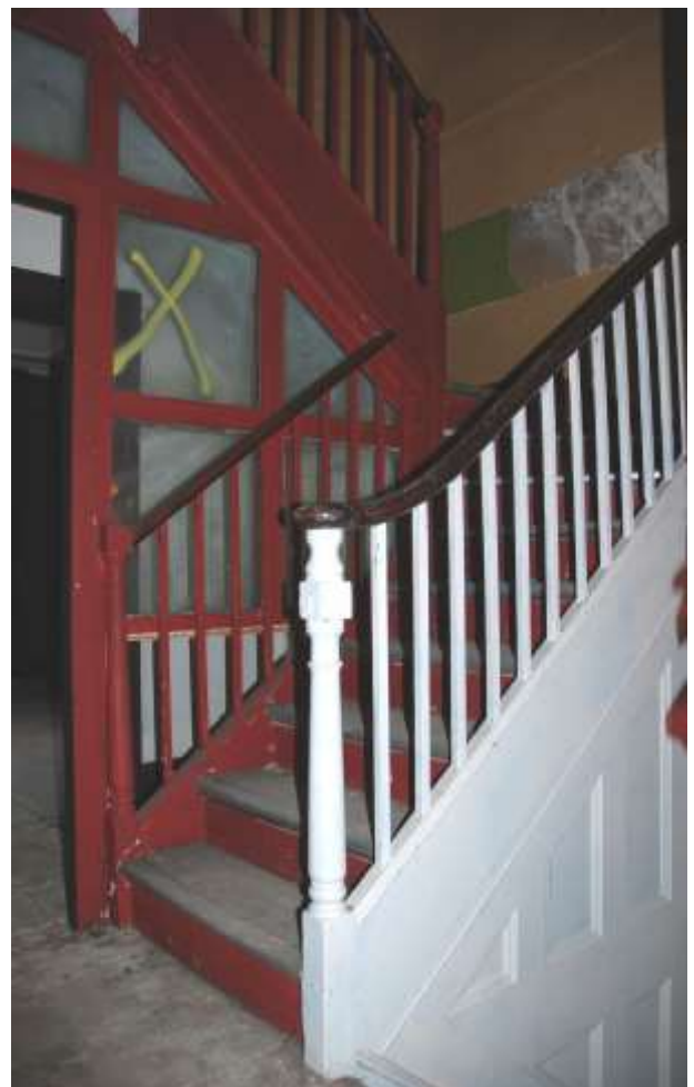
Fig. 66: The servants staircase, running from the first-floor up to the second-floor.
