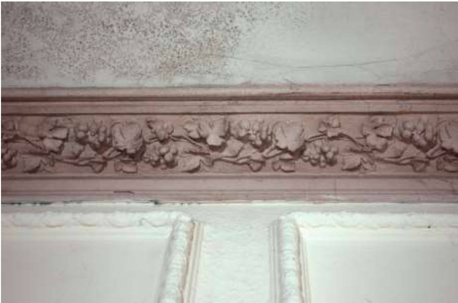
Fig. 207: Photograph of the cornice detail in the Billiard Room.
