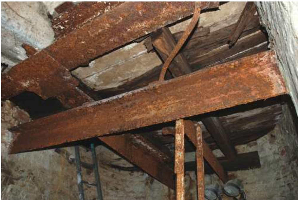
g raph showing the planking and roughly positioned supporting beams.
