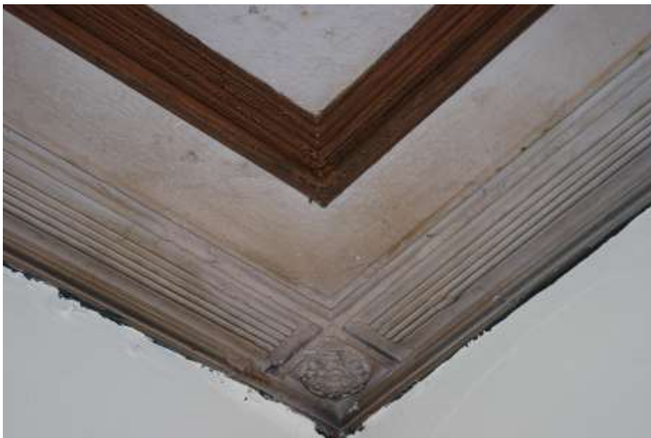
Fig. 126: Photograph of the library cornice.
