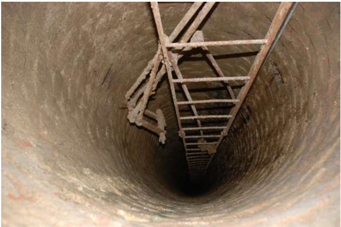
Fig. 114: Photograph looking directly down the well. The axle-type arrangement attached to the actuating rods and now at the lowest level (to the left of the ladder) was probably originally fixed at the top of the well.
