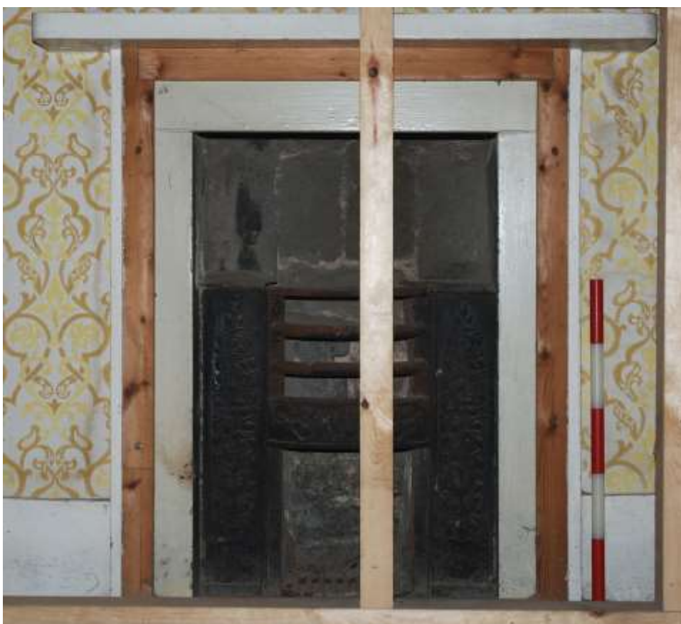
Fig. 81: Fireplace in room S16.
