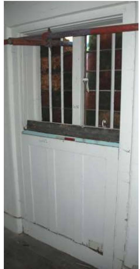
Fig. 40: Unusual window in room F18 with shutters which move up and down.
