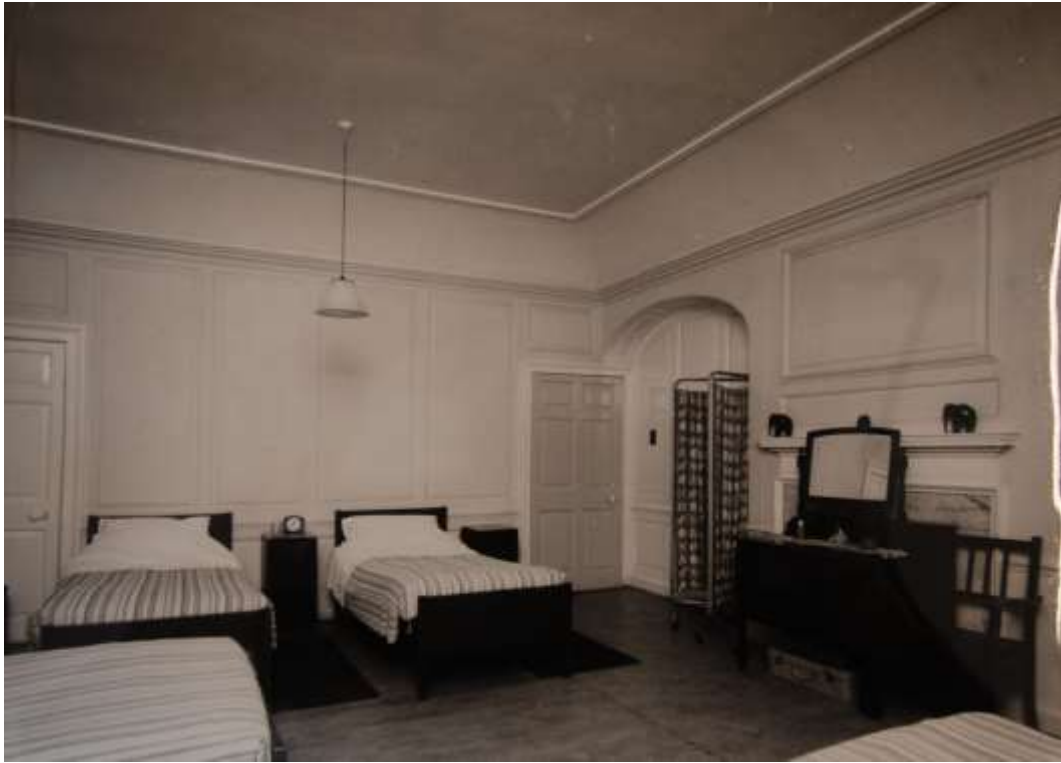
Fig. 266: 1968 photograph of one of the dormitories (room F6) when it was in use as a care home.
