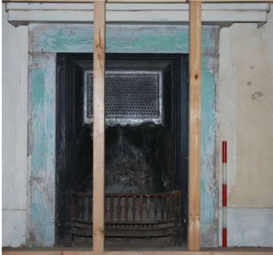
Fig. 80: Fireplace in room S15.
