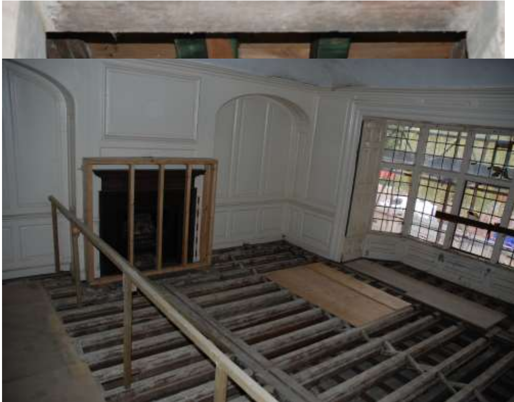
Fig. 230: Photograph of the joists in room F6.
