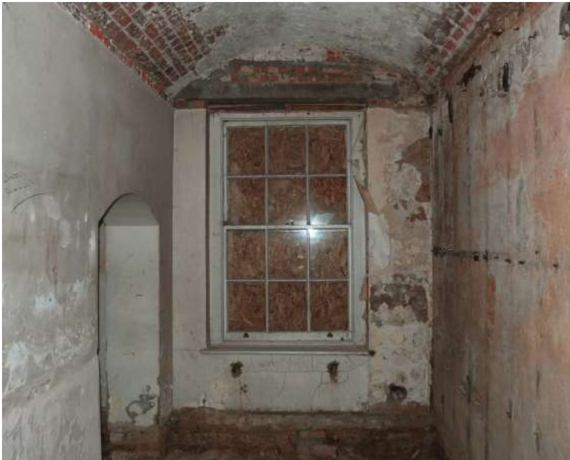
Fig. 281: Photograph of one of the windows in the southern wall of the Beer Cellar, inserted when Breakspears was converted into a care home. The concrete lintel and modern brickwork above this can clearly be seen.
