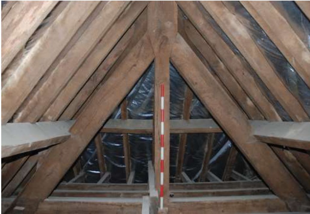
Fig. 99: Photograph of one of the king posts (behind the scale), with the blades and common rafters clearly visible. Looking south.
