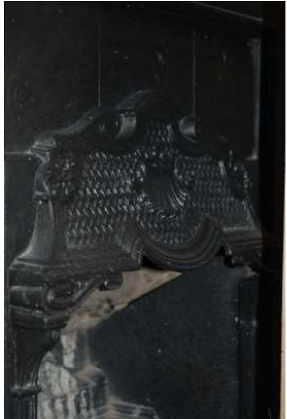
Fig. 223: Close-up of fireplace in room S1.
