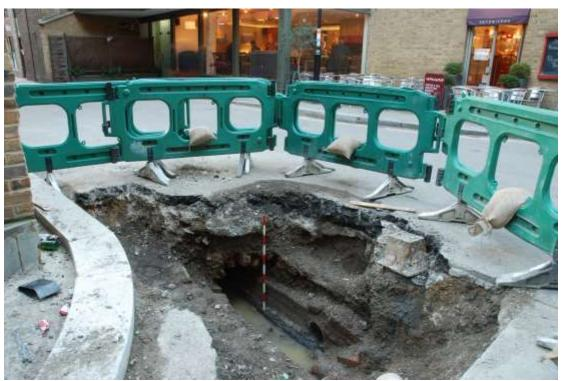
Fig.23: Victorian Sewer exposed in trenching on 6<sup>th</sup> December 2012. Facing SE
