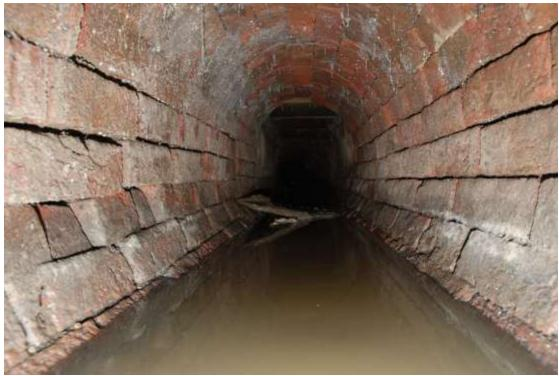
Fig.25: Interior of sewer, facing S. (9<sup>th</sup> January 2012). The roof of the sewer is cut by a later inspection chamber some 2.5m to the south, but the structure continues beyond this point for an unknown distance.
