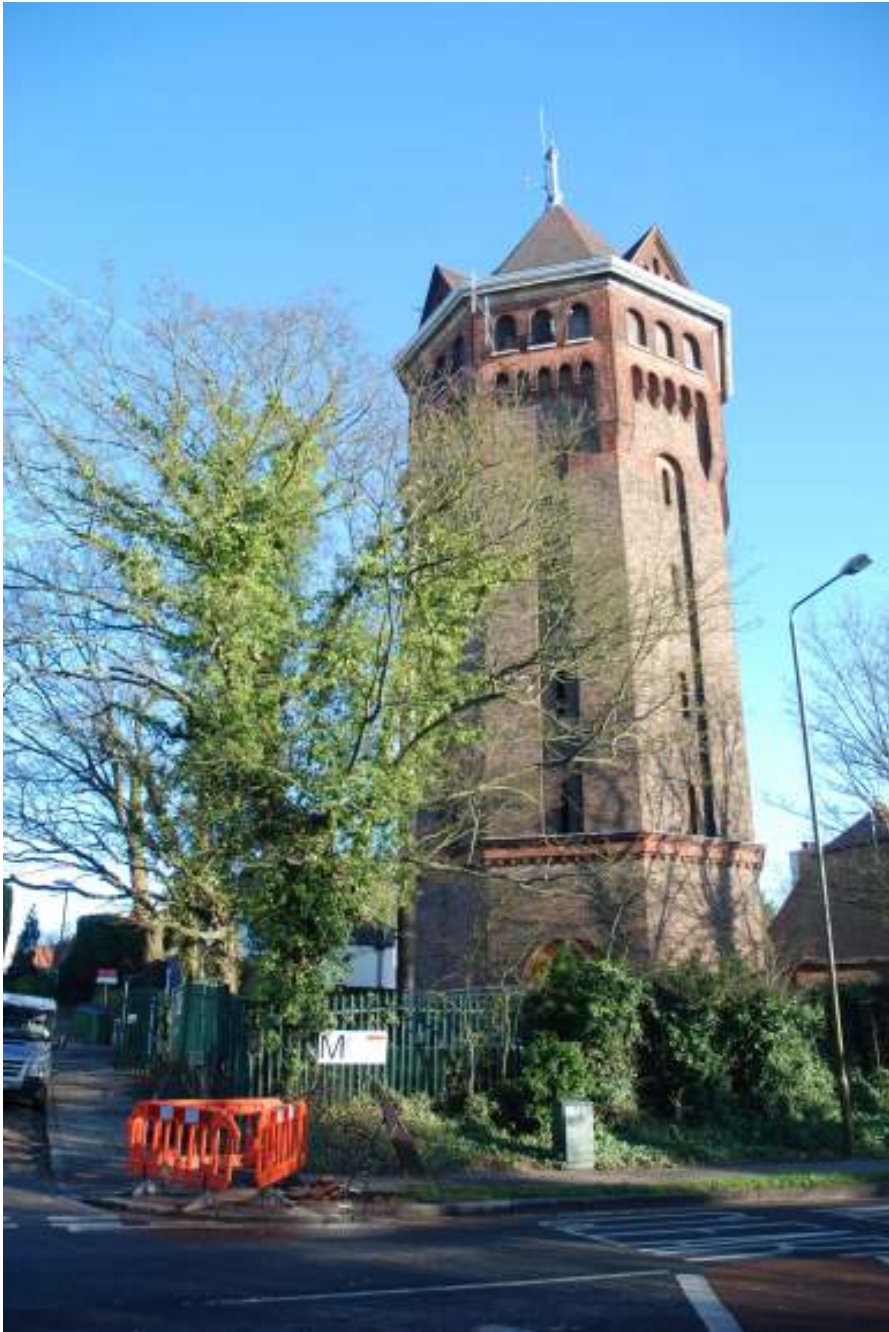
Fig.1: General location shot of chamber excavated on corner of Cleanthus Road, (left of frame), and Dover road, (foreground). Facing N
