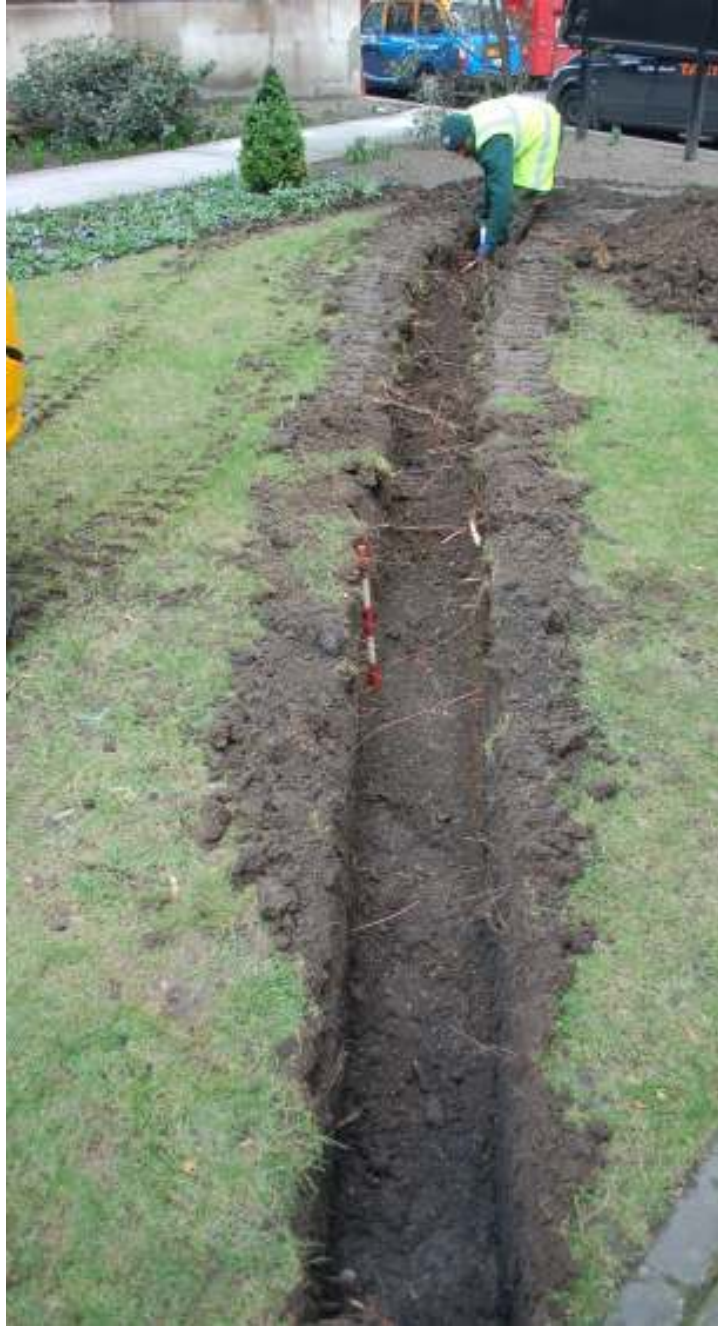
Fig.18: Clearing loose from the base of Trench 10 post machine dig, facing N, (0.5m scale)
