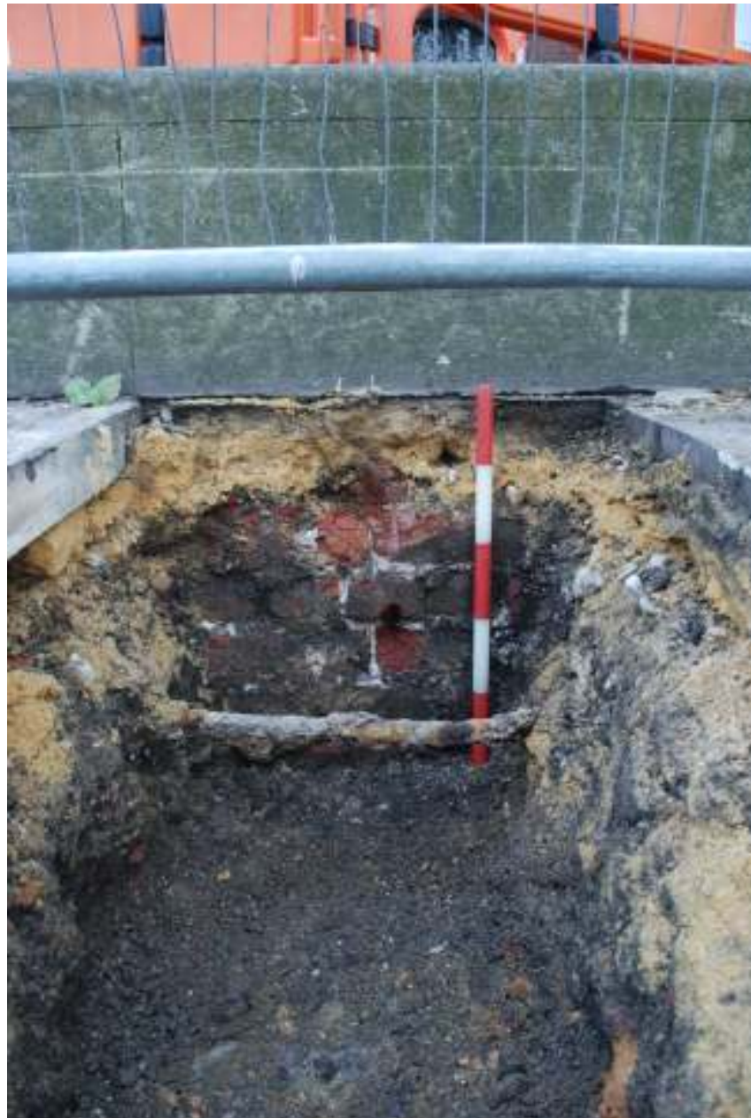
Fig.24: Wall footings exposed at NW end of trench 13, facing NW. (0.5m scale)
