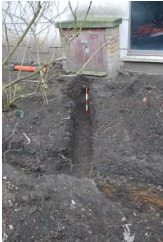
Fig.30: Trench from electricity box to trench 4. (0.5m scale)
