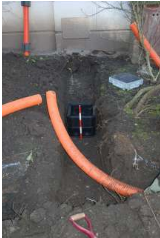
Fig.31: Trenching by electricity box on 12 th March 2012, facing SE
