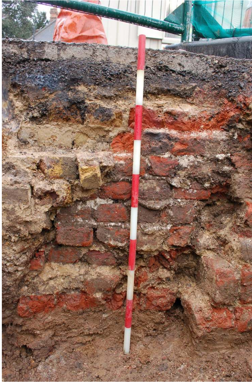
Fig.13: Red brick wall built on natural clay geology, later yellow brick wall built on southern end. Facing SW, (1m scale)
