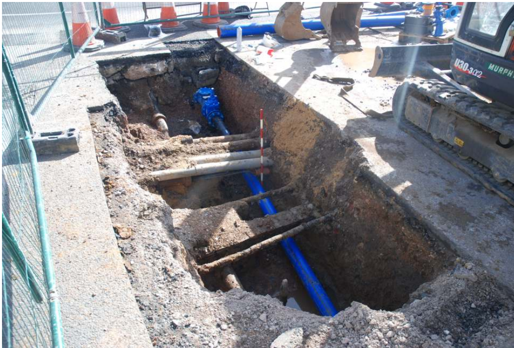
Fig.17: Pit dug on corner of Strafford Road and Richmond Road, facing S, (1m scale) Note the densely packed services and disturbed ground / backfill within the pit.
