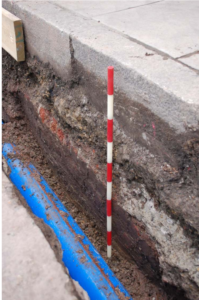
Fig.18: Curved back wall of coal cellar present beneath western kerbing of Farringdon Road, facing SSW 15 th February 2012, (1m scale)
