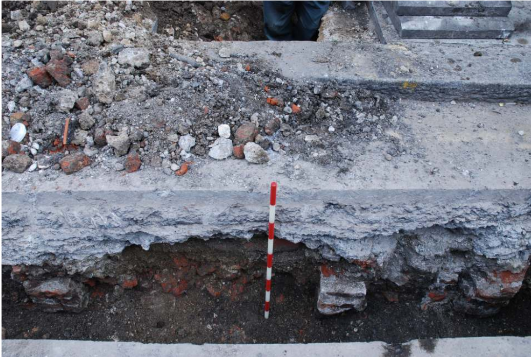
Fig.21: Stub walls within trench outside No.136 Grays Inn Road, facing E, 14 th July 2011. (1m scale)
