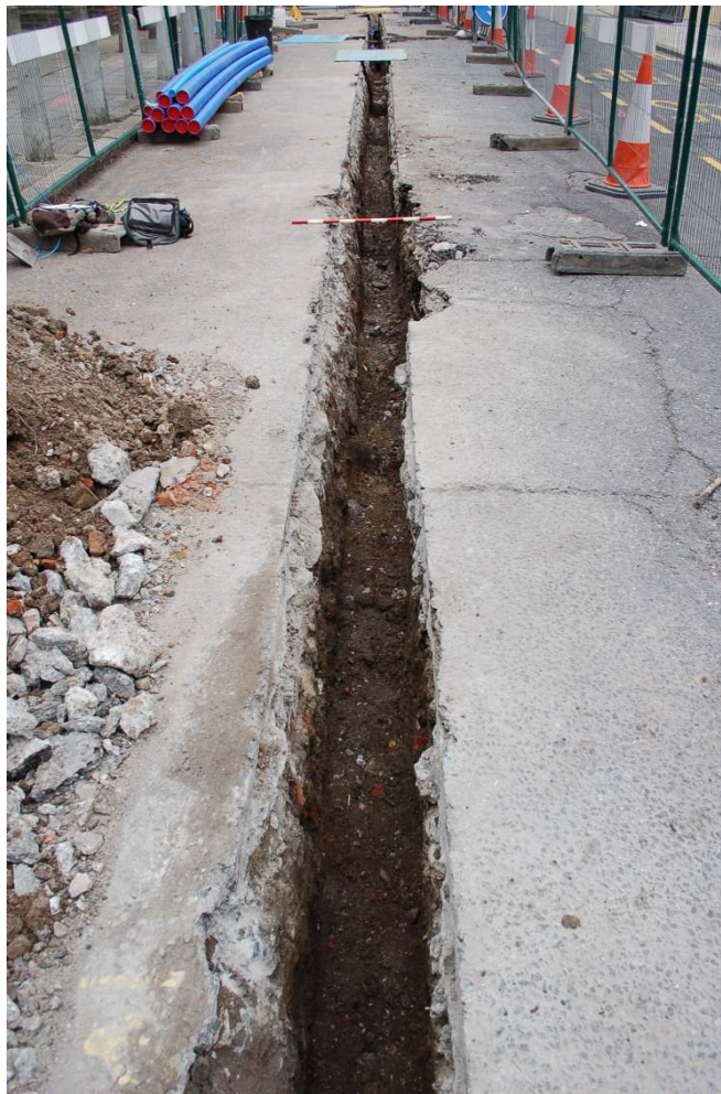
Fig.20: Trenching along Grays Inn Road, 6 th July 2011, facing S. (1m scale)
