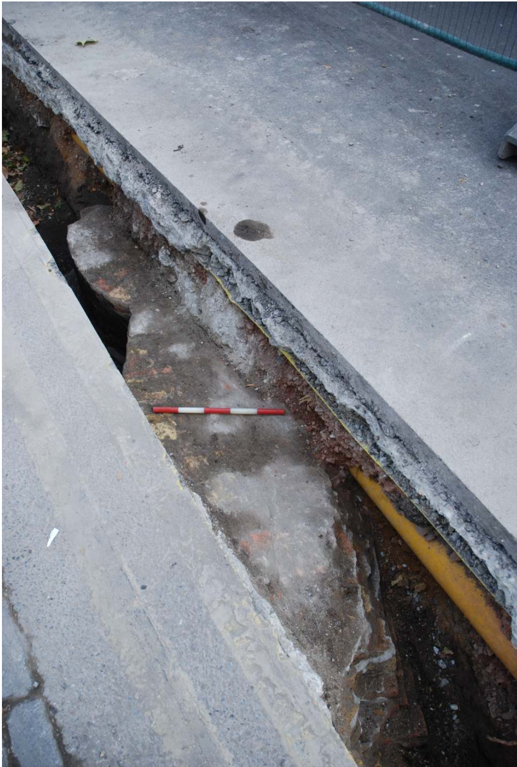
Fig.26: Wall found in trenching on Roseberry Avenue, 6 th December 2011. Facing NE (0.5m scale)
