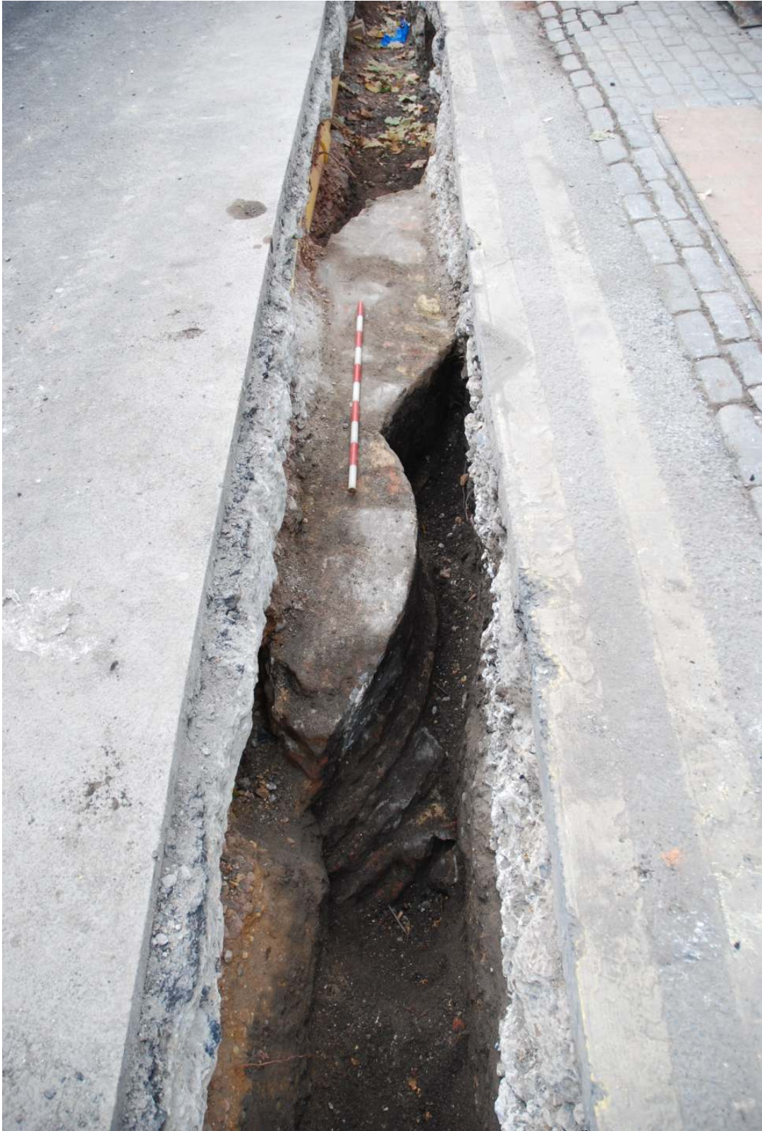
Fig.27: Corner buttress in brickwork of prison wall. Facing SSW, 6 th December 2011
