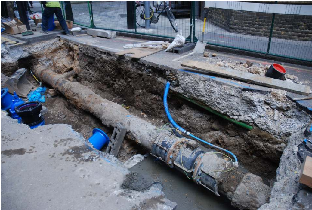
Fig.22: Pit opened on Leather Lane, 11 th September 2011, facing NW
