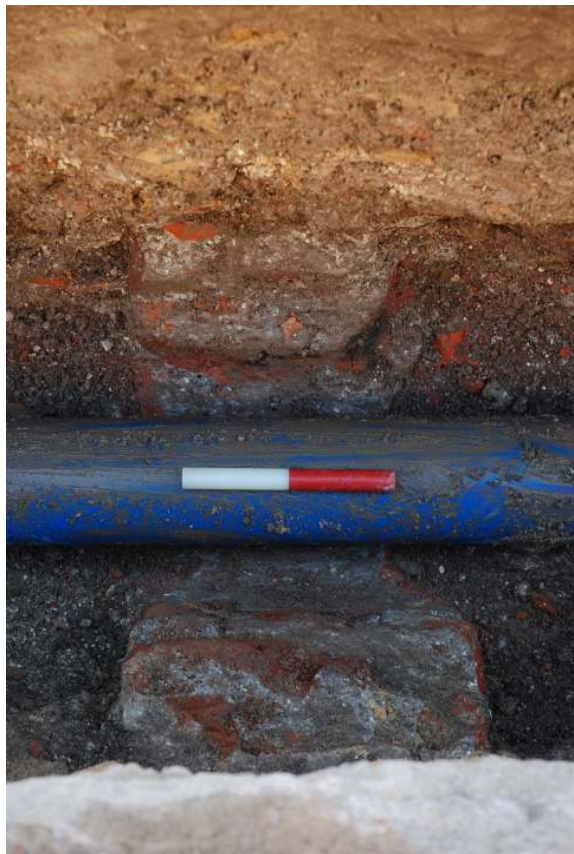
Fig.14: Brick wall in base of trenching 28 th October 2011, facing S. (20cm scale)
