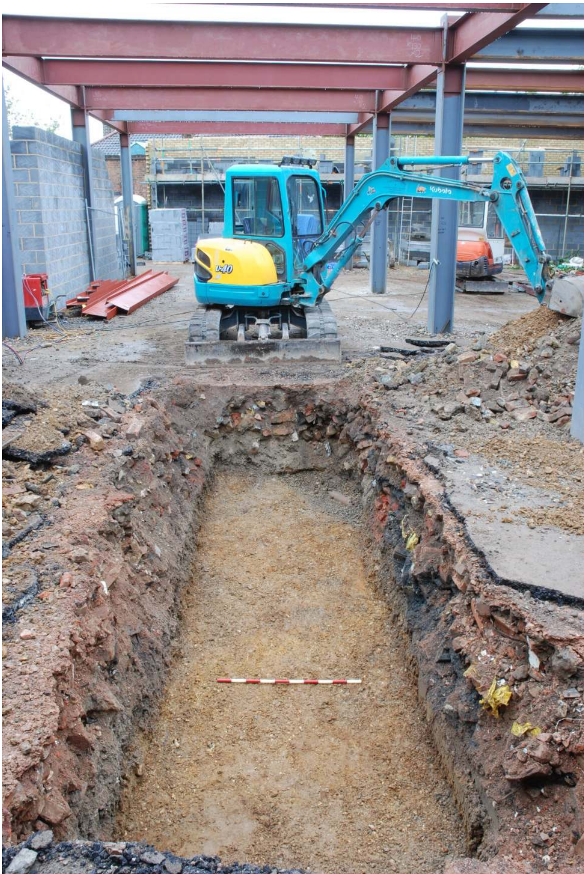
Fig. 13: Photograph of trench 1, looking west. The modern drain, cutting into the natural deposits, is visible in the top right of frame.
