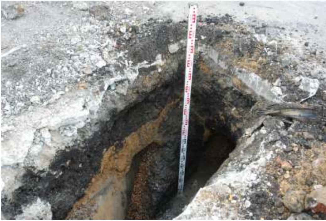
Fig. 15: Photograph of pit 2, looking south-west. The large pipe in the south-eastern corner of the pit is visible, alongside the dark grey-brown silty-gravel deposit (behind the scale)
