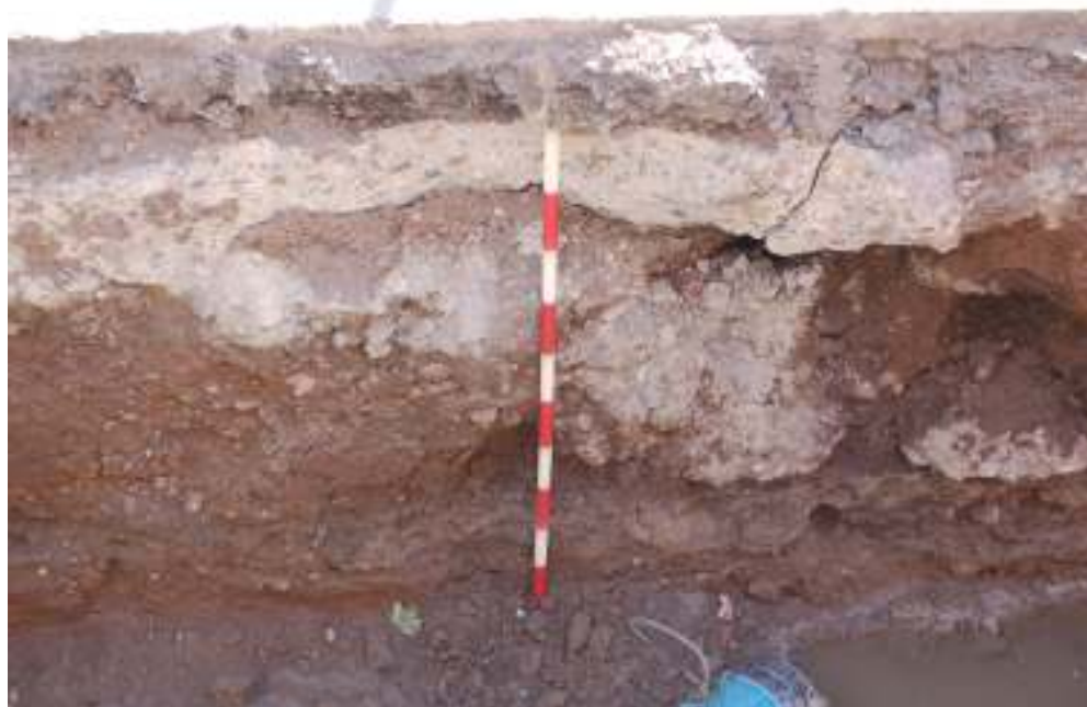
Fig. 33: Photograph of a section in one of the pits on East Road, showing the modern road-surface over the mid grey-brown clay made-ground deposit.
