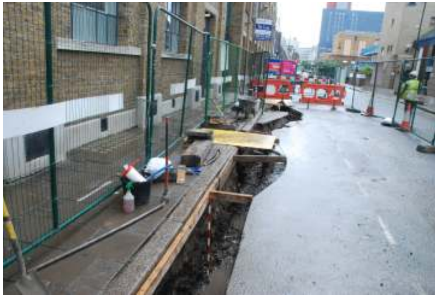
Fig. 98: General photograph of trenching on Wharf Road, looking south.
