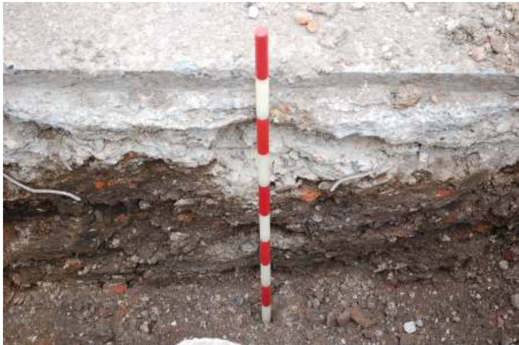
Fig. 90: Photograph of a section in the trenching on Wenlock Street, showing the modern road-surface overlying made-ground deposits.
