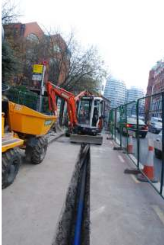
Fig. 19: Photograph of the trenching along City Road, looking east.
