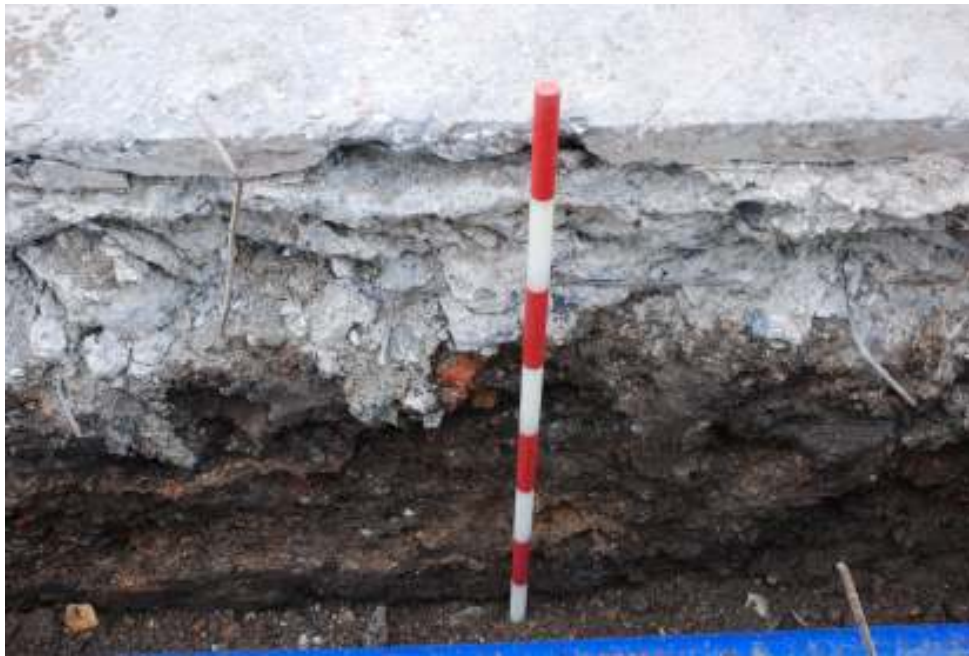
Fig. 25: Photograph of a section in the trenching on Cropley Street, showing the modern road-surface overlying made-ground deposits.
