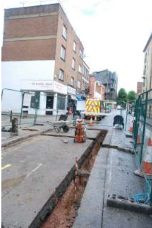
Fig. 59: Photograph of trenching on Nile Street, looking east.
