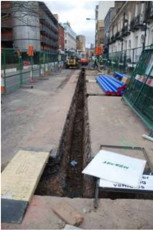
Fig. 77: Photograph of trenching on Shepherdess Walk, looking south.
