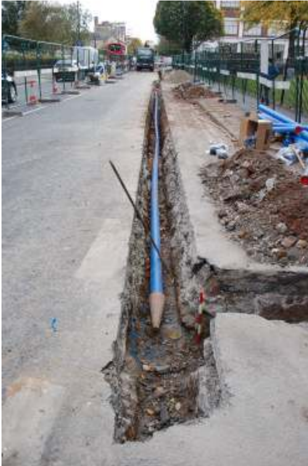
Fig. 55: General photograph of the trenching on New North Road, looking south.
