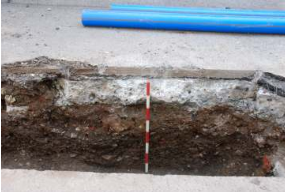
Fig. 92: Photograph of a section in the trenching on Wenlock Street, showing the modern road-surface overlying silty-sand made-ground deposits over more compact clayey deposits.
