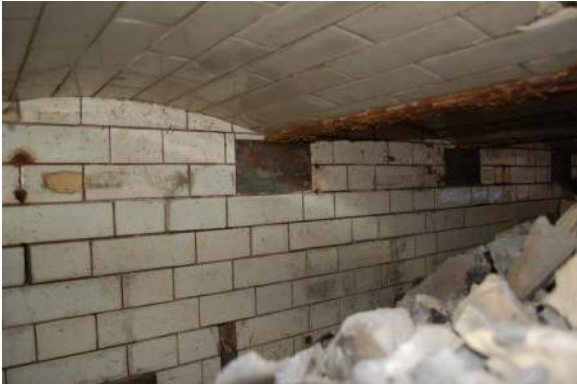
Fig. 50: Photograph of the underground toilet observed on New North Road. The vaulted ceiling, plus white-glazed bricks, are clearly visible.
