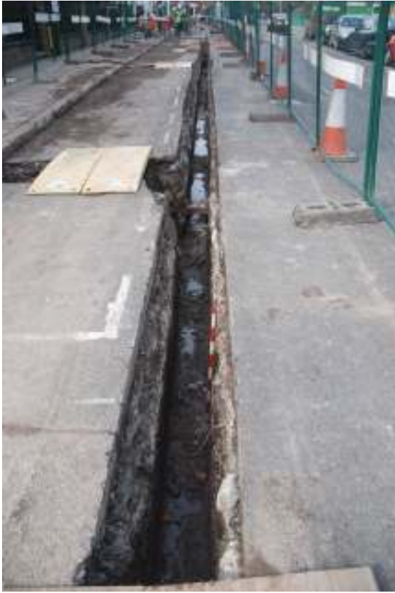
Fig. 49: Photograph of the trenching on New North Road.
