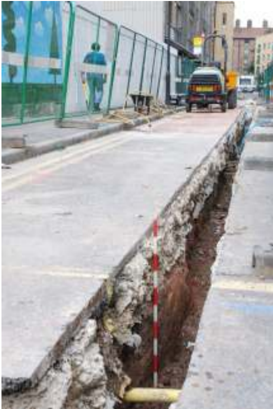
Fig. 63: Photograph of the brick wall base observed towards the southern end of Provost Street.
