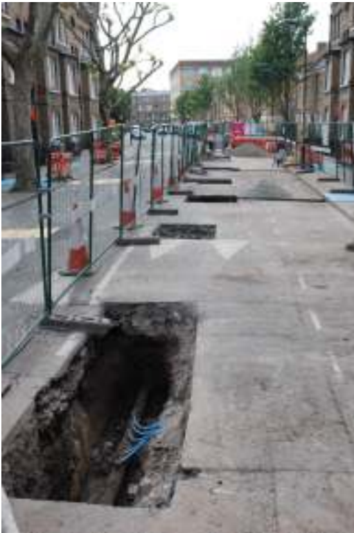
Fig. 40: Photograph of some of the pits on Haberdasher Street, looking west.
