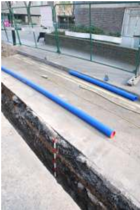
Fig. 44: Photograph of trenching along Murray Grove, looking south-east.
