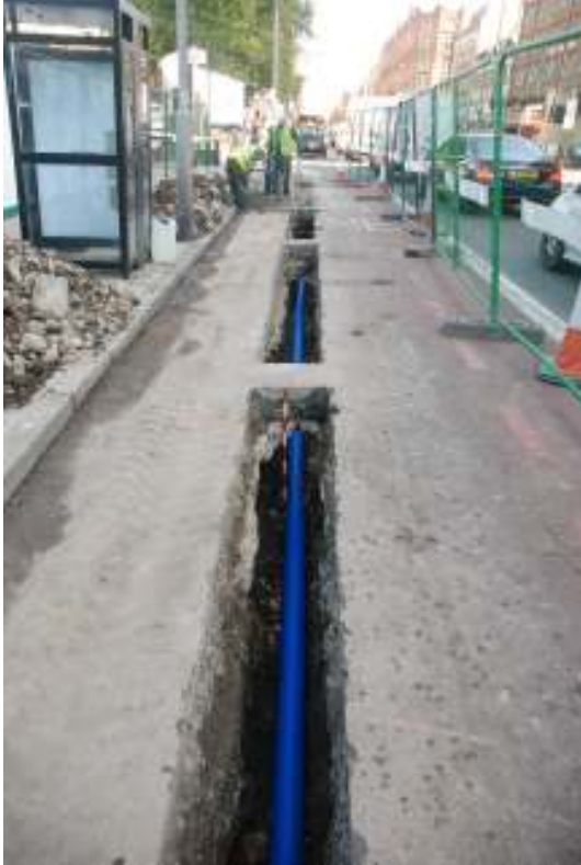
Fig. 18: Photograph of the trenching along City Road, looking east.
