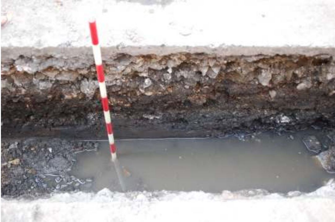
Fig. 87: Photograph of section in trenching along Wenlock Road, northern end.
