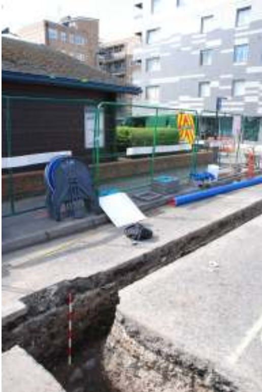
Fig. 45: Photograph of trenching along Murray Grove, looking south-west.
