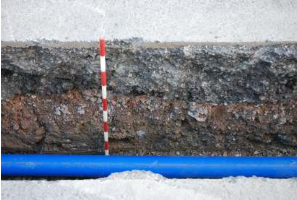
Fig. 52: Photograph of a section in the trenching along New North Road, showing the modern road-surface overlying the made-ground deposit.
