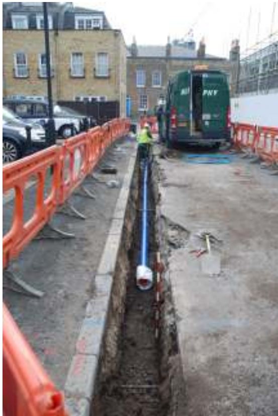
Fig. 81: General photograph of the trenching along Taplow Street.
