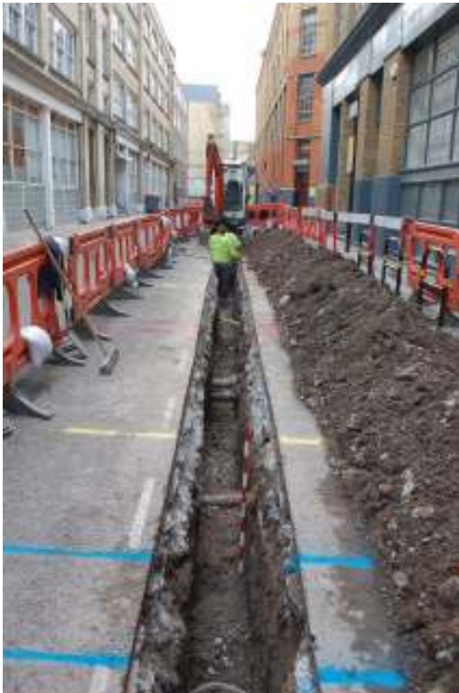
Fig. 85: Photograph of trenching on Underwood Street, looking south.
