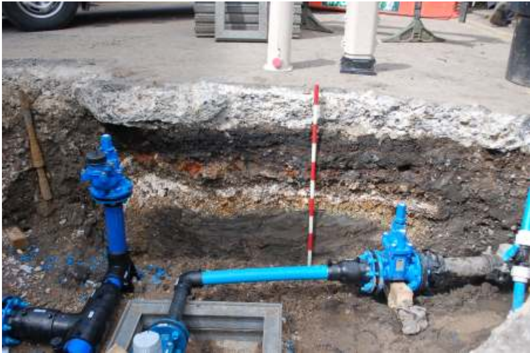
Fig. 88: Photograph of pit at far northern end of Wenlock Road, showing various made-ground layers over blue / black alluvium.
