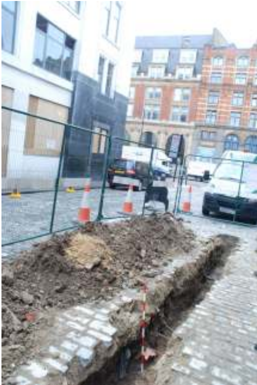
Fig. 94: Photograph of trenching on Westland Place, looking south.
