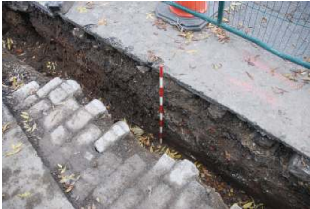
Fig. 23: Photograph of the trenching on Cropley Street, showing the modern road-surface overlying made-ground deposits.
