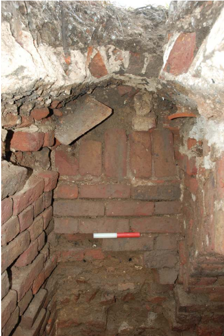
Fig.30: Remains of the transverse arch, which once covered the NE end of the structure. The main arched ceiling of the chamber is visible in the bottom right of the frame. Facing SE, (20cm scale. Note the shovel blade protruding from the section. Obviously the result of some previous episode of disturbance!)
