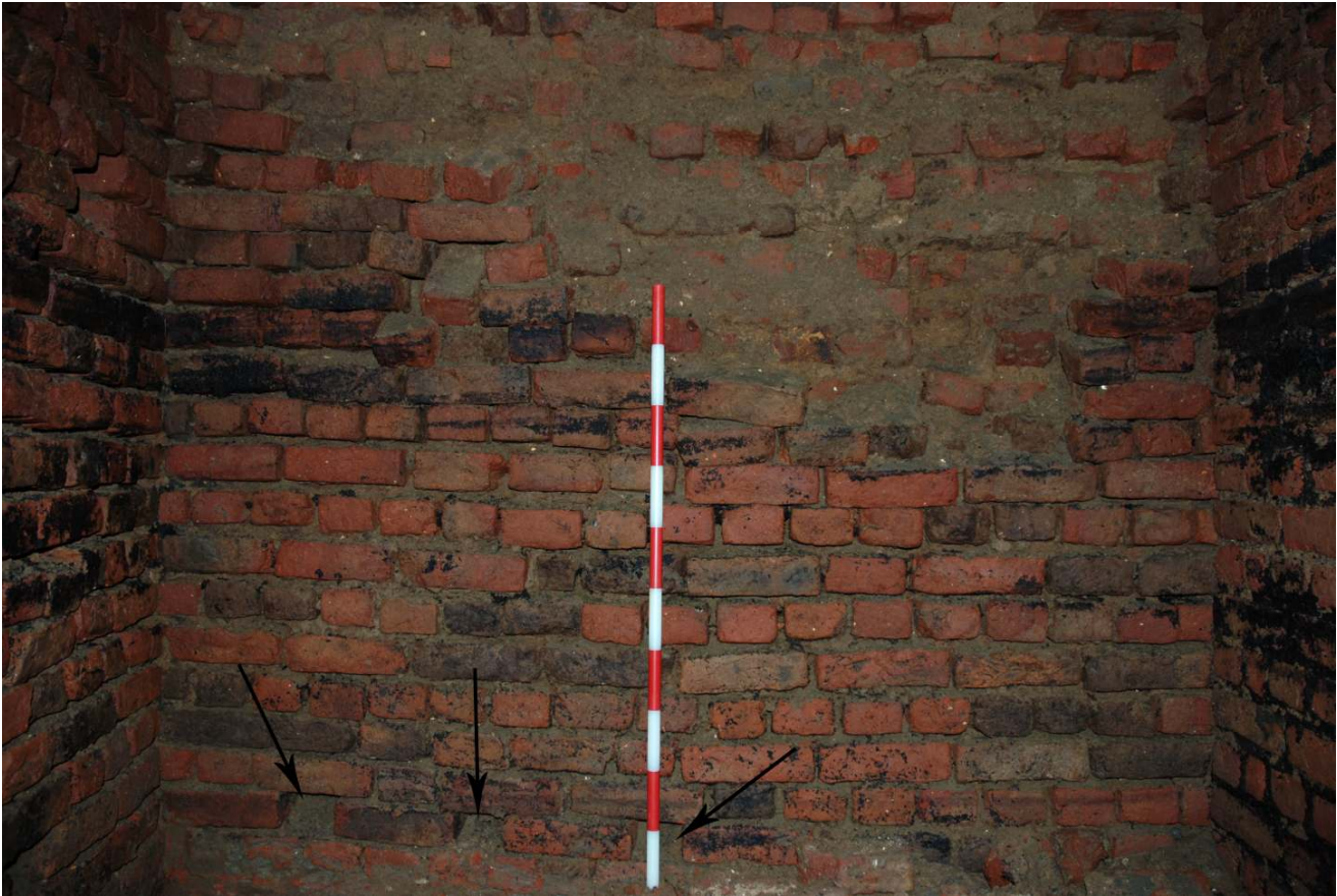
Fig.23: Rear wall showing the three openings near the base of the chamber, the third is visible behind the bottom of the scale, (1m), and measured 320mm deep and continued back. The other two openings are visible to the left. Facing SW
