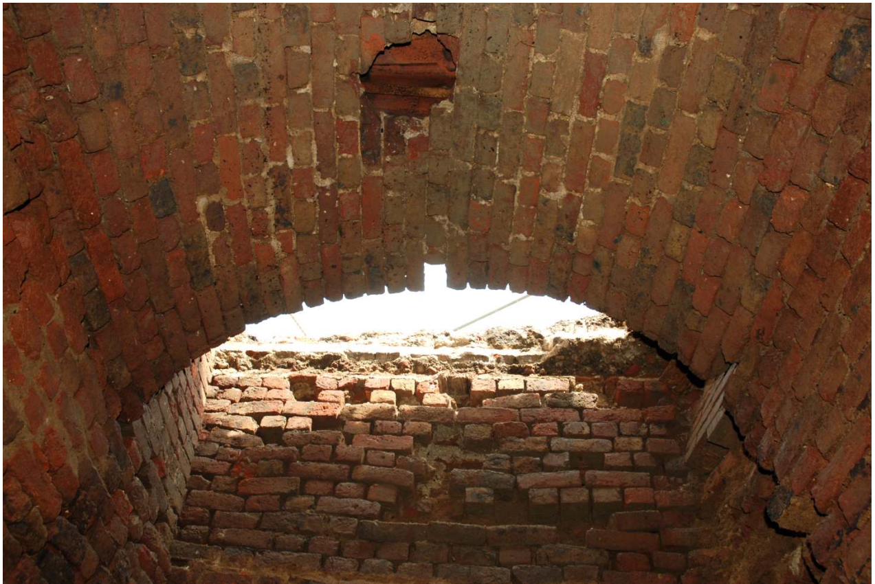
Fig.27: Photograph of the open-ended arched ceiling, taken from the rear wall of the chamber, facing NE. The far spring work of the transverse arch is just visible as a white line towards the top of the front wall. A hole has been crudely patched in the roof with metal slats and pan tiles. The hole does not appear deliberate and there is no sign of a structural feature having been removed. It may have been an earlier case of collapse, or accidental damage
