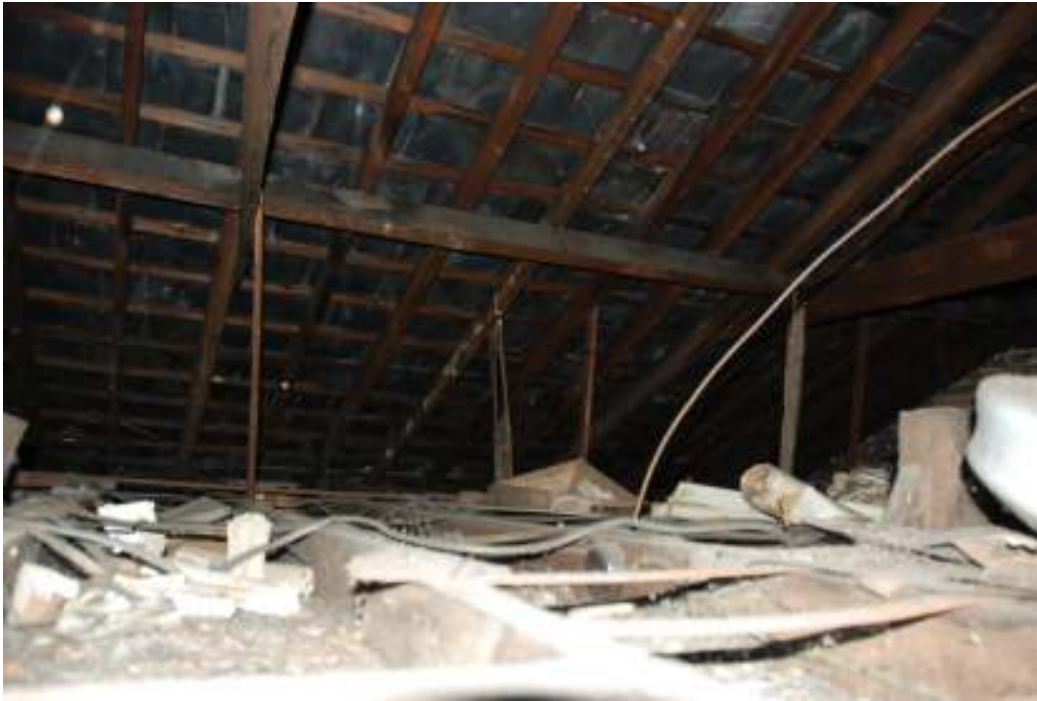
Fig. 45: Photograph of the roof-space above the main building.
