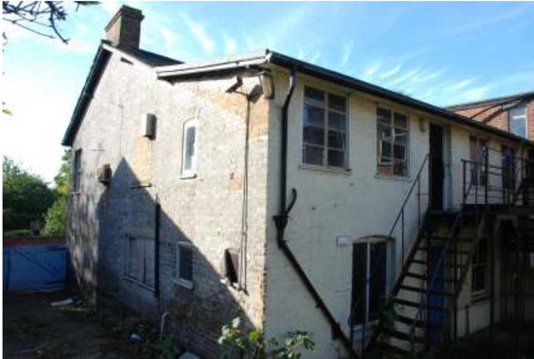
Fig. 51: Photograph of main building, looking south-west, and showing the raising of the roof at the northern end.
