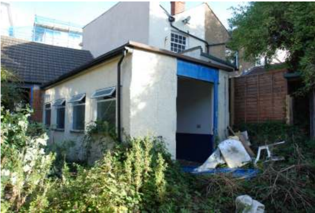
Fig. 77: Photograph of room 1, looking north-east.
