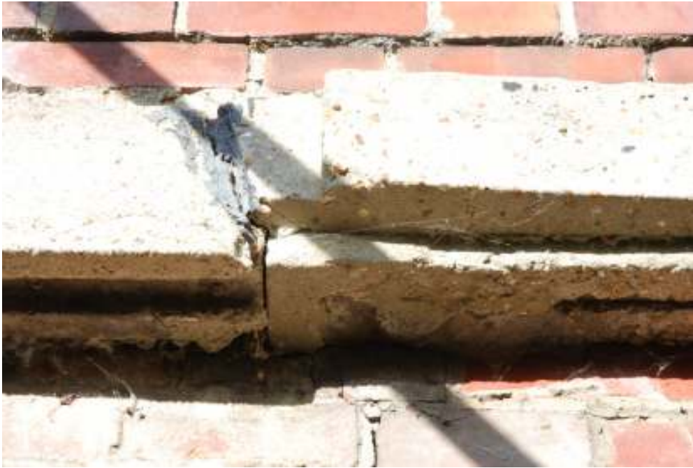
Fig. 102: Photograph of line in concrete where limit of original building was.
