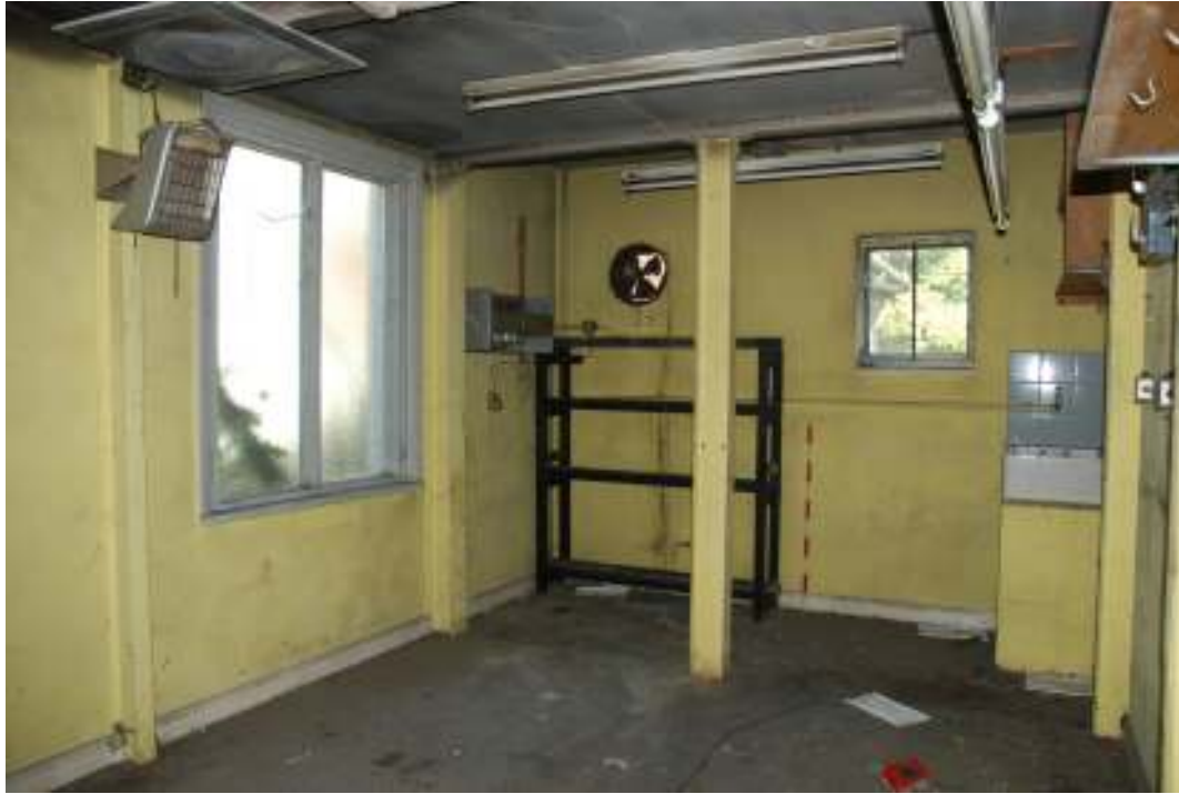
Fig. 56: Photograph of room 31, looking east, showing the modern fixtures and fittings, alongside the shelves for electrical equipment (left of scale) and plug-sockets (right side of image).
