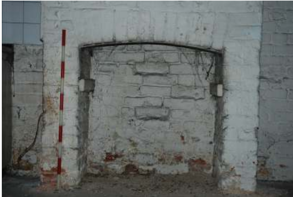
Fig. 37: Photograph of north-eastern fireplace in room 32.
