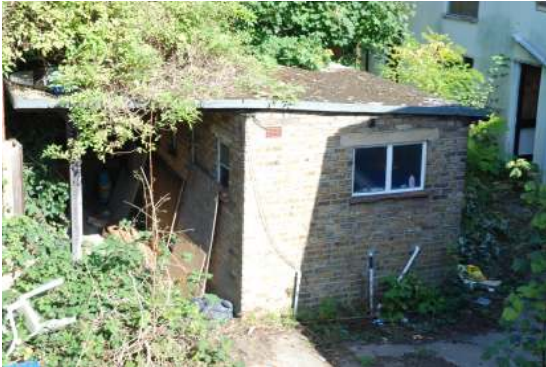
Fig. 120: Photograph of toilet block (rooms 8 – 9) and projecting northern lean-to, looking south-east.
