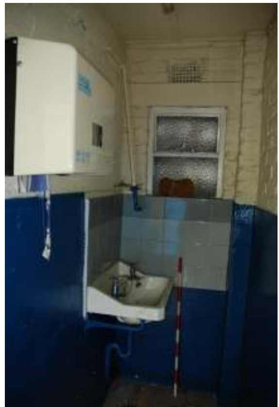
Fig. 119: Photograph of interior of room 9, looking west.
