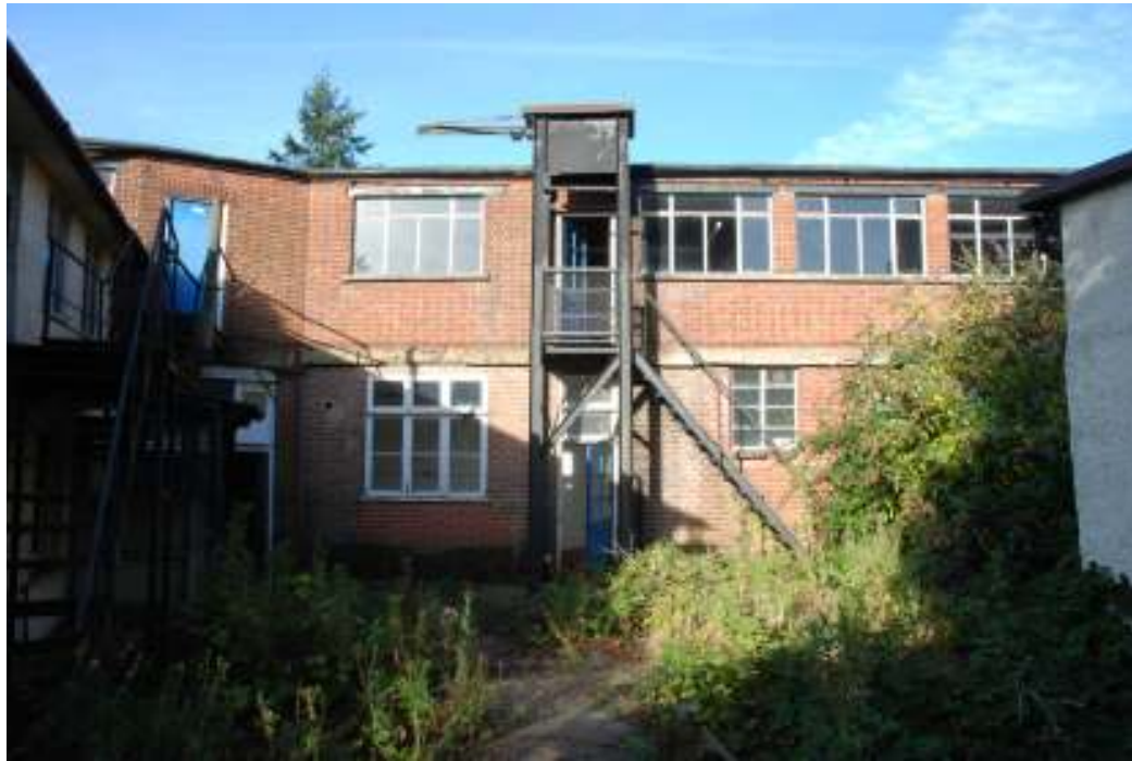
Fig. 111: Photograph of the eastern side of the north-south building, showing how the first-floor is one construction, with the same windows, brickwork, etc.
