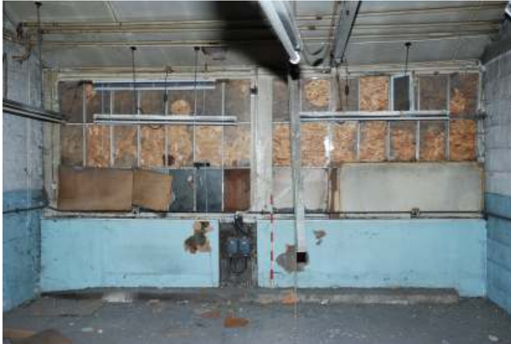
Fig. 89: Photograph of windows in southern wall of room 7, from the inside.
