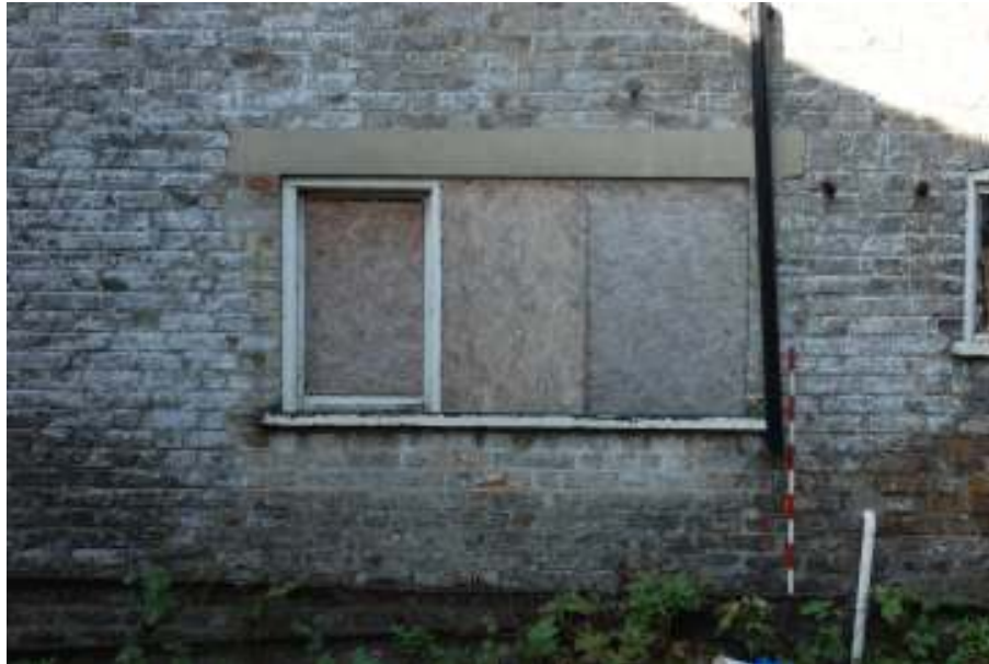
Fig. 60: Photograph of inserted window in eastern wall of main building.
