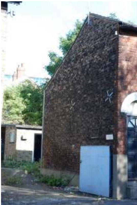
Fig. 18: Photograph of western exterior wall of cottages.
