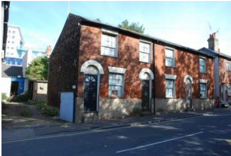
Fig. 17: Photograph of southern frontage of cottages (fronting on to Queen's Road), looking north-west.
