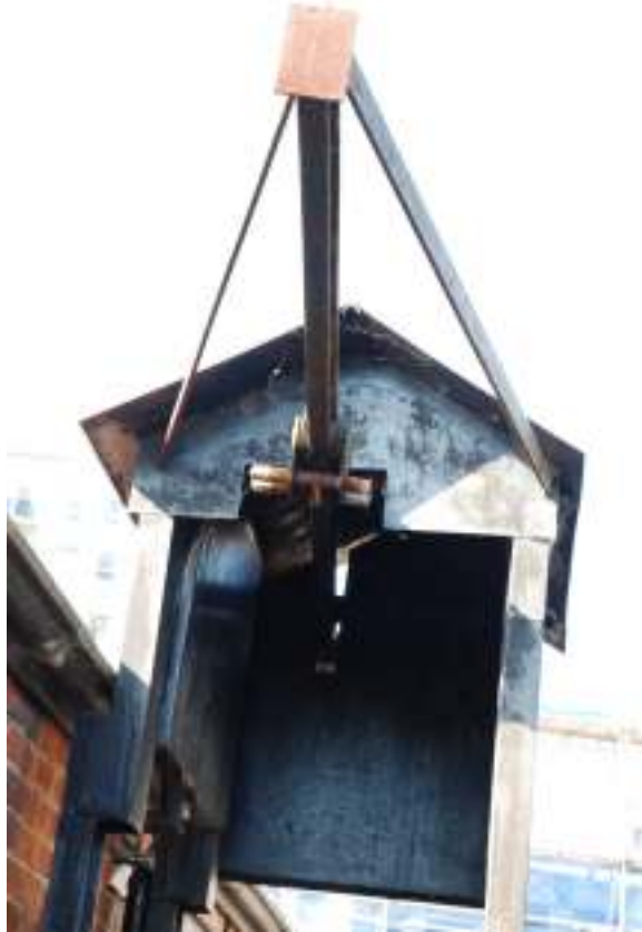
Fig. 114: Photograph of hoist outside room 6.
