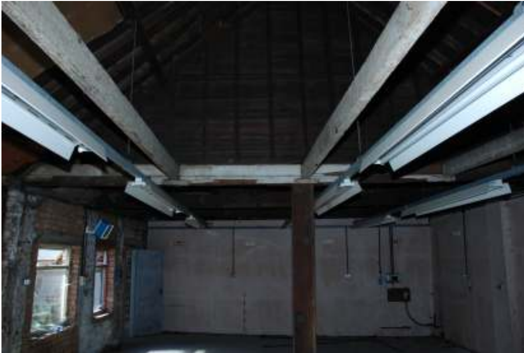
Fig. 72: Photograph of room 2, looking west.
