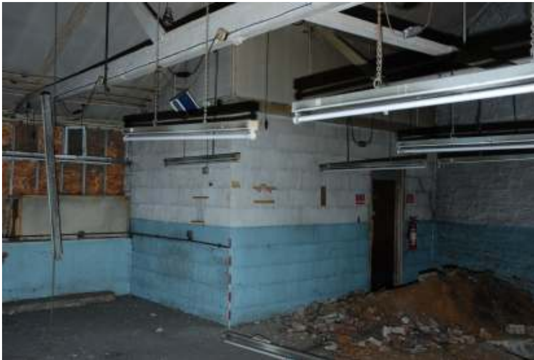
Fig. 91: Photograph of modern breeze-block addition in south-west corner of room 7.
