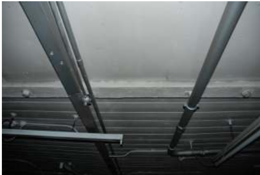
Fig. 39: Photograph of ceiling of room 32, showing the two different ceiling constructions.
