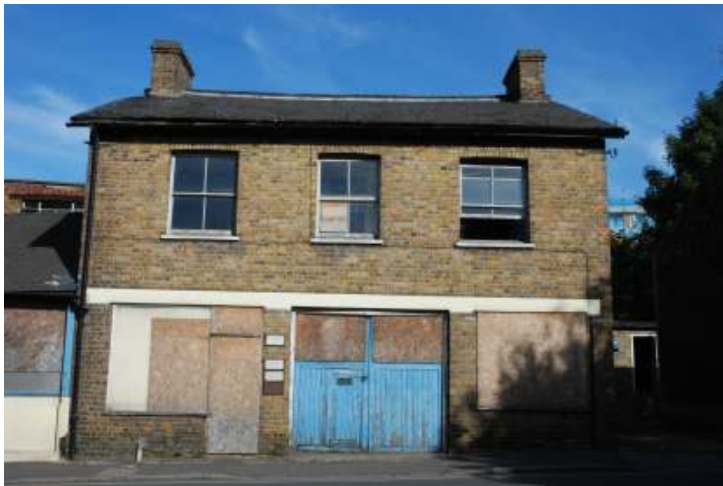
Fig. 50: Photograph of southern frontage of the main building (all inserted alongside the new southern frontage).
