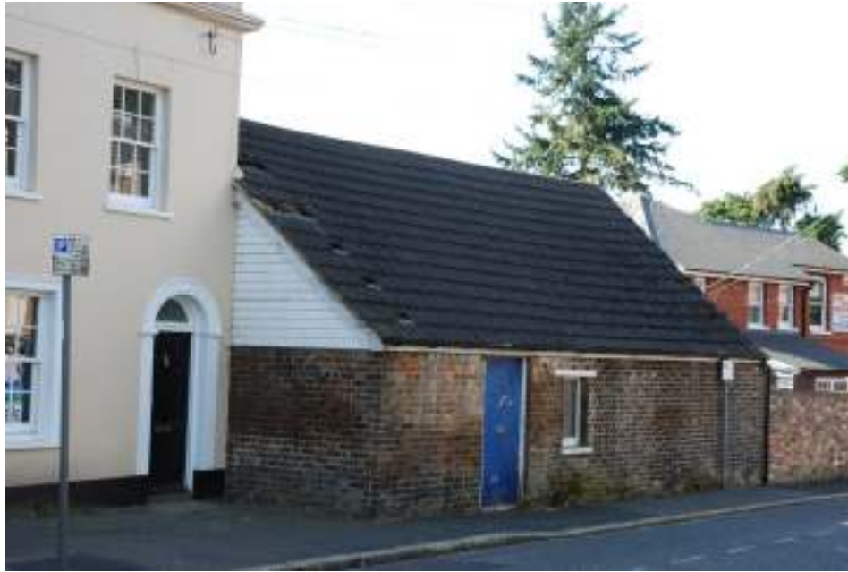
Fig. 65: Photograph of northern wall and northern part of the eastern wall of room 2, looking south-west.
