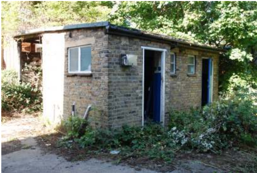
Fig. 117: Photograph of toilet block (rooms 8 – 9), looking north-east.
