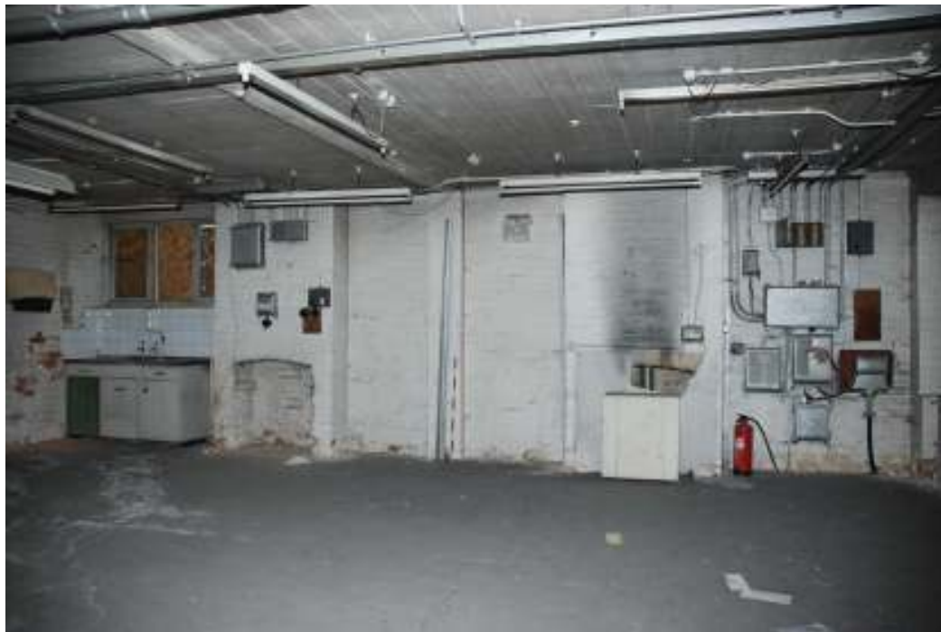
Fig. 36: Photograph of room 32, looking east, and showing its utilitarian nature.
