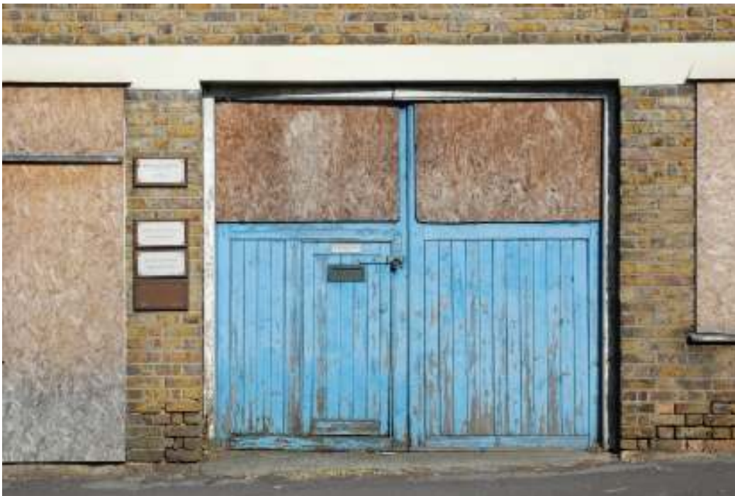
Fig. 49: Photograph of large garage doors in southern frontage of main building.
