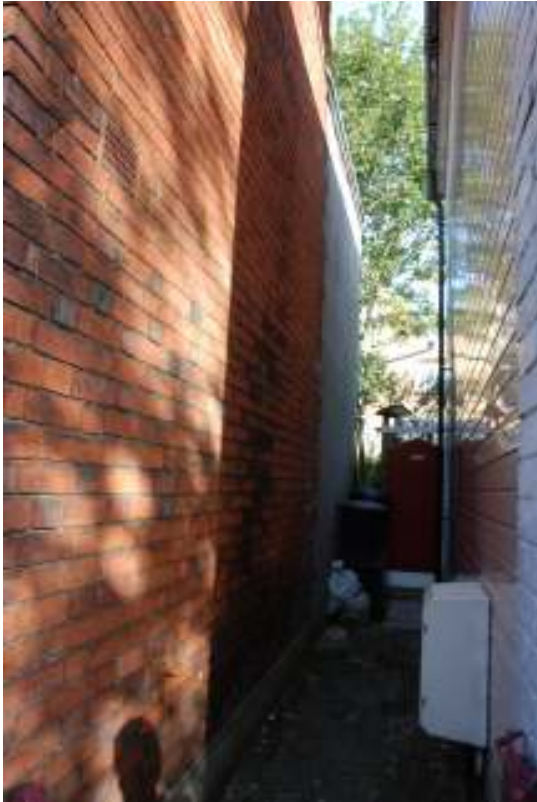
Fig. 19: Photograph of eastern exterior wall of cottages.
