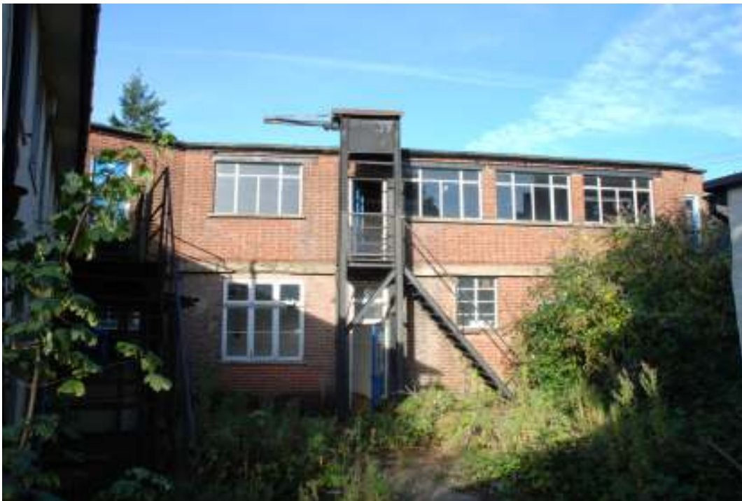
Fig. 103: Photograph of eastern side of north-south building.
