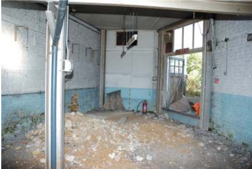
Fig. 97: Photograph of the northern part of room 7, looking north.
