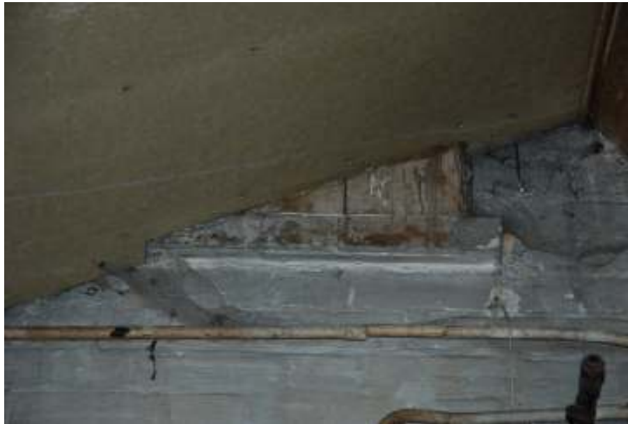
Fig. 86: Photograph of the blocked window in the western wall of the main building, blocked by the roof of room 7.
