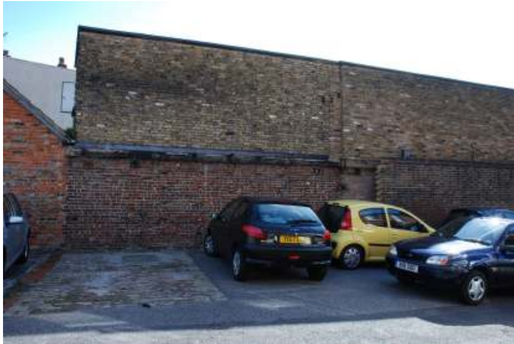
Fig. 100: Photograph of western side of north-south building. The step-back in brickwork, and change in brickwork at the ground-floor level, can be seen behind the yellow car.
