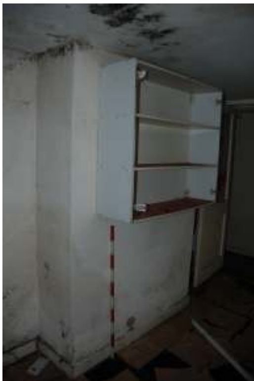
Fig. 22: Photograph of chimney-breast in southern wall of room 15.
