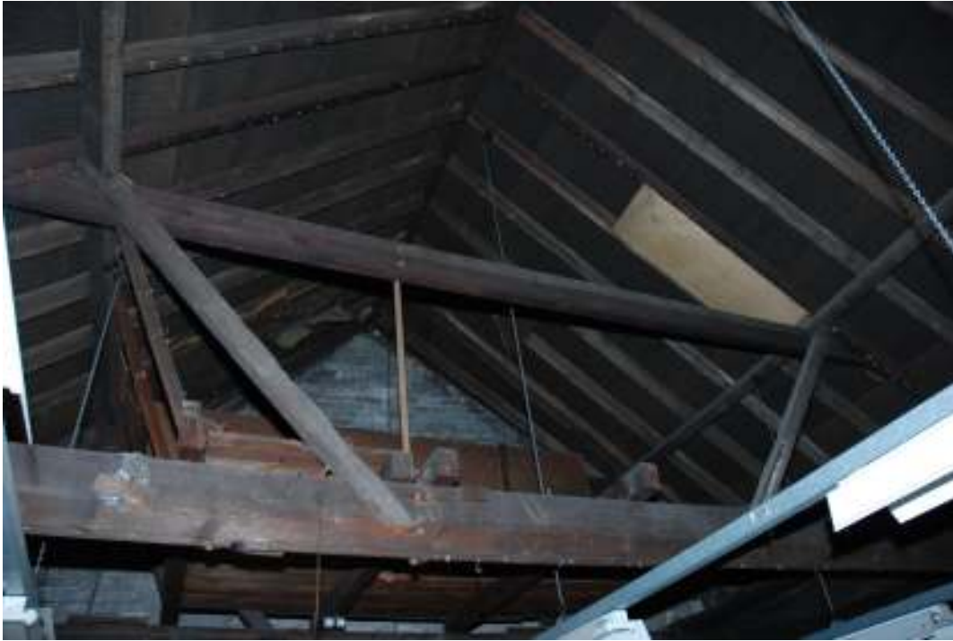
Fig. 70: Photograph of timber-feature (platform holding tank?) in western part of room.
