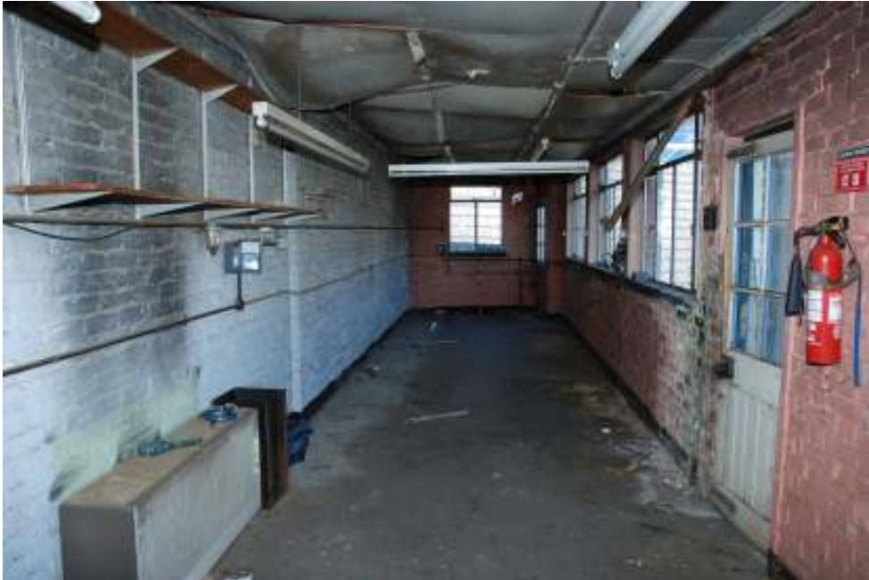
Fig. 112: Photograph of room 6, looking north.
