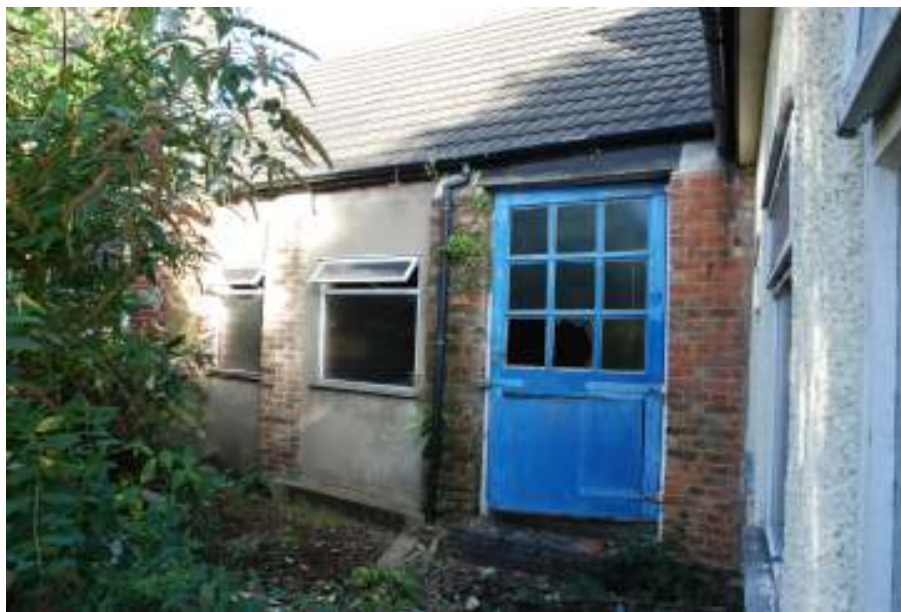
Fig. 63: Photograph of southern wall of room 2 (left of image) and western wall of room 1 (right of image), showing where the room 1 building has simply been built onto the room 2 building.
