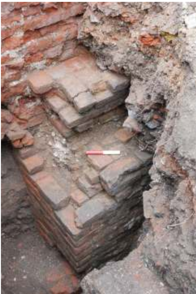
Fig.35: Photo of the eastern basement wall [130], looking south-east, showing its plastered face (immediately behind the 1m scale), and the way it is built up against the earlier wall (behind and at upper level).
