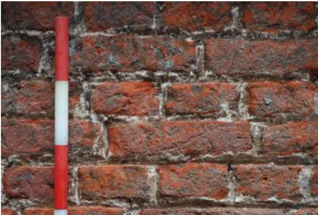
Fig.26: Detail photo of the 16 th century wall within the standing wall in the southern part of site showing the neat pointing. (30cm scale)
