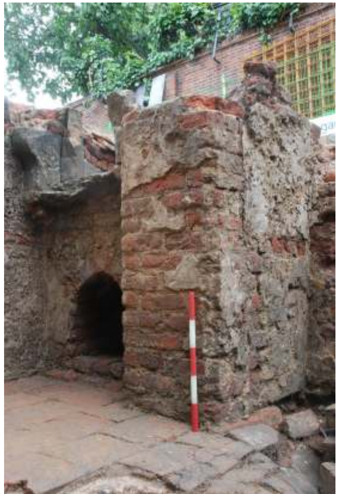
Fig.56: Photo of oven [127], looking north-west. (50cm scale)
