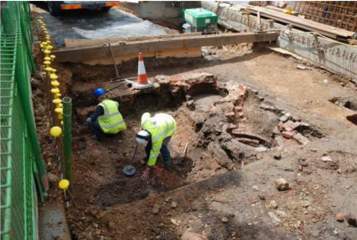
Fig.88: Photo of excavation and investigation of basement infill, looking approximately north-west
