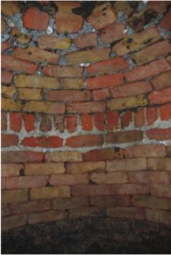
Fig.135: Photo of interior of brick domed well [25]
