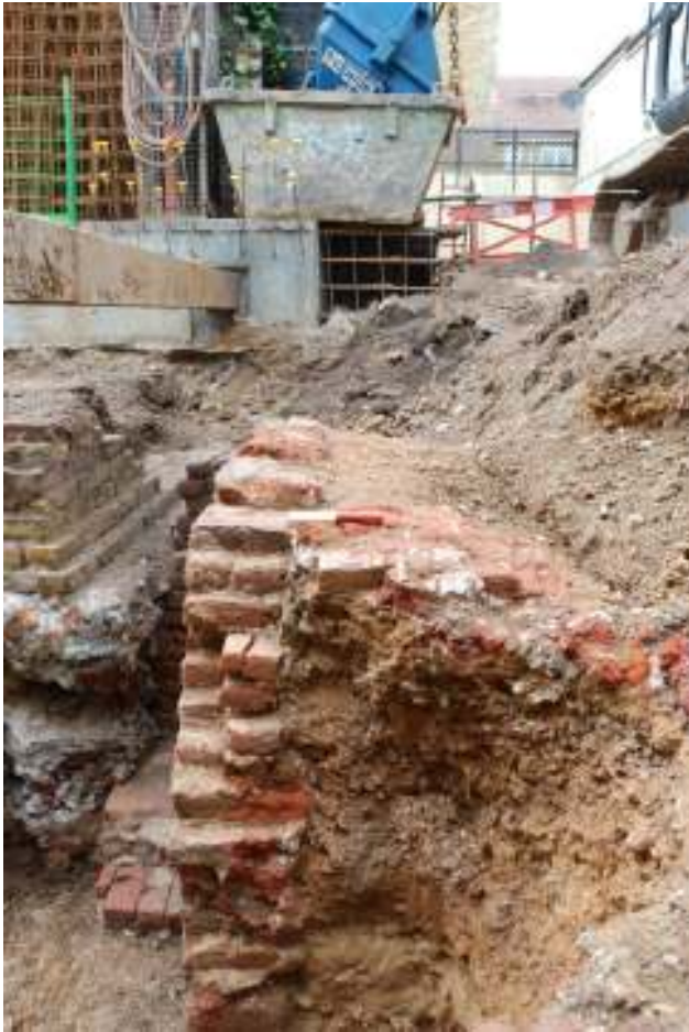
Fig.37: Photo of eastern basement wall [130], and earlier wall [31] to the right, showing how the basement wall was constructed against the earlier wall. (20cm scale)
