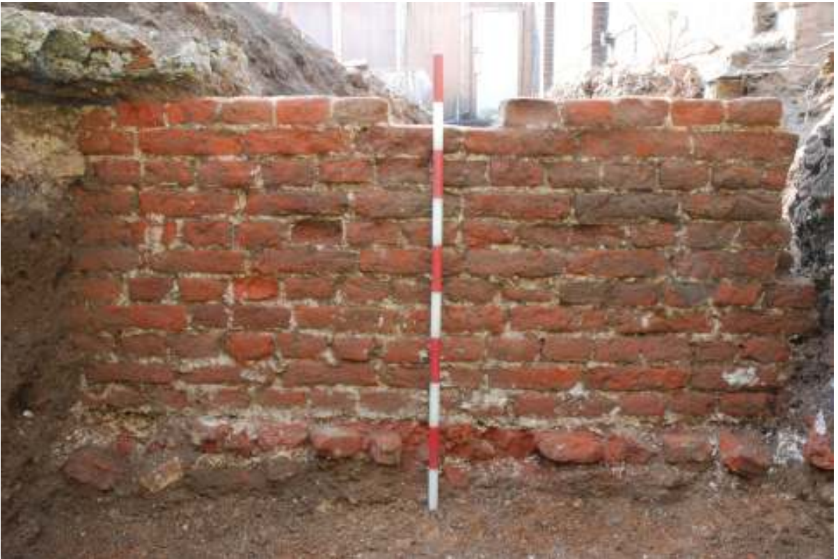
Fig.18: Photo of wall [59] – eastern side. (1m scale)
