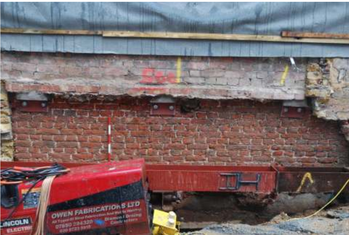
Fig.24: Photo of the 16 th century wall within the standing wall in the southern part of the site. Note the neat pointwork (50cm scale)
