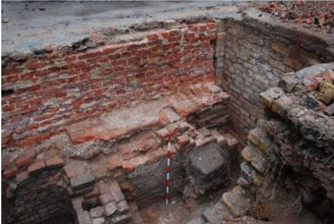
Fig.35: Photo of the eastern basement wall [130], looking south-east, showing its plastered face (immediately behind the 1m scale), and the way it is built up against the earlier wall (behind and at upper level).
