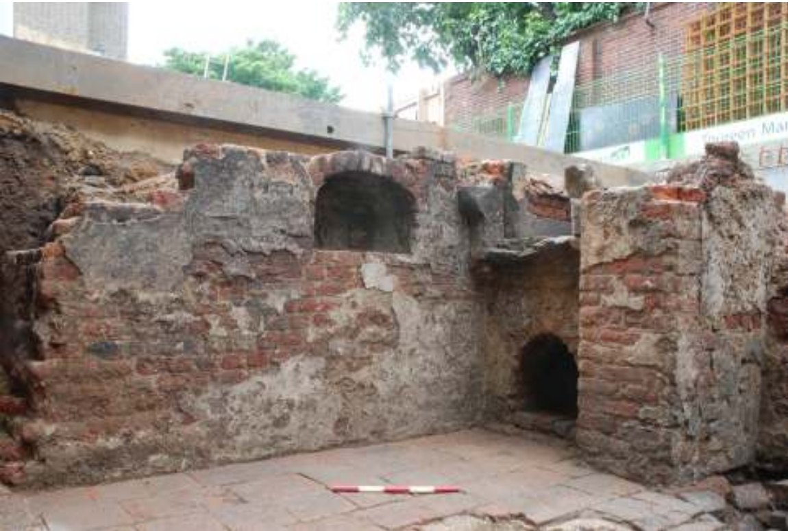
Fig.40: Photo of the western basement wall, looking north-west. (50cm scale)
