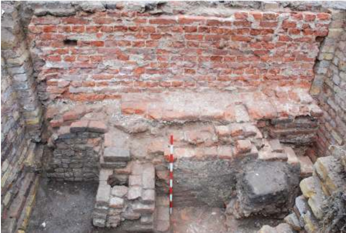
Fig.114: Photo of wall [26] (to the left of the 1m scale), looking east
