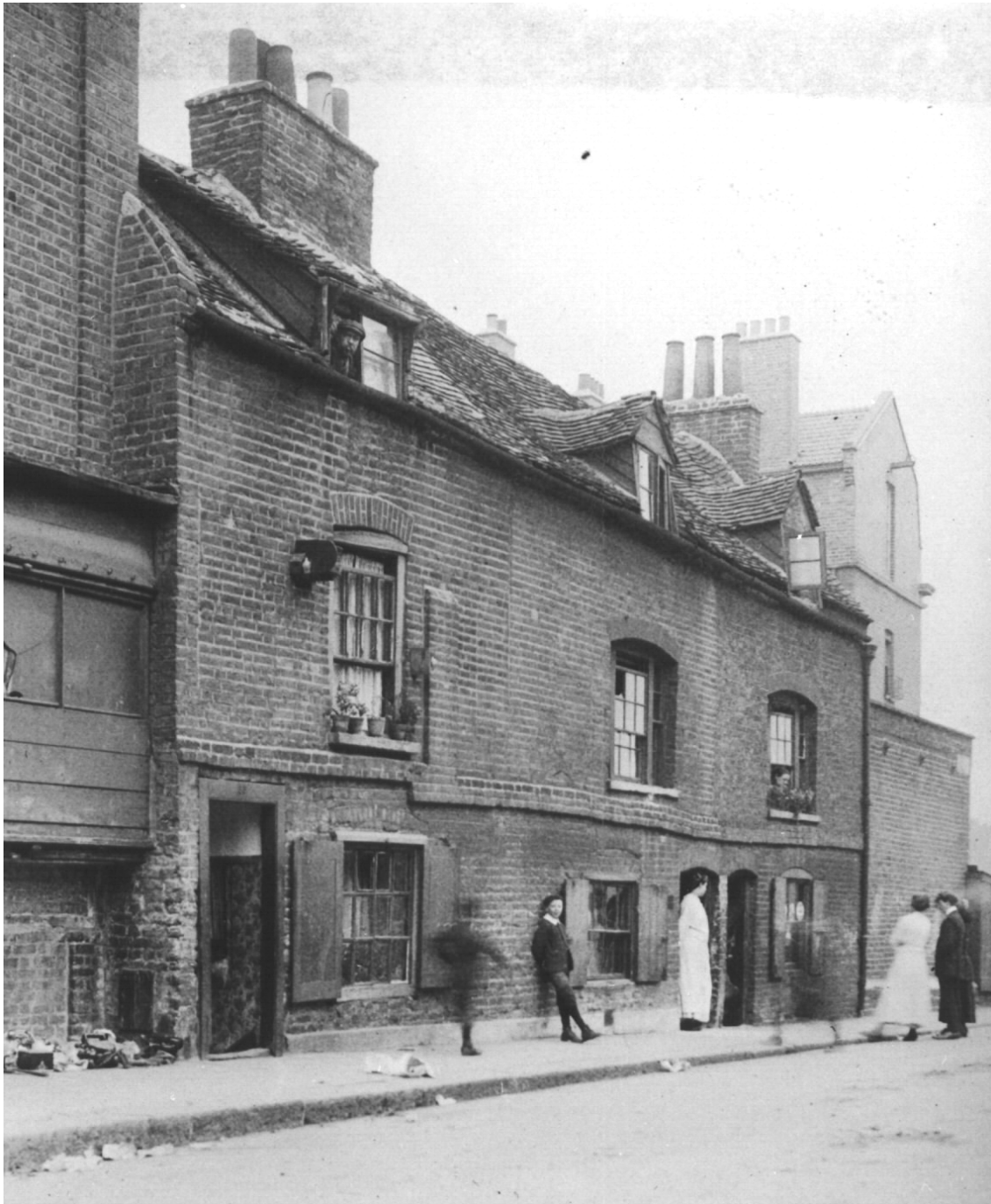
Fig.99: 19 th century photograph of cottages on Milmans Row, looking south. Note the difference between the two cottages to the right and the third in the foreground with different roof tiles, dormer window, main windows and doorway. Also note the wallpaper and skirting board in the doorway of the third cottage appearing to slope as if the entrance steps down from the pavement to internal floor level. © English Heritage, NMR. BB013038.
