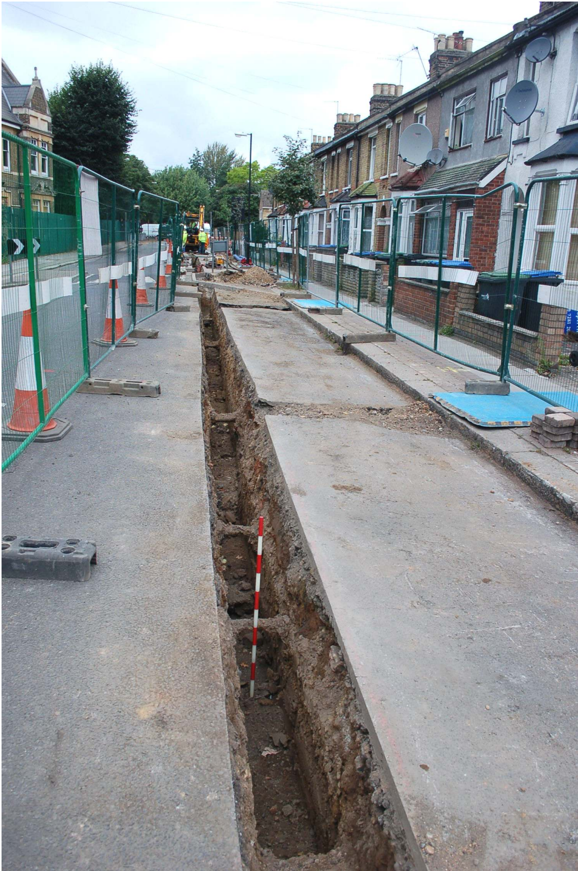
Fig.7: Trenching on Brettenham Road, facing W, (20 th August 2012)
