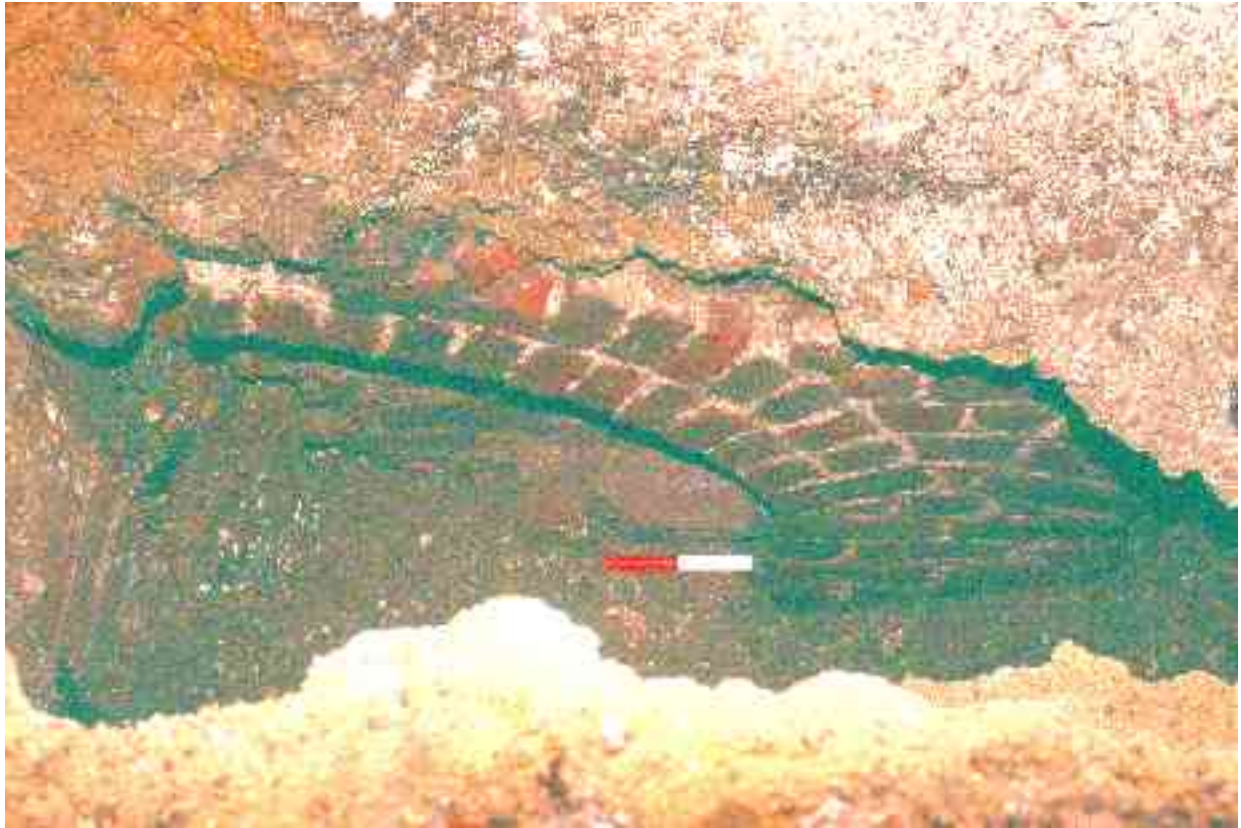
Fig 5 Trench 1, eastern end: view of the blocked brick arch and supporting base as drawn in Figure 4 (0.2m scale)
