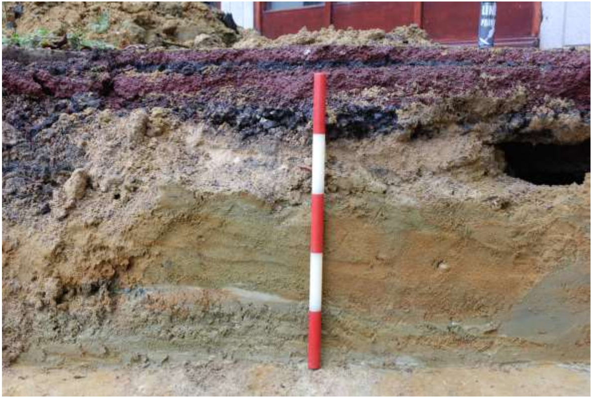
Fig. 26: Photo of northwest-facing section in trench 3
