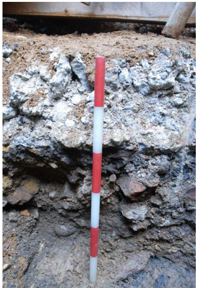
Fig.10: Close-up photograph of the concrete base in shaft 2. The underlying brick rubble deposit, plus the yellow-brown clayey-gravel (the natural deposits), are all visible.
