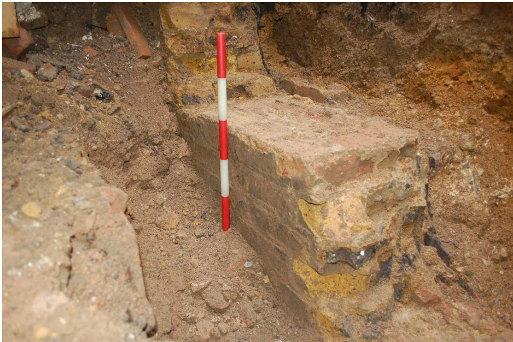
Fig. 8: Photograph of the main wall in shaft 1, looking southwest.
