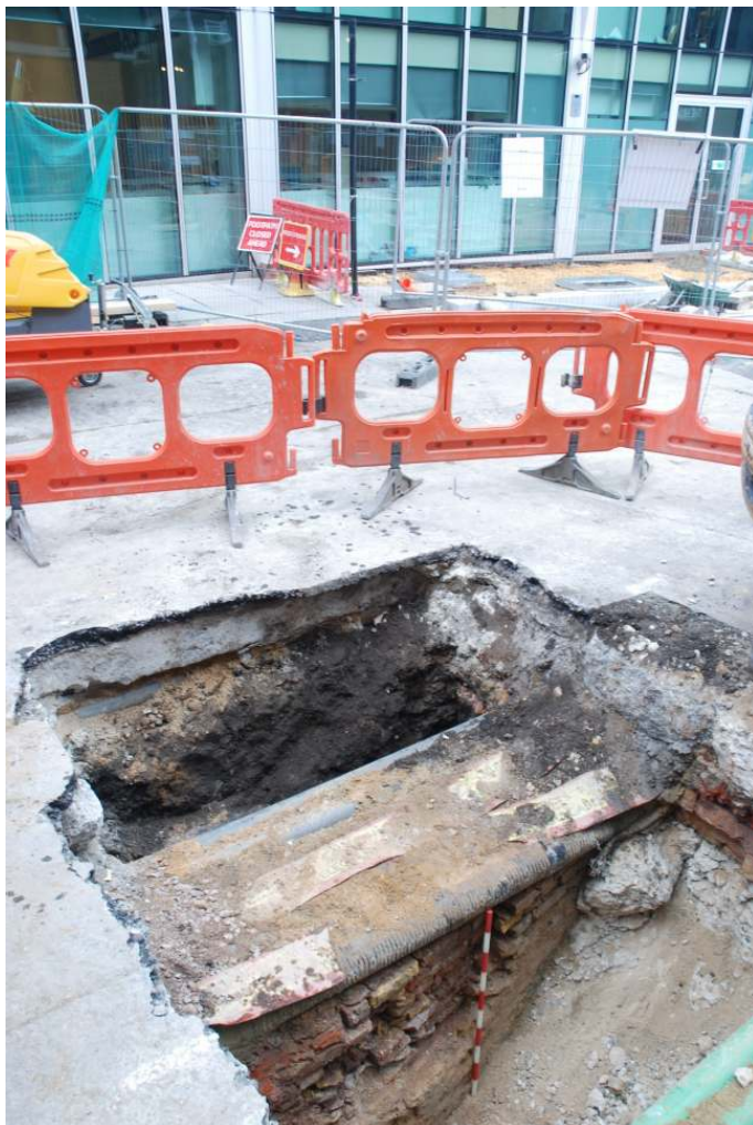
Fig.12: Photograph of shaft 3, looking southeast. The infilled coal cellars and their eastern walls are visible in the foreground, with the loose dark silty deposit in the background.
