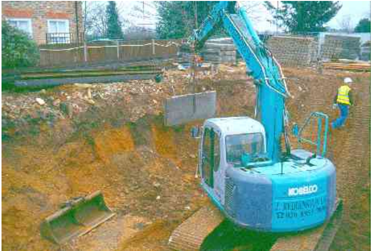
Fig 4 View during the bulk excavation, looking northeast toward the Common
