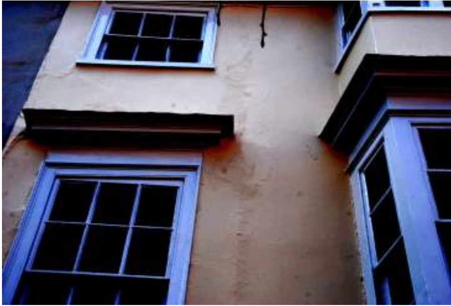
Fig.44: Photo (with enhanced contrast) showing the line on the exterior front wall between the original part of the building and the rooms above the passageway
