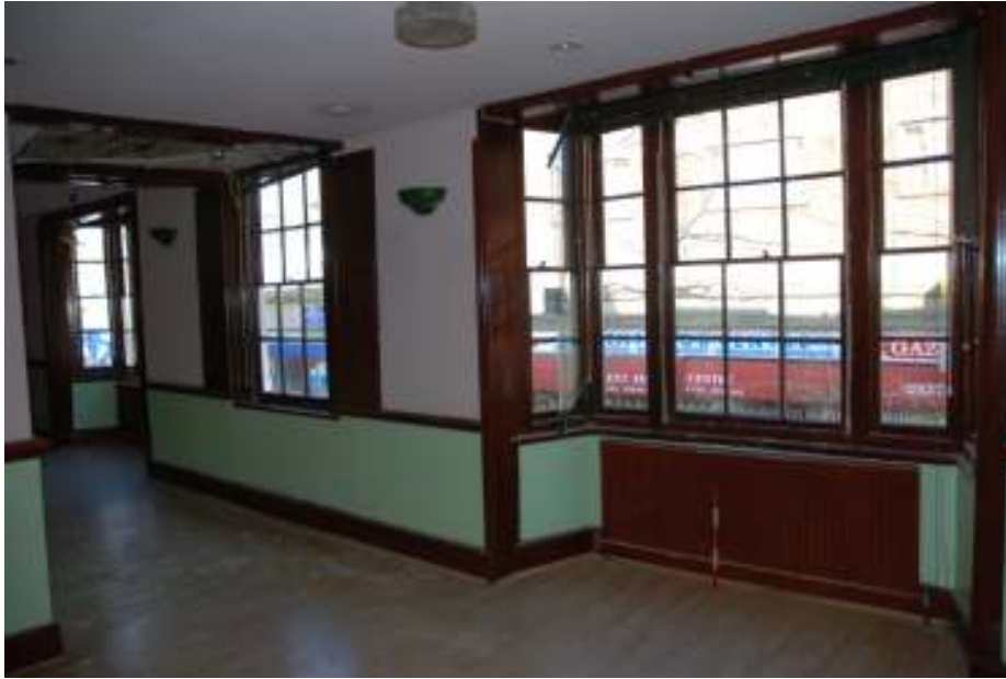
Fig.51: Photo of bay-windows in rooms 1 and 2 on the first-floor, looking north-east
