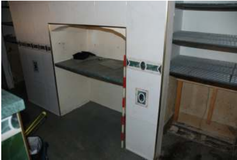
Fig.21: Photo of fireplace opening in room 1
