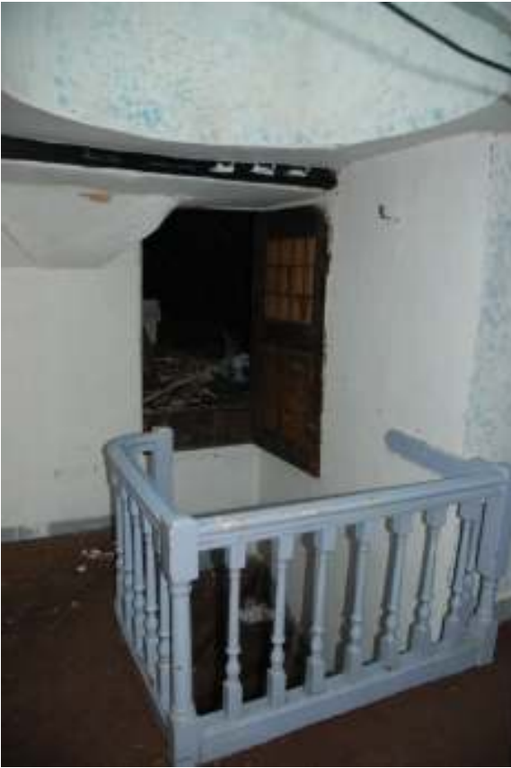
Fig.27: Photo of the top of the winder staircase leading from the first to the second-floor
