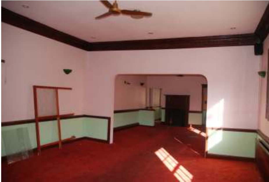
Fig.30: General photo of room 5, within the western extension, looking east
