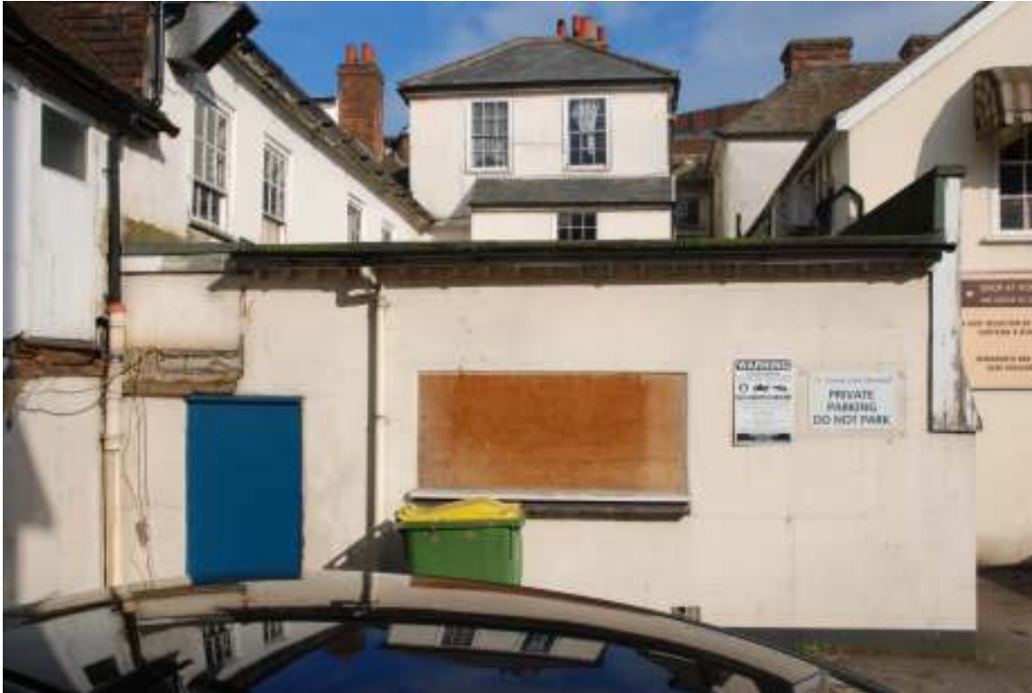
Fig.69: Photo of the flat-roofed ground-floor area, looking east
