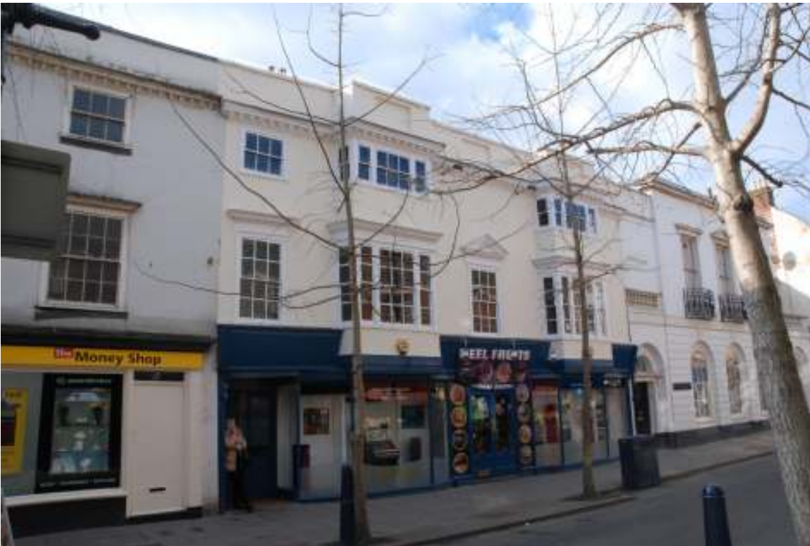
Fig.48: Photo of the frontage of the building, looking north-west
