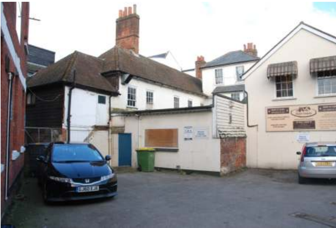
Fig.29: Photo showing the western extension (the long range, with chimney at this end), looking north-east
