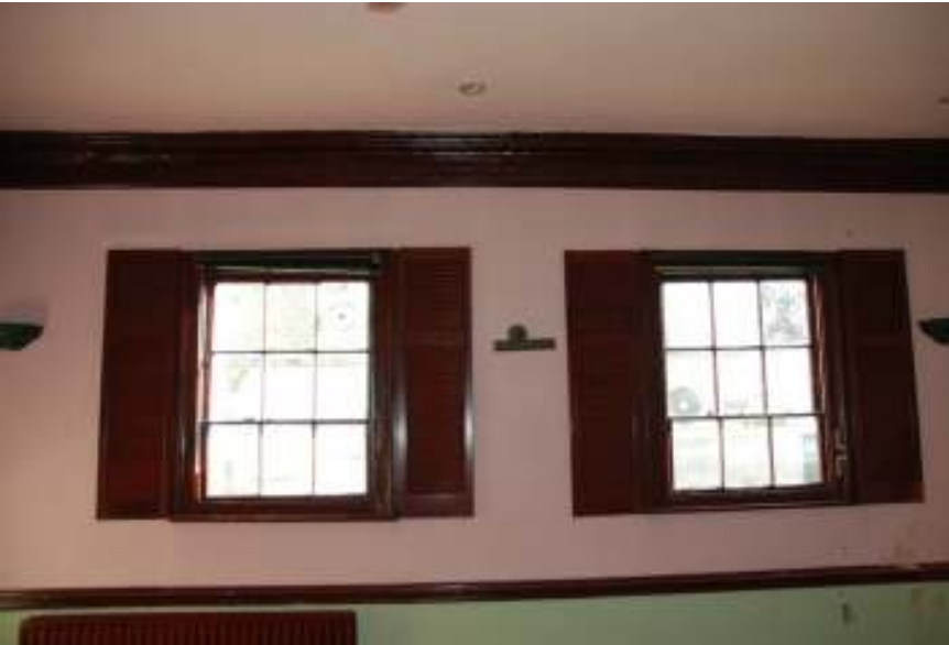
Fig.39: Photo of windows in room 5
