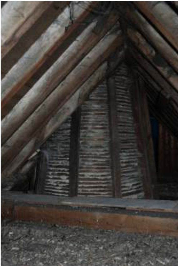
Fig.42: Photo of the lathe-and-plaster skylight, in the roof-space
