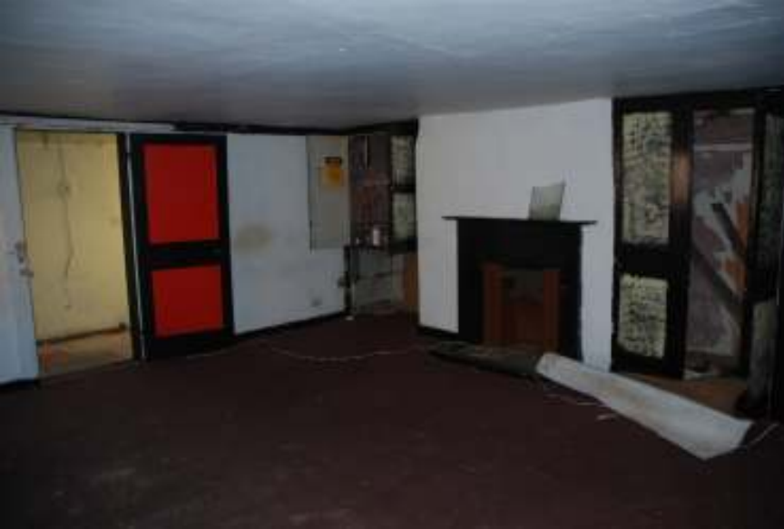
Fig.15: Photo of room 13, looking south-west
