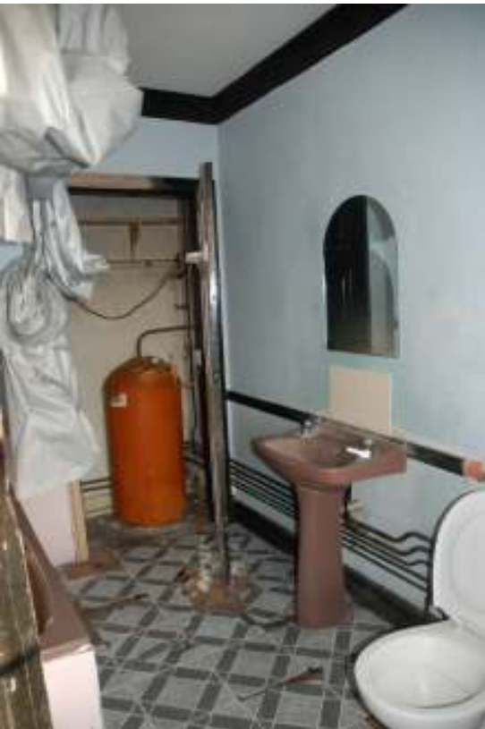
Fig.62: Photo of room 18, in the second south-western extension, looking east
