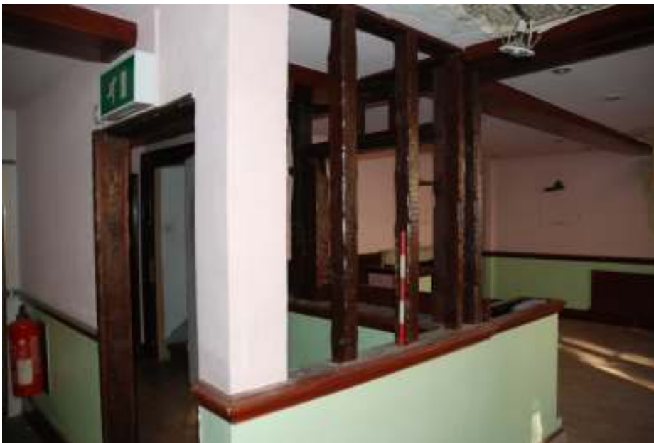
Fig.28: Photo of pieces of reused timber in the entrance to rooms 1 and 2
