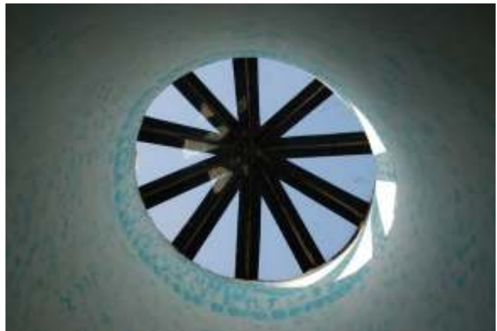
Fig.41: Photo looking up at the skylight
