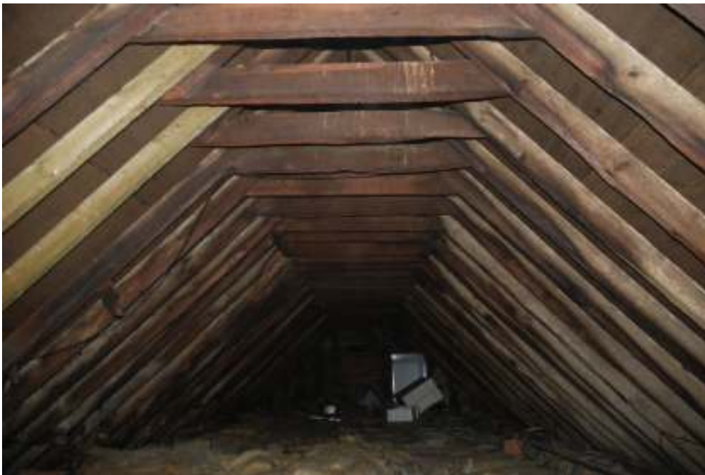
Fig.33: Photo of the roof-structure in the western extension, looking west
