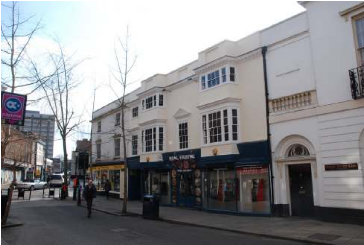
Fig.49: Photo of the frontage of the building, looking south-west
