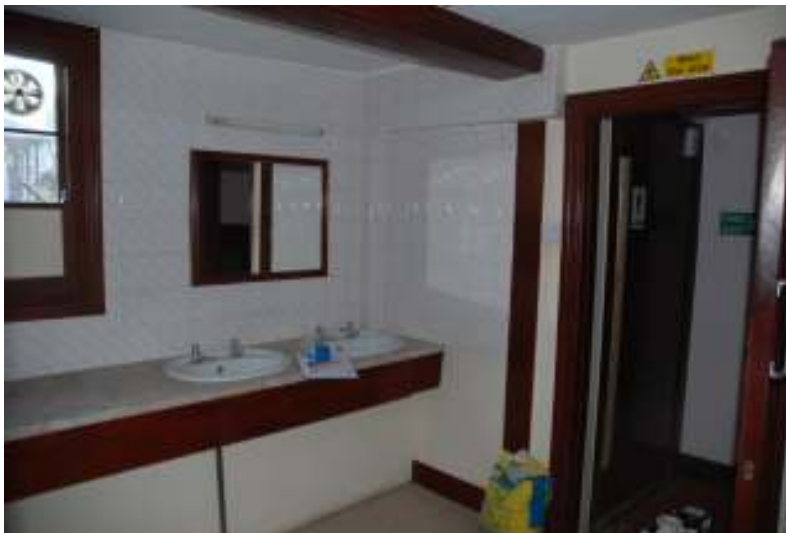
Fig.60: Photo of room 12, in second south-western extension, looking north-west
