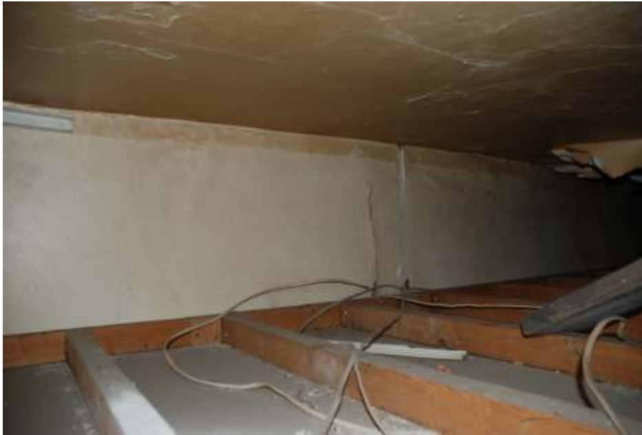
Fig.32: Photo through the ceiling of room 7, showing the original higher ceiling
