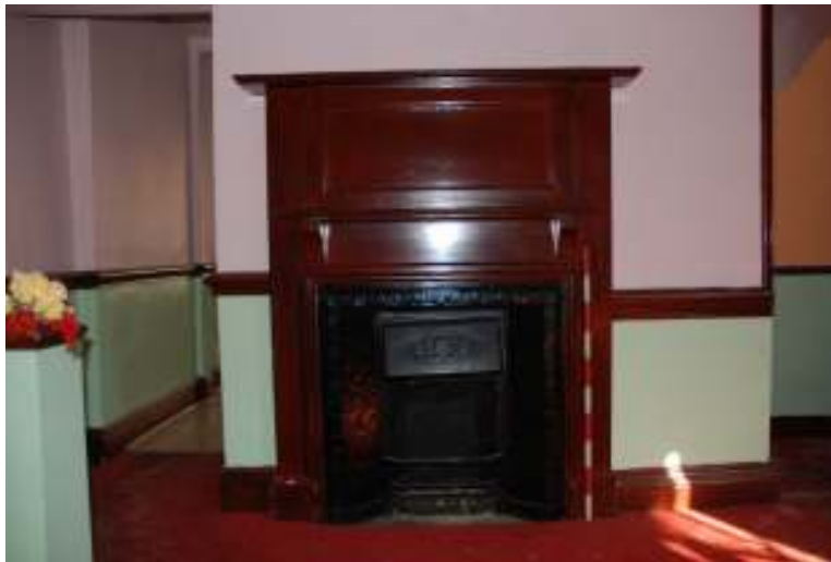
Fig.36: Photo of the extant fireplace at the eastern end of room 5
