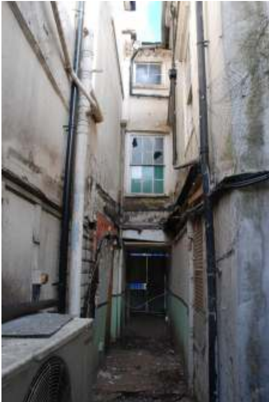
Fig.45: Photo of rooms over the passageway, looking east
