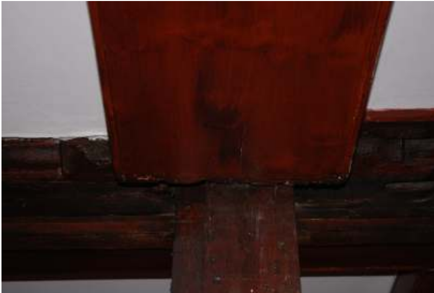
Fig.24: Photo of the moulded ceiling beam running east-west between rooms 1 and 2 (running left to right across the image)
