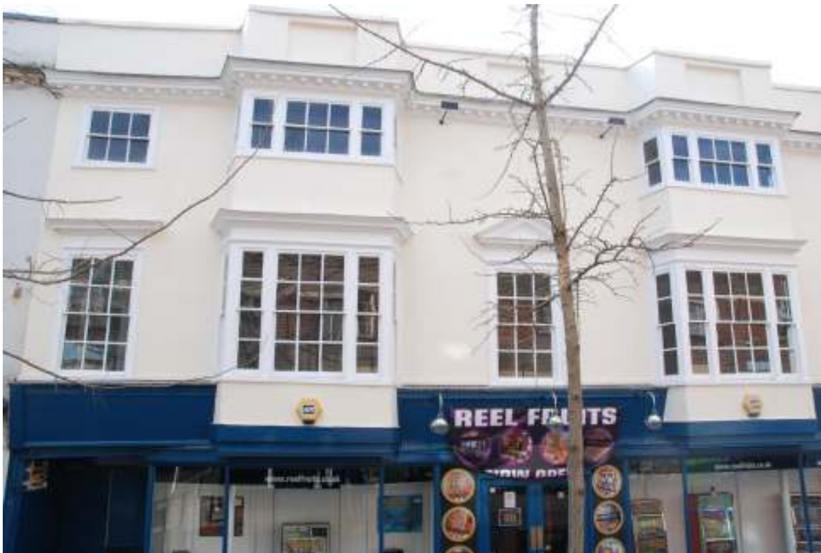
Fig.50: Photo of the frontage of the building, looking west
