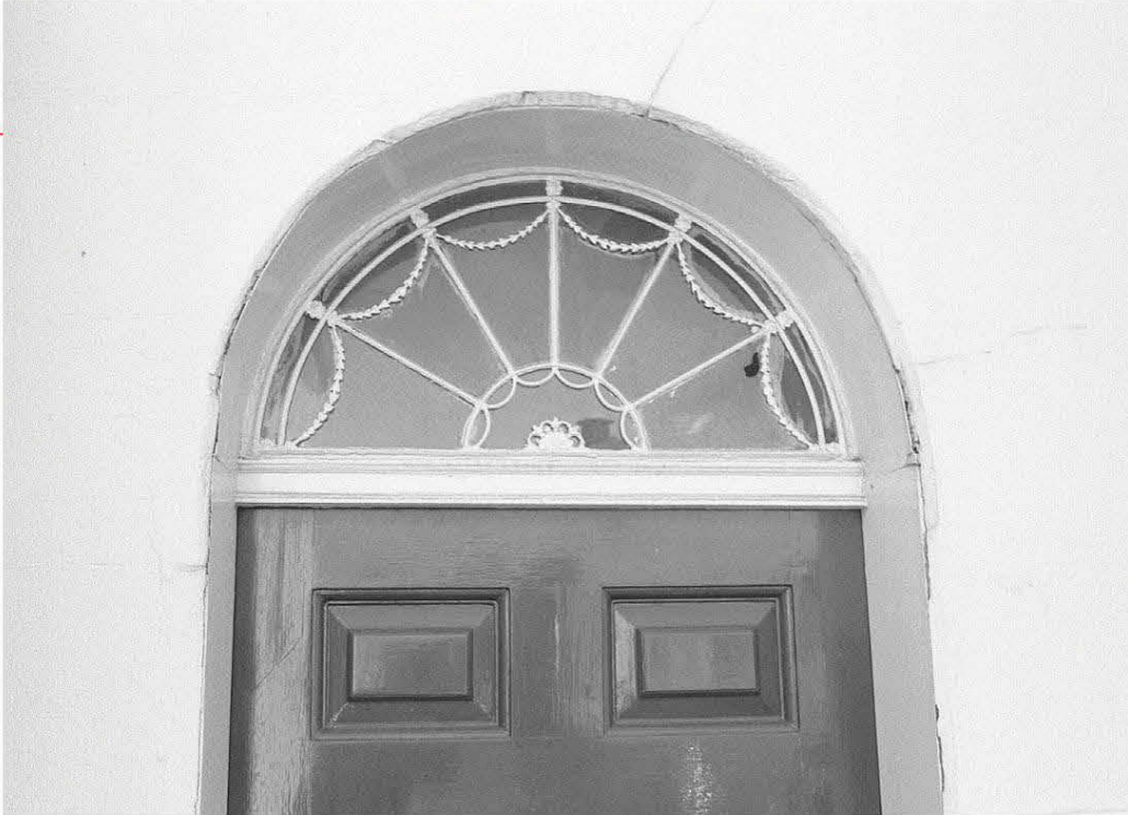
Fanlight of radiating pattern over the main entrance door, measuring c 980mm x 480mm
