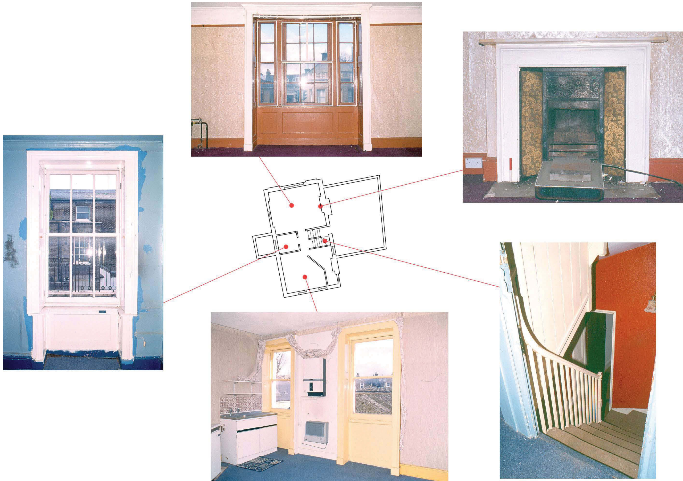
Fig 19 First floor internal views, including sash windows with shutters and a later cast iron and tiled fireplace inserted into the front room
