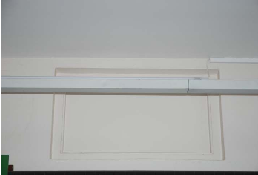
Fig.27: Small high-level blocked-up opening on southern side of room 3
