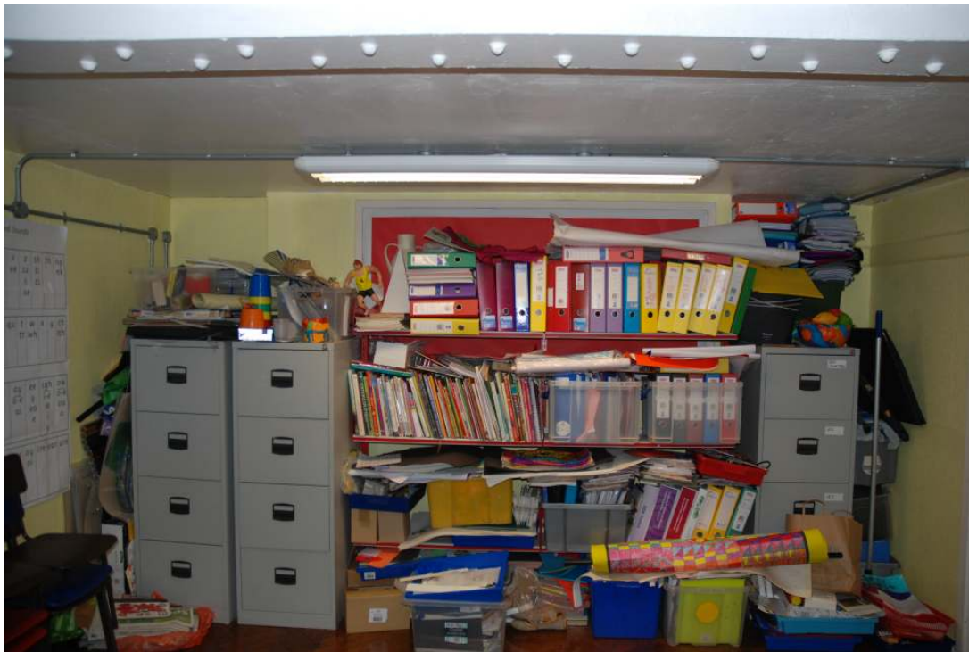
Fig.65: Mezzanine level 2B, looking east, showing the blocked fireplace wall and riveted cross-beam in foreground
