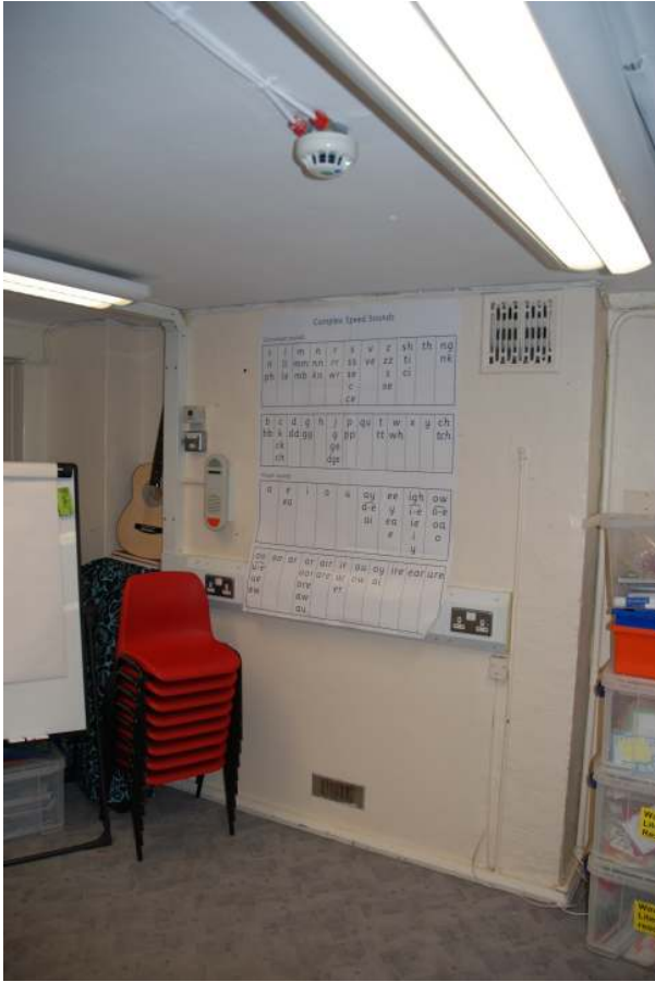
Fig.68: The blocked fireplace on eastern wall of mezzanine level 1A
