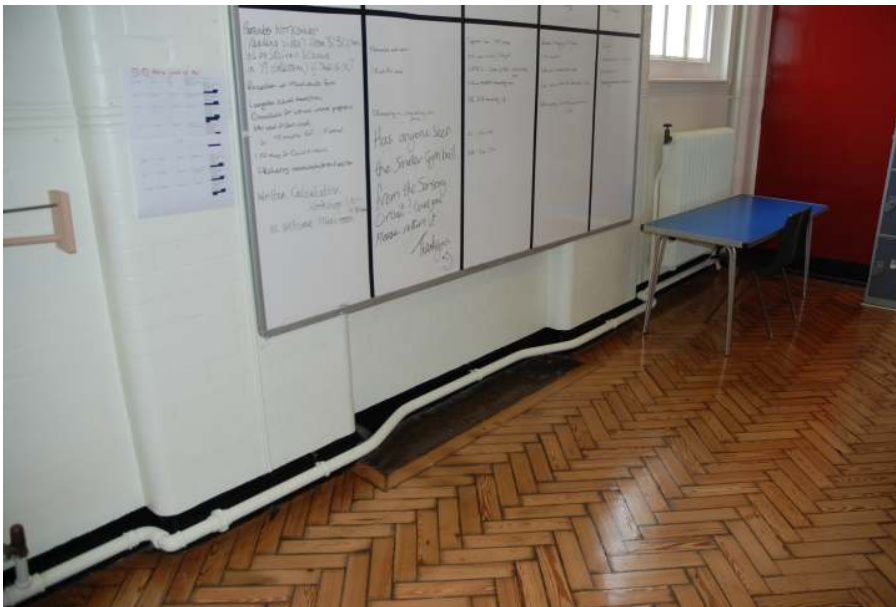
Fig.28: Original position of one of the radiators in room 3
