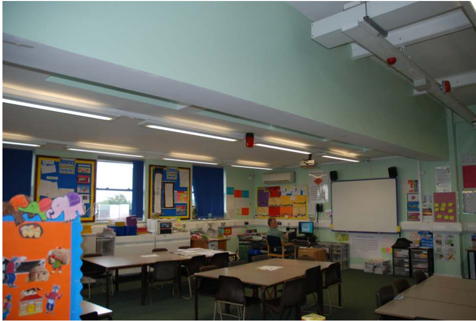
Fig.45: Room 6, looking north-east (towards the modern extension), showing the beam running across and separating the modern extension from the older part
