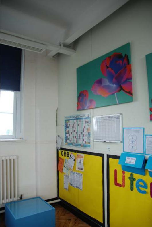
Fig.39: The later chipboard wall between rooms 3 and 4
