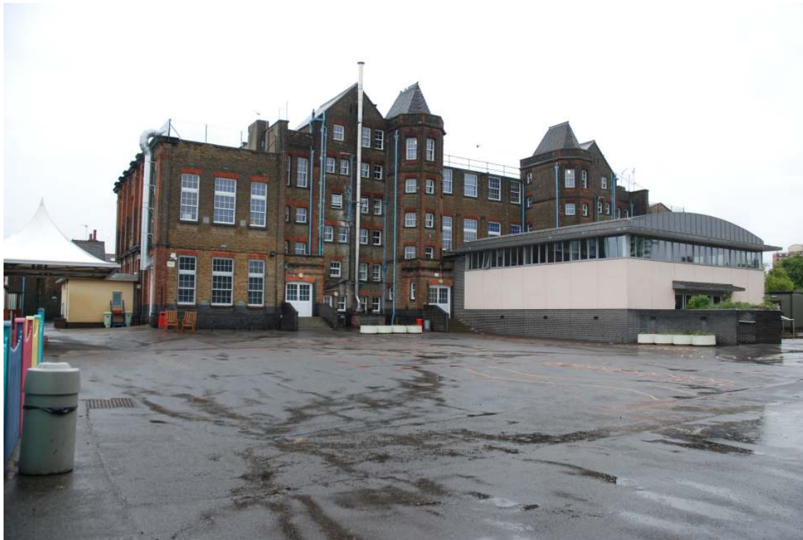
Fig.47: The southern elevation, showing the existing gables towards the centre of the building
