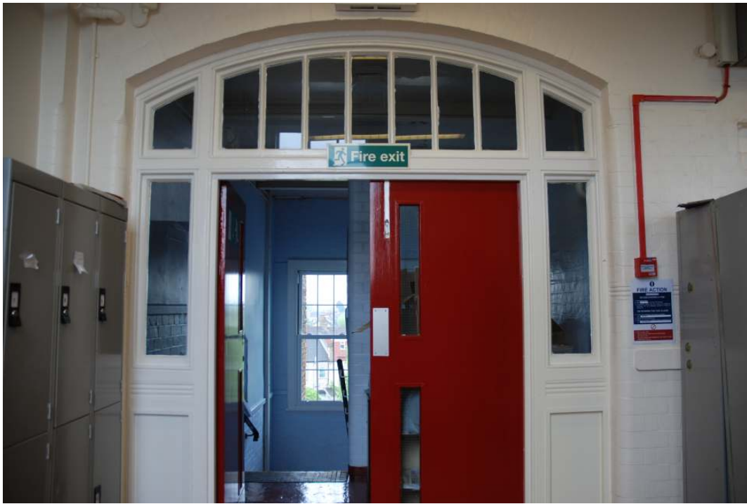
Fig.25: Original doorway and glass panelling in the eastern part of room 3, leading to the stairs
