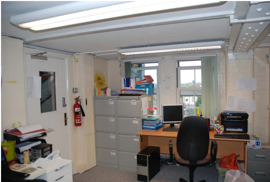
Fig.61: Mezzanine level 2A, looking south, showing the area of the proposed new lobby
