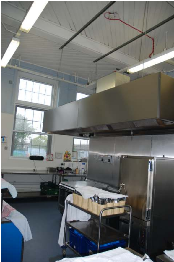
Fig.54: Room 15, looking south-west, and showing the original windows
