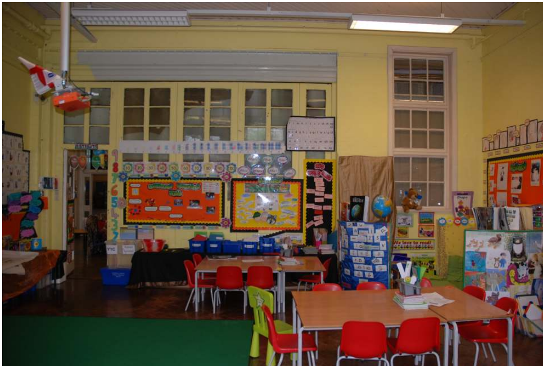
Fig.70: The southern wall of room 13, showing the original doorway, overhead light, and adjacent windows into hall / corridor
