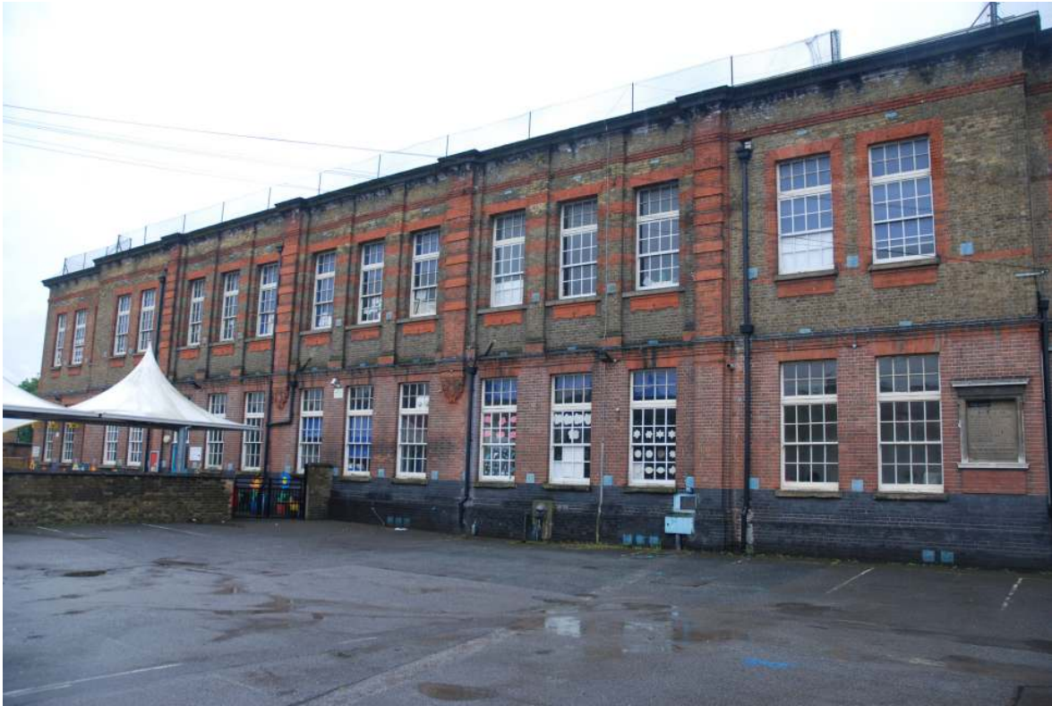
Fig.46: The northern elevation, showing the flat roof
