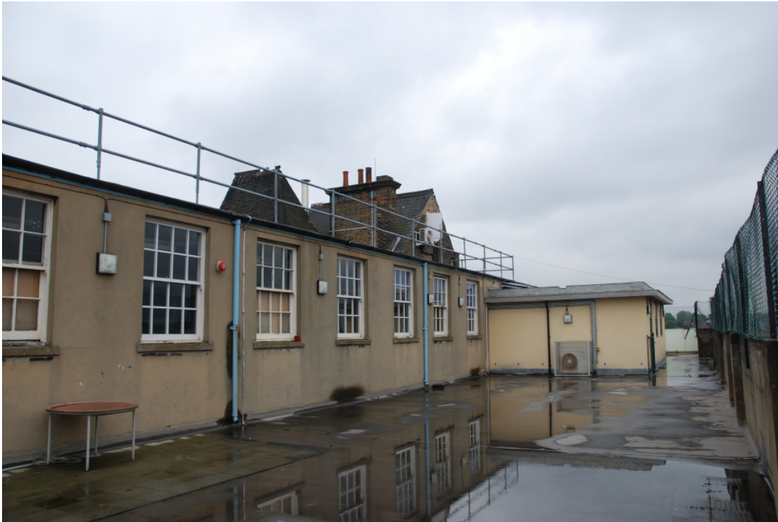
Fig.42: The modern extension, looking south-west
