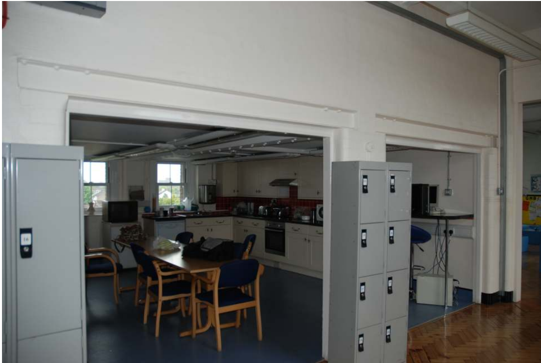
Fig.29: Room 2, looking south-west, through openings that would originally have held a pair of double doors
