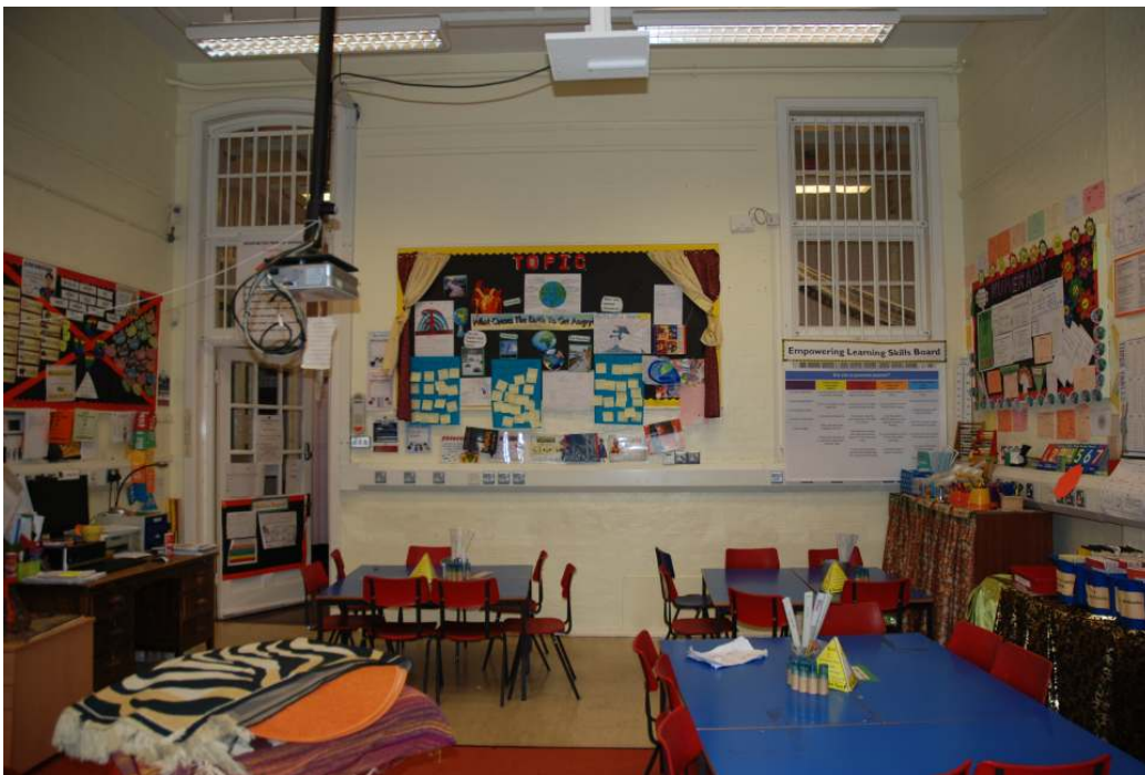
Fig.74: The southern wall of room 9, showing the original doorway, overlight, and internal window to the west
