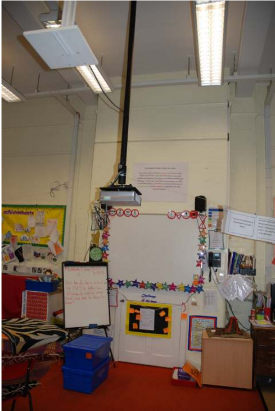
Fig.77: The blocked fireplace in the eastern wall of room 9
