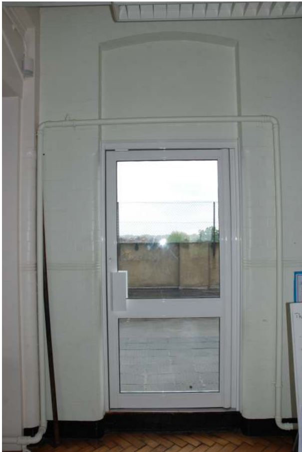
Fig.23: The modern door in the original doorway opening in the northern wall of room 3
