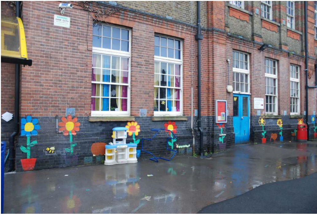
Fig.53: Part of the northern frontage of the building, showing the area of the proposed new door (left of image), and the existing door with overlying window light (right of image)
