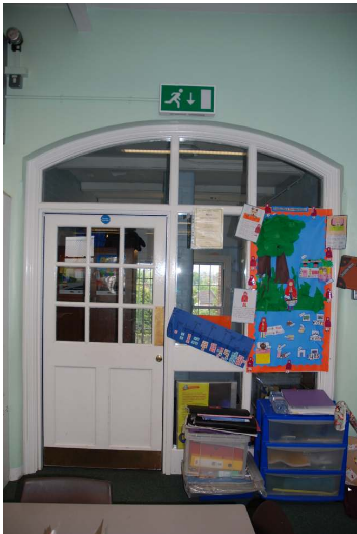
Fig.26: Later doorway and glass panelling in the south-western corner of room 6
