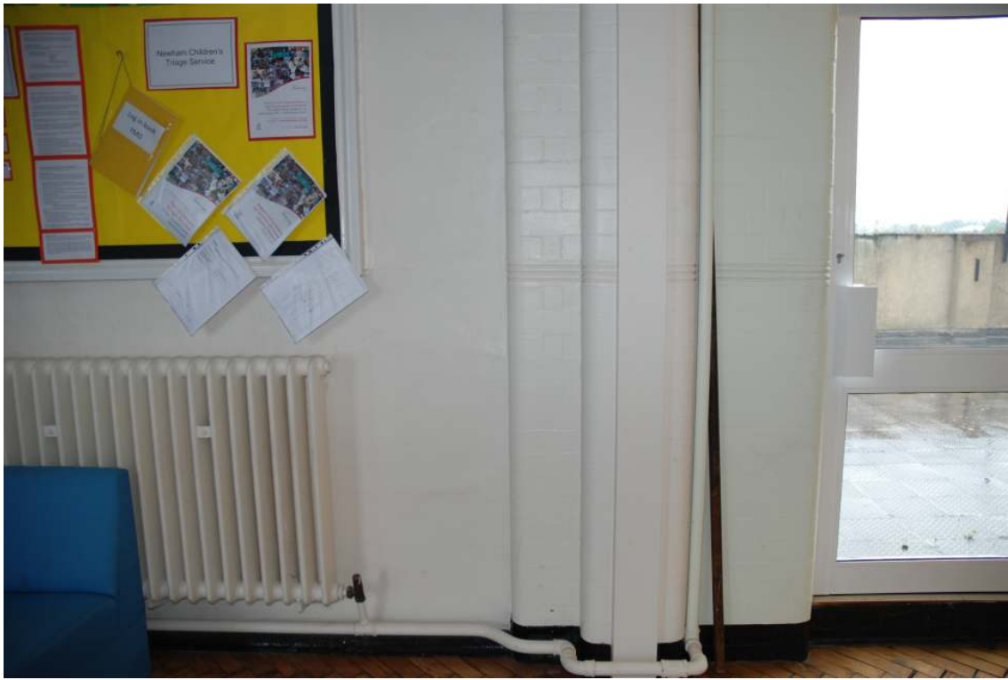
Fig.35: The join between the original and new parts of the northern wall of room 3 – the original (eastern) part has a string course and visible brick coursing; the later (western) part lacks these
