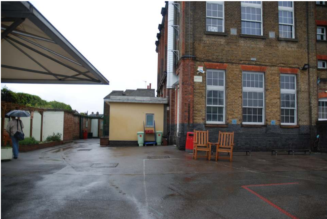
Fig.60: The area of the proposed extension between rooms 15 and 16, looking north
