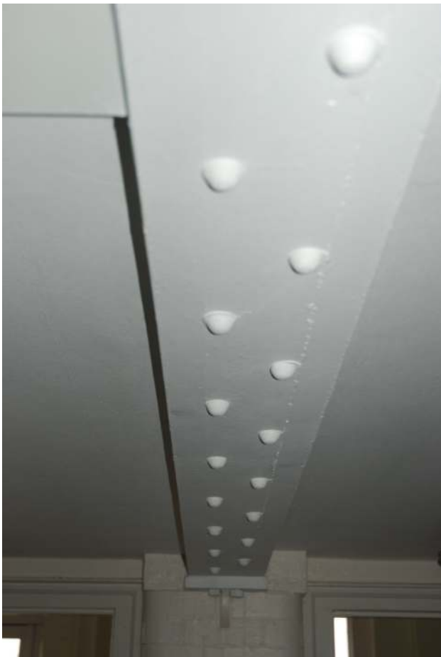
Fig.32: One of the riveted metal beams in rooms 2 and 5
