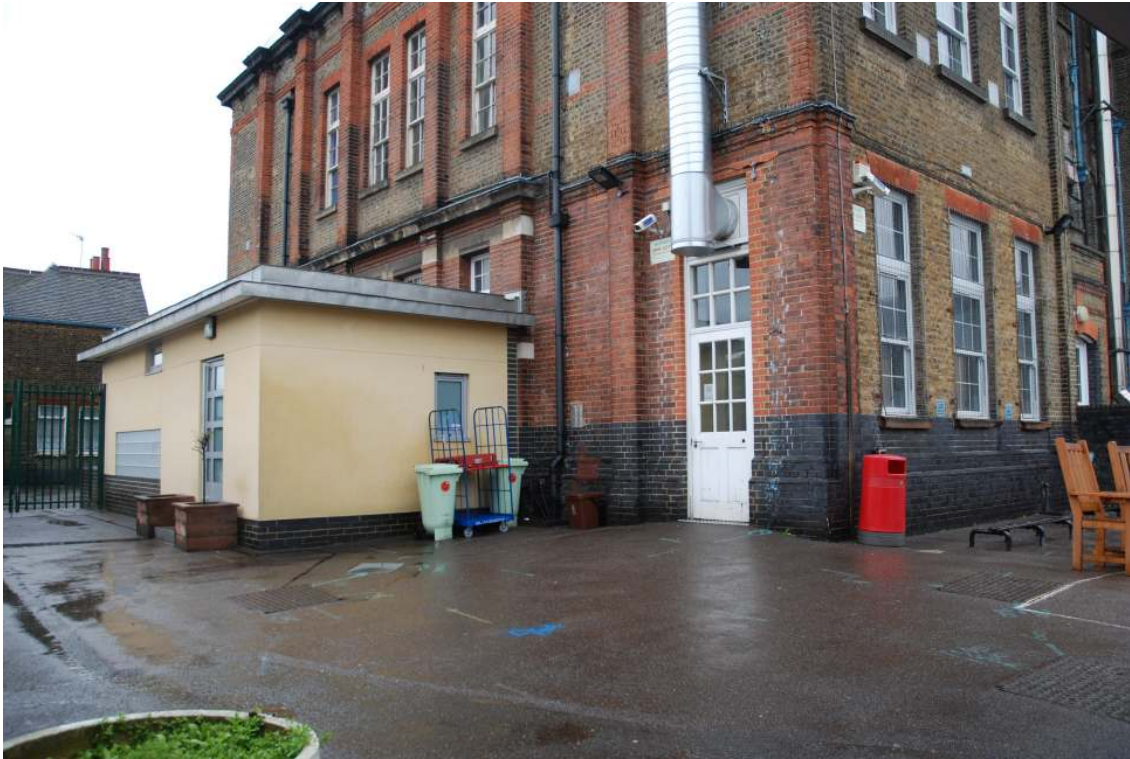
Fig.59: The area of the proposed extension between rooms 15 and 16, looking north-east, and showing the original school building and later single-storey extension
