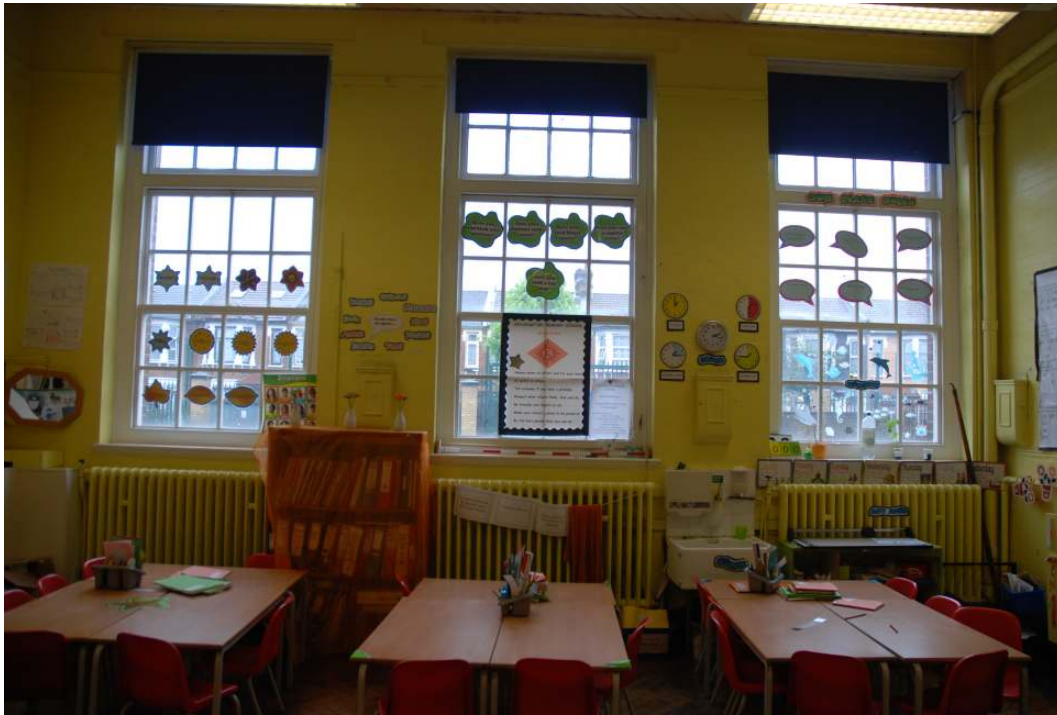
Fig.71: The northern wall of room 13, showing the original windows and ventilation boxes (between windows and on adjacent eastern wall)
