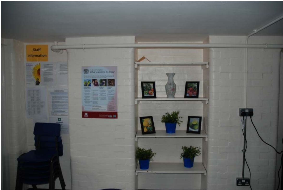
Fig.30: The chimney supports on the eastern side of room 2, for fireplace in overlying mezzanine level
