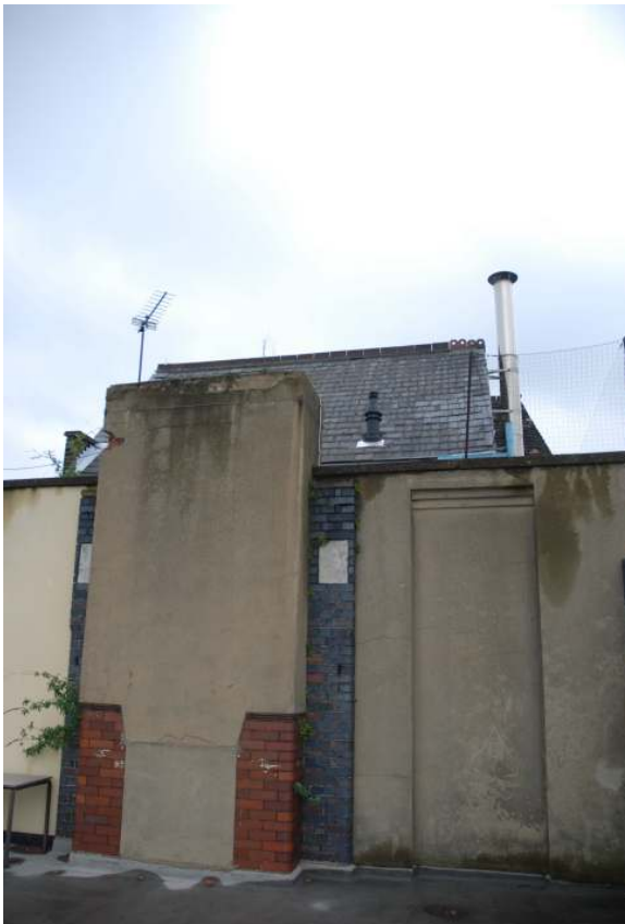
Fig.33: The chimney on the western side of the building
