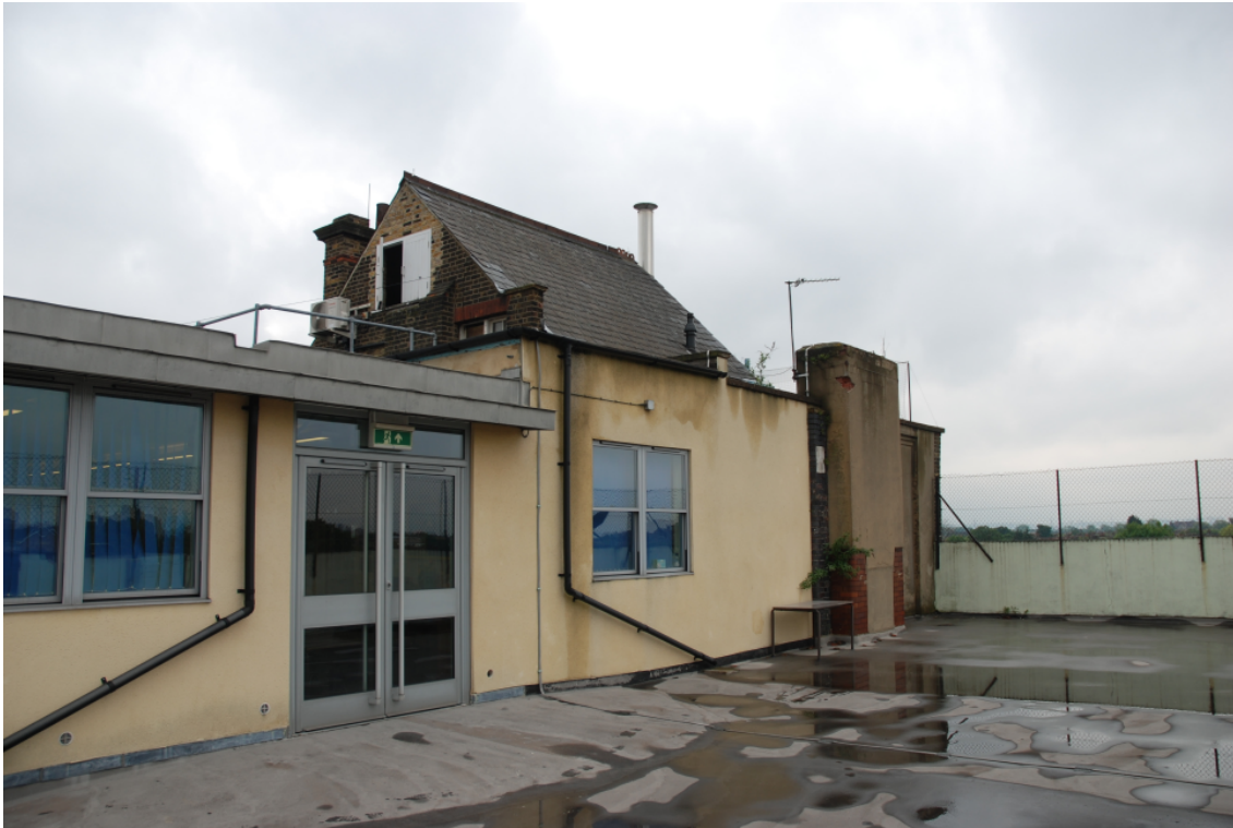
Fig.41: The western end of the second-floor buildings, and adjacent roof terrace
