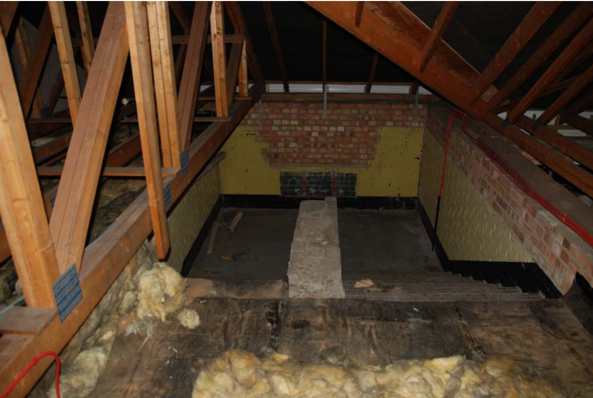
Fig.27: The stairs in the roof-space, western end
