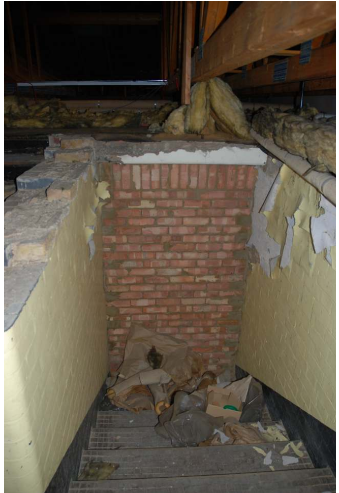
Fig.29: The blocked-up doorway between the first-floor mezzanine and roof-space, western end
