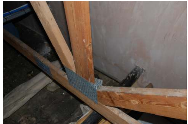
Fig.26: Close-up of a junction of the roof-timbers
