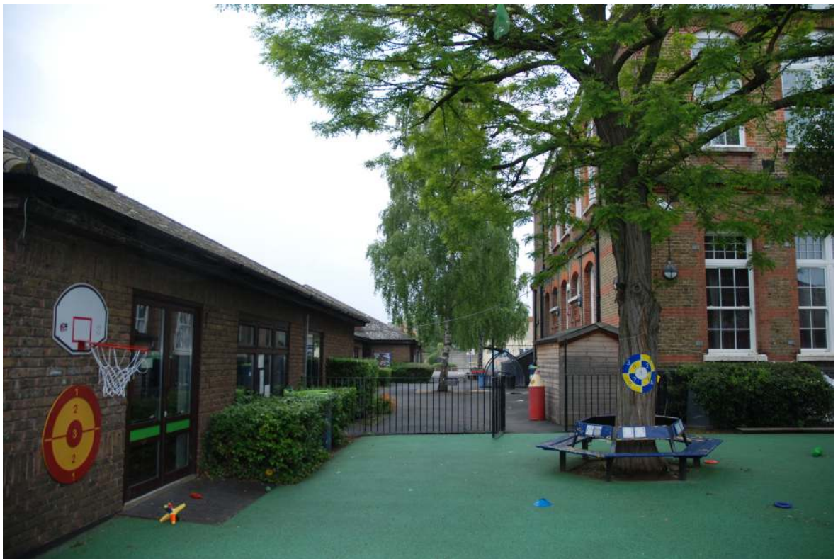
Fig.34: The area of the proposed extension, looking north
