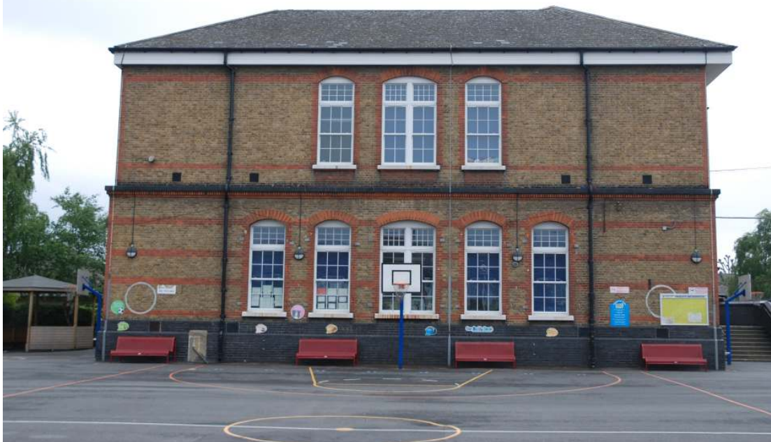
Fig.41: The eastern frontage, showing the lines of coloured brickwork and moulded string course
