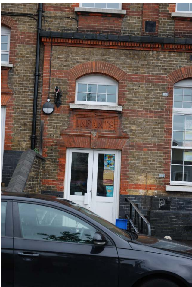
Fig.41: The eastern frontage, showing the lines of coloured brickwork and moulded string course
