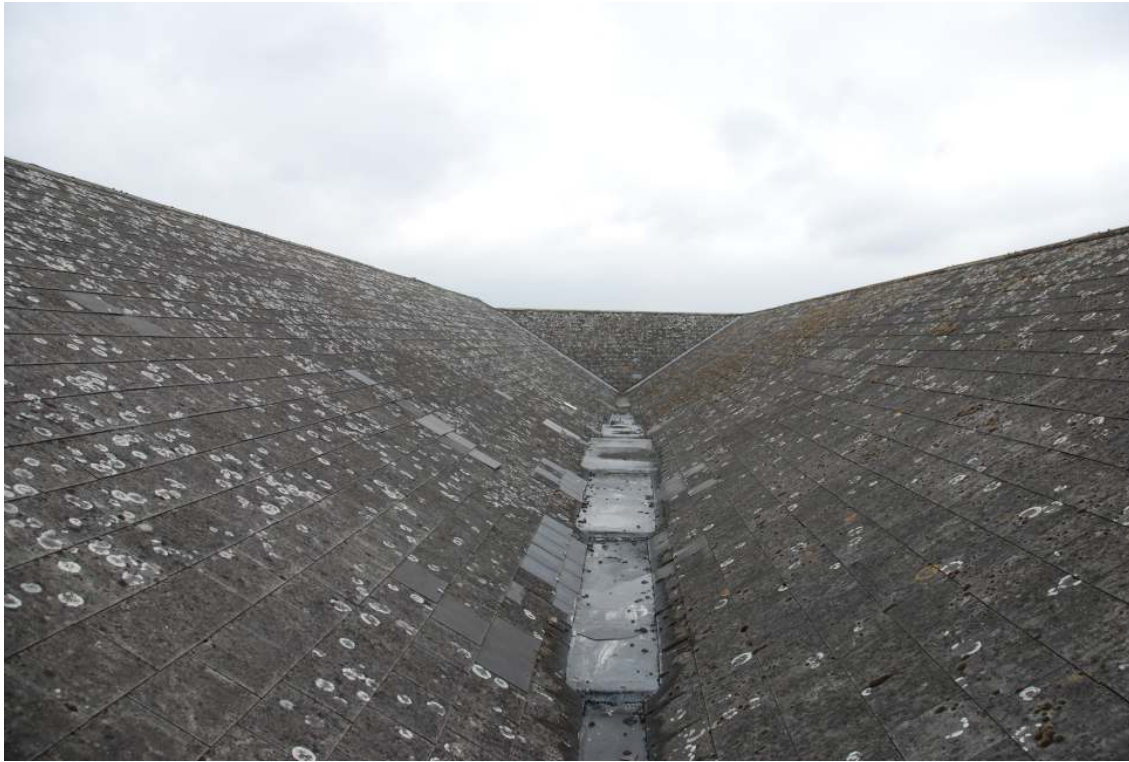
Fig.21: The roof today
