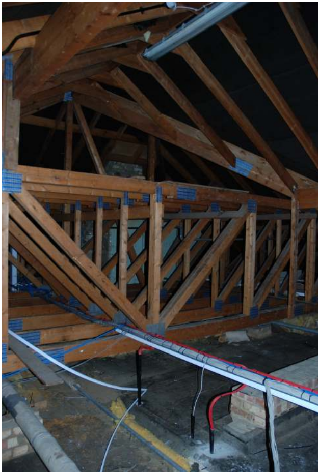
Fig.25: The roof-space today, showing the concrete floor
