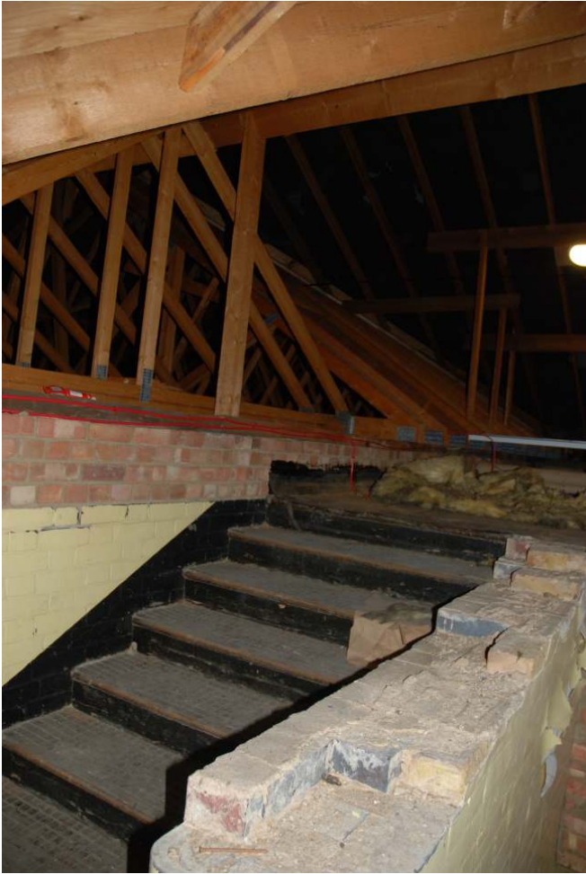
Fig.28: Close-up of the stairs in the roof-space, western end
