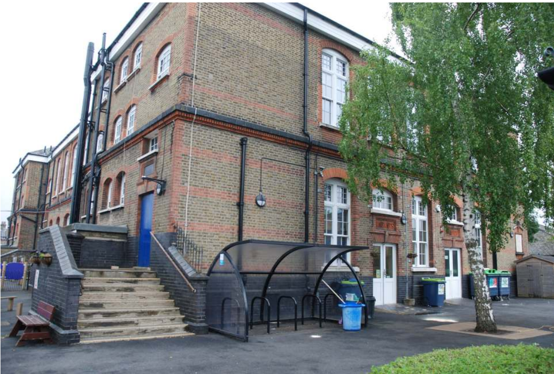
Fig.37: The original western frontage of the main school building, looking south-east
