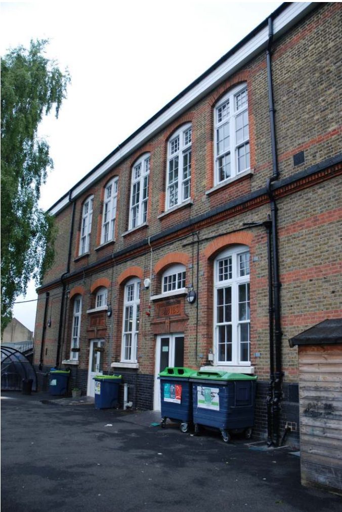
Fig.36: The original western frontage of the main school building, looking north-east
