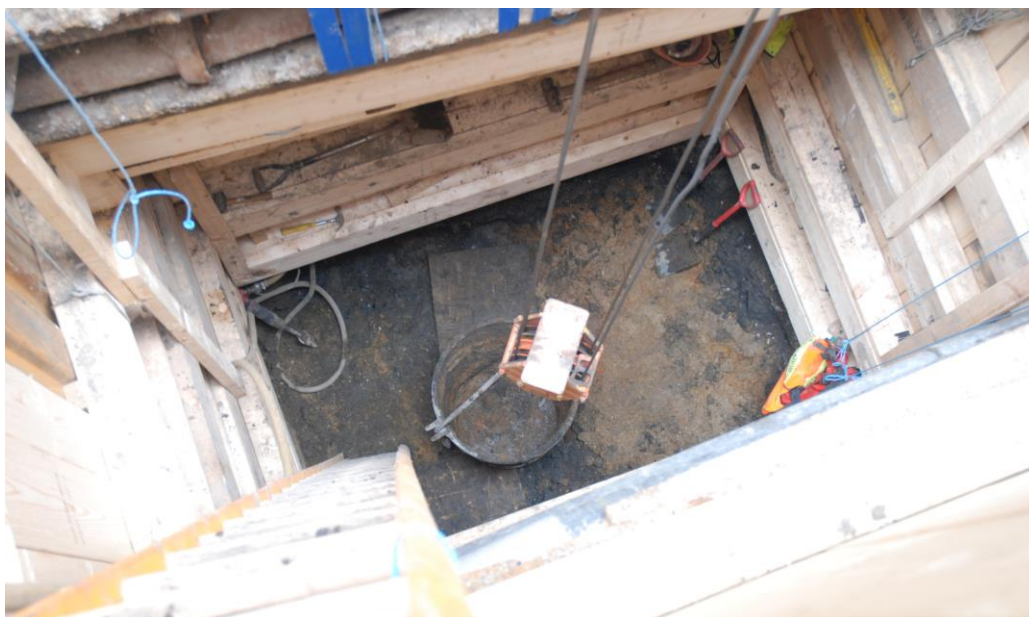
Fig.14: Pit 3 at c5.5m below ground level showing the dark-grey silt overlying natural gravels and sands
