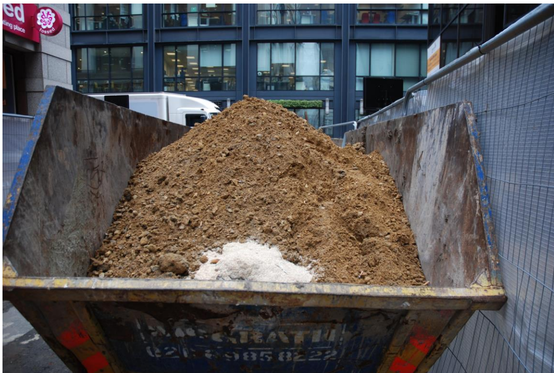
Fig.16: Natural gravels as excavated from the pit.
