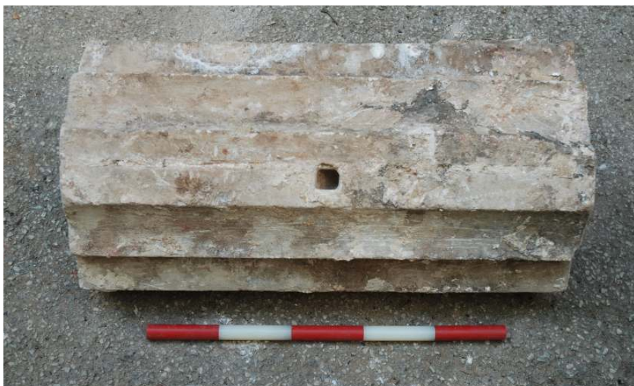
Fig.46: Block H showing internal face of possible window mullion fragment with hole for fitting, and groove just visible above this (50cm scale)
