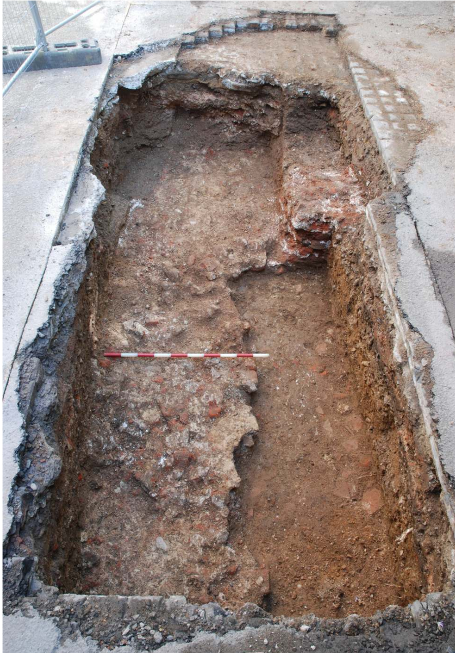
Fig.18: Foundations [5], left, and [7], right, in Trench 1 facing N. (1m scale)
