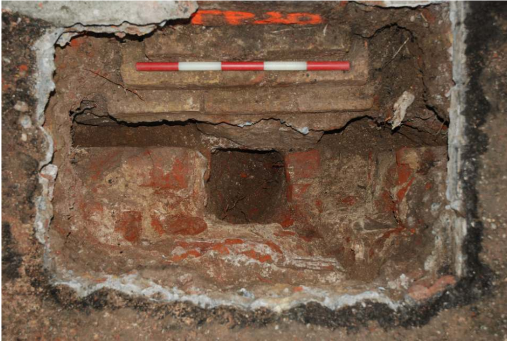
Fig.8: Trial pit 20 showing existing footings to north wall of 94 Cheyne Walk and continuation of E-W aligned wall from Trial pit 8 in bottom of frame. (50cm scale)
