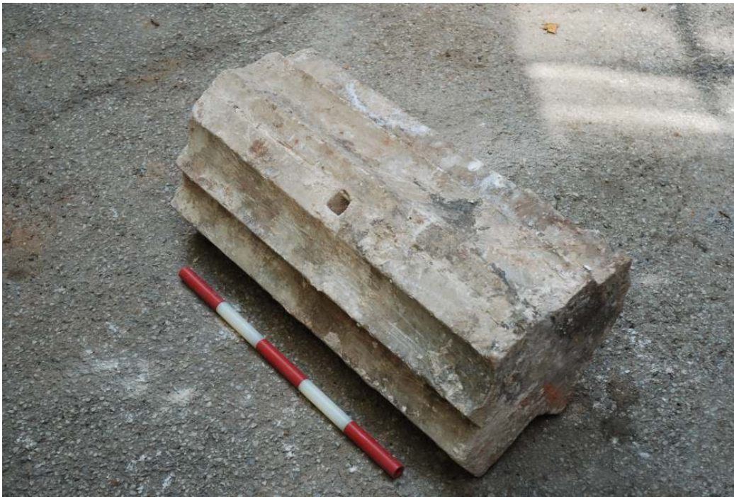
Fig.24: Block H having been removed from foundations. It shows the opposite side to that visible in fig.23 above. (50cm scale)
