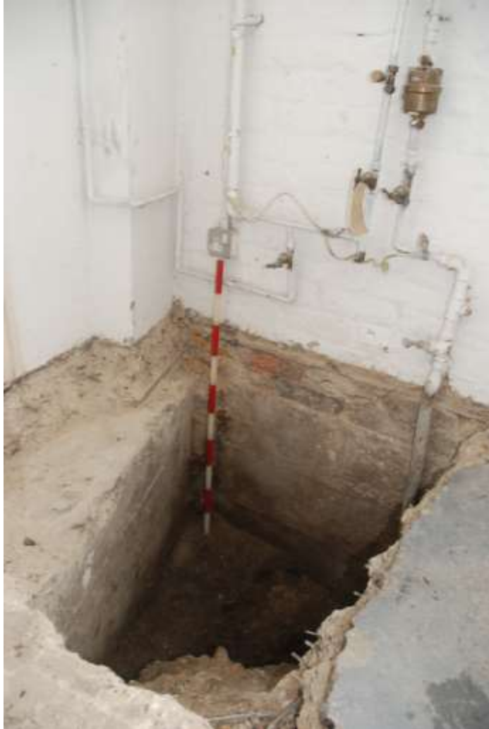
Fig.9: Photo of the trial pit, looking south-east. The concrete foundations of both the southern and eastern walls can be seen
