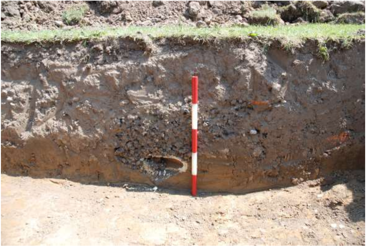
Fig.21: Photo of the section around the land drain, trench 2
