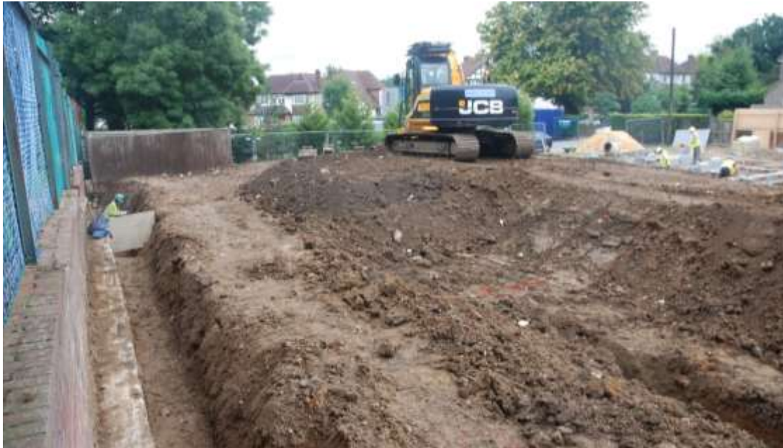
Fig.16: General shot of strip footings along northern boundary facing ESE
