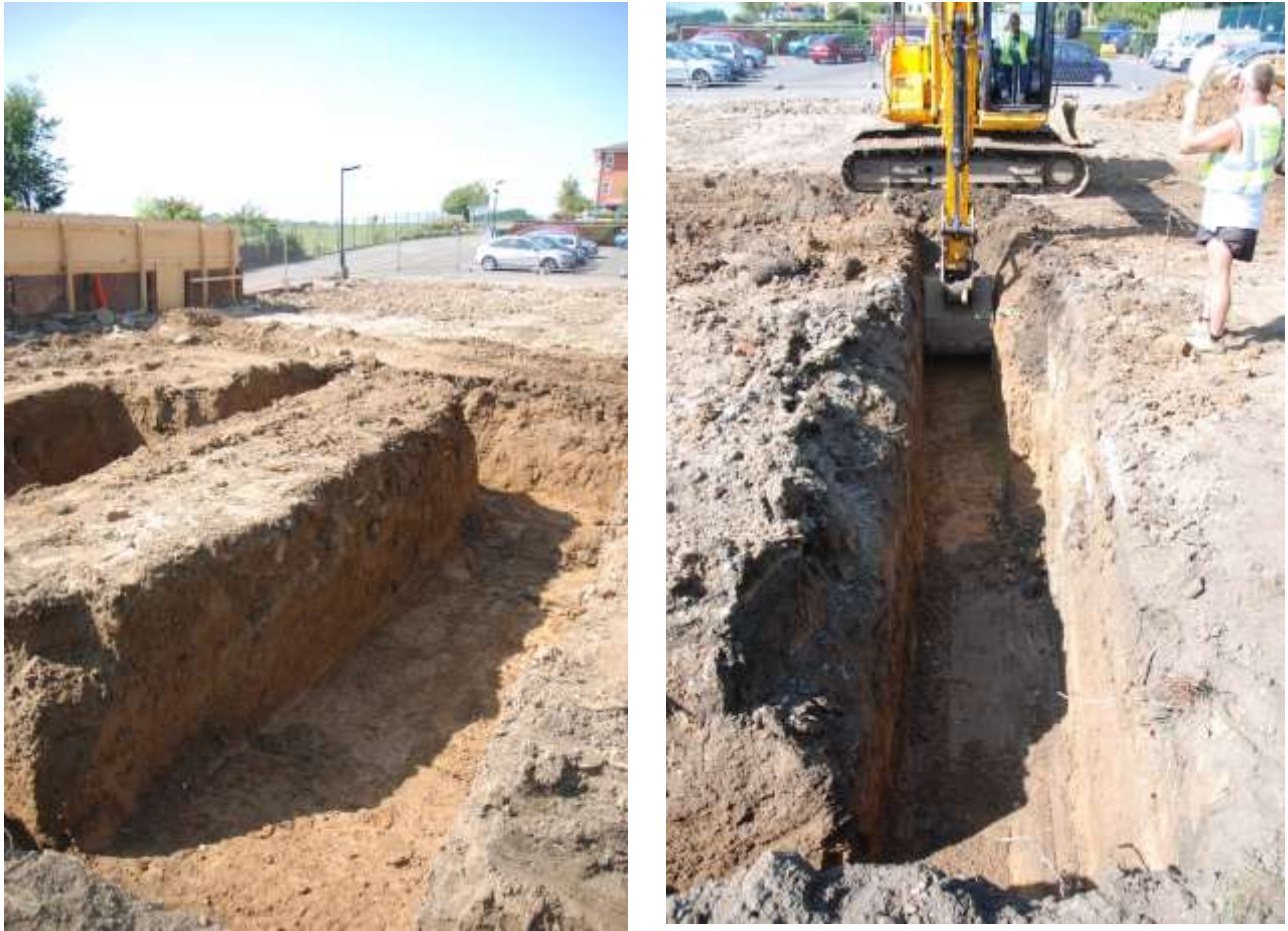
Fig.9: General photos of the foundations of the main building
