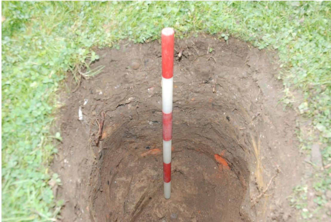
Fig.26: Photo of the southern section of soakage pit 2. 0.6m scale.
