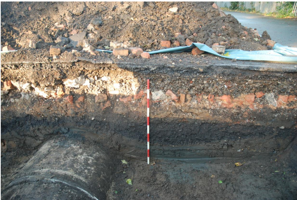
Fig.25: Photo of section in trench 3, the concrete pipe assumed to contain the culverted stream to left of frame
