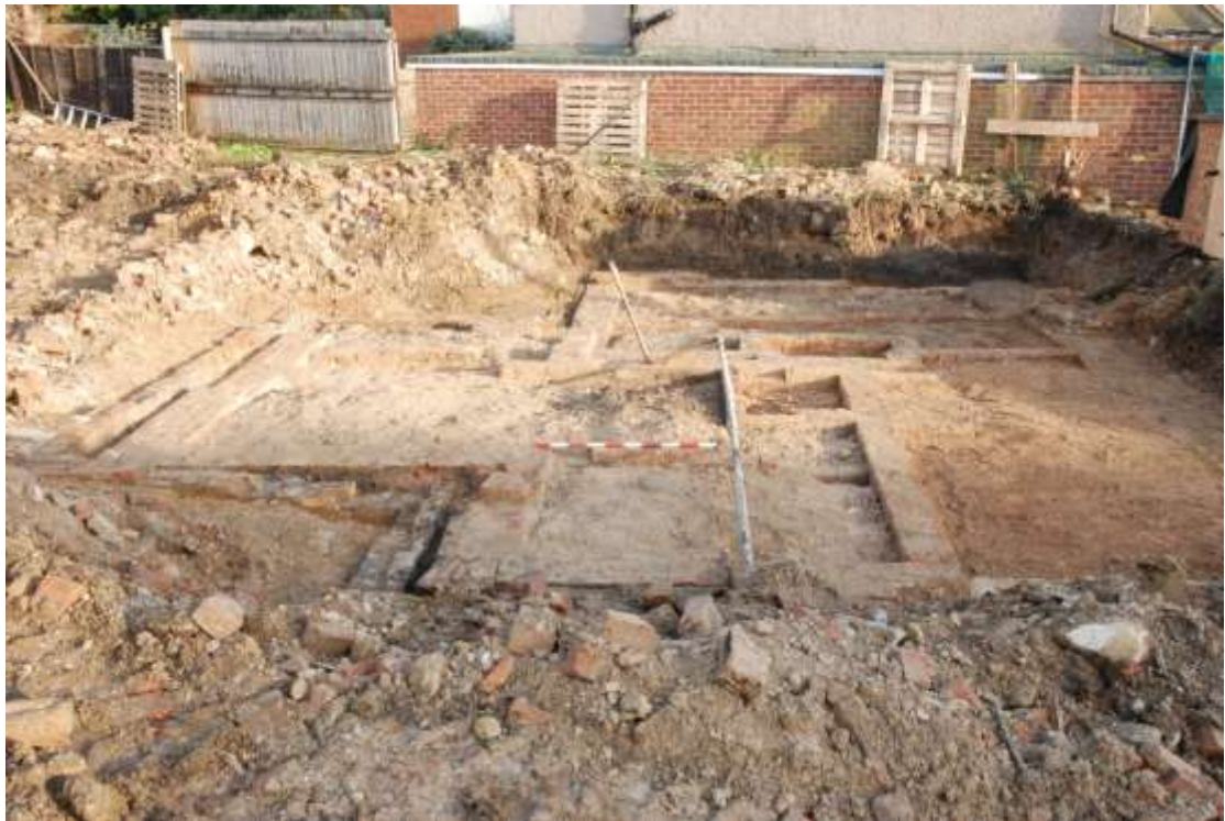
Fig.16: 'Lodge' footings facing E, (1m scale)
