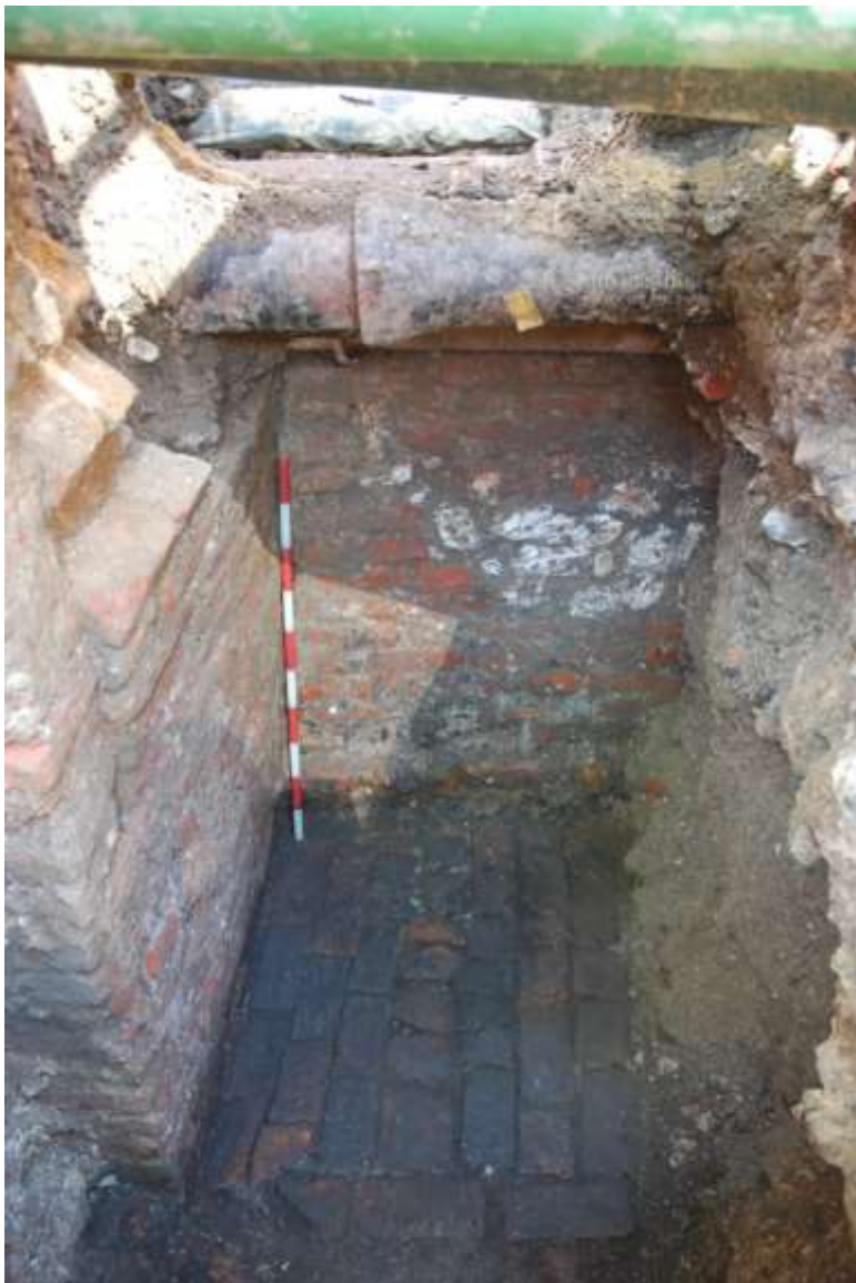
Fig.6: The brick-built chamber, [6], facing SW. Note the springing for an arch to the left of the frame. The rear wall, against which the 1m scale rests probably represents the furthest extent of the chamber. The corner of the wall in the left foreground was probably on a line with the early street frontage
