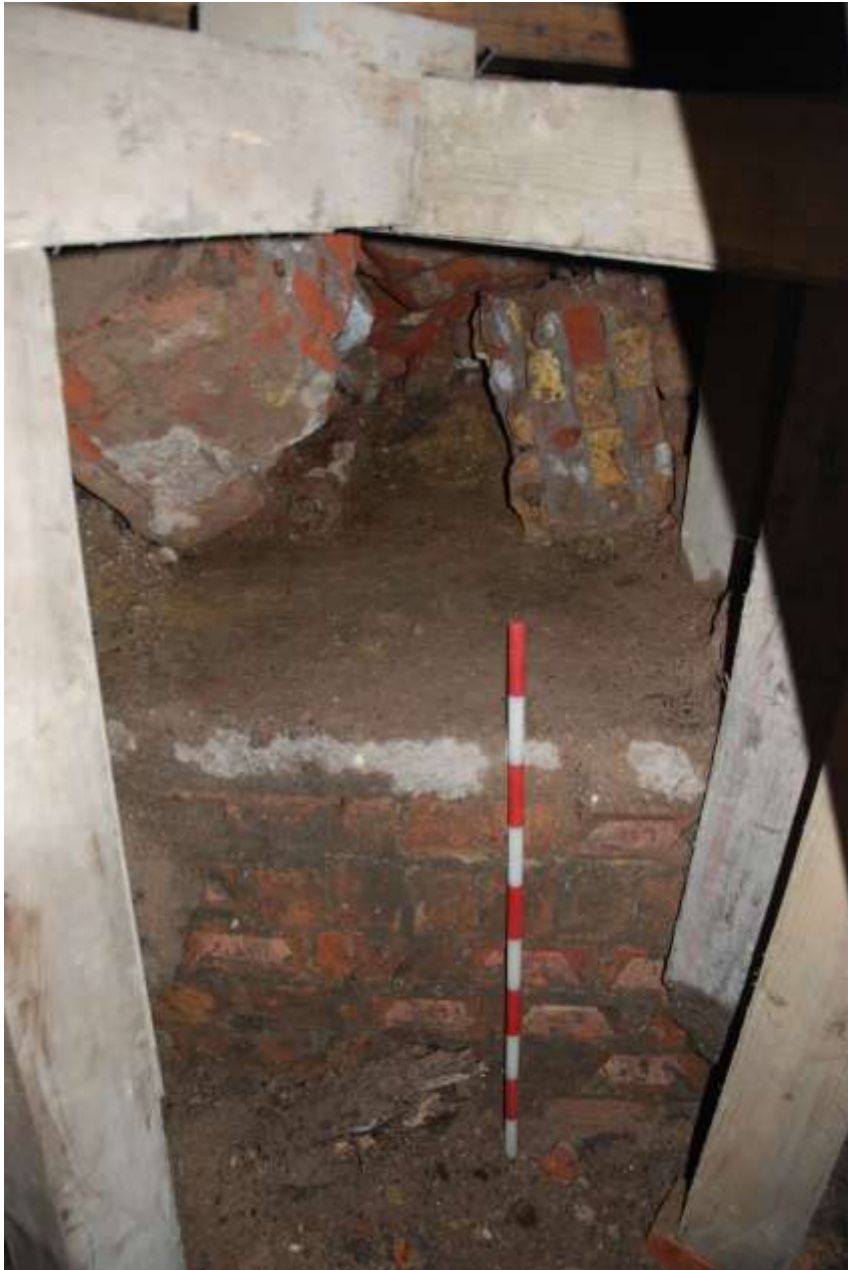
Fig.22: View of the roof of the pedestrian subway in the SW corner of Pit 3, (1m scale). Note the large blocks of brickwork used as backfill, probably derived from earlier buildings that once stood on site
