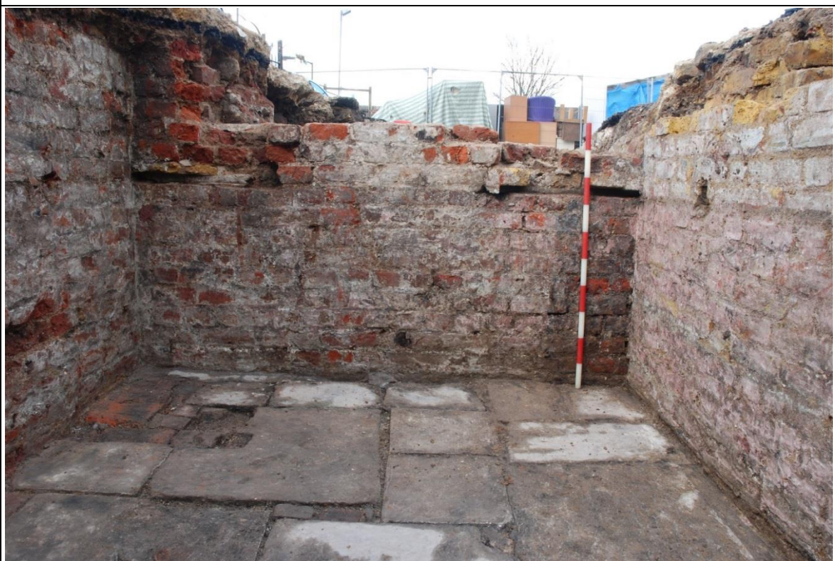
Plate 11: The north wall of the cellar [12] showing later shelf rebates
