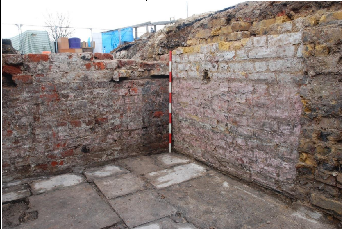
Plate 10: NE corner of cellar with later wall [8] to right
