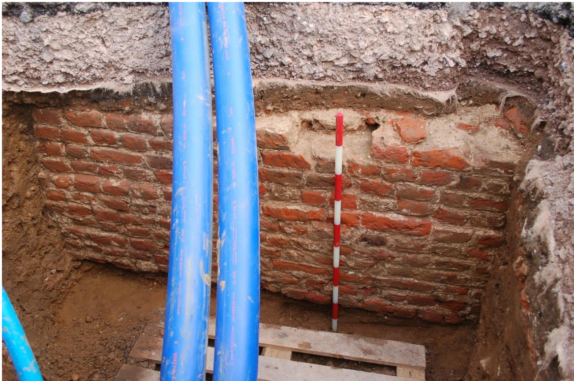
Fig.4: Wall in Trench 1 of the 2010 watching brief, facing SE. This wall would potentially continue through Zone 1 of the proposed glasshouse
