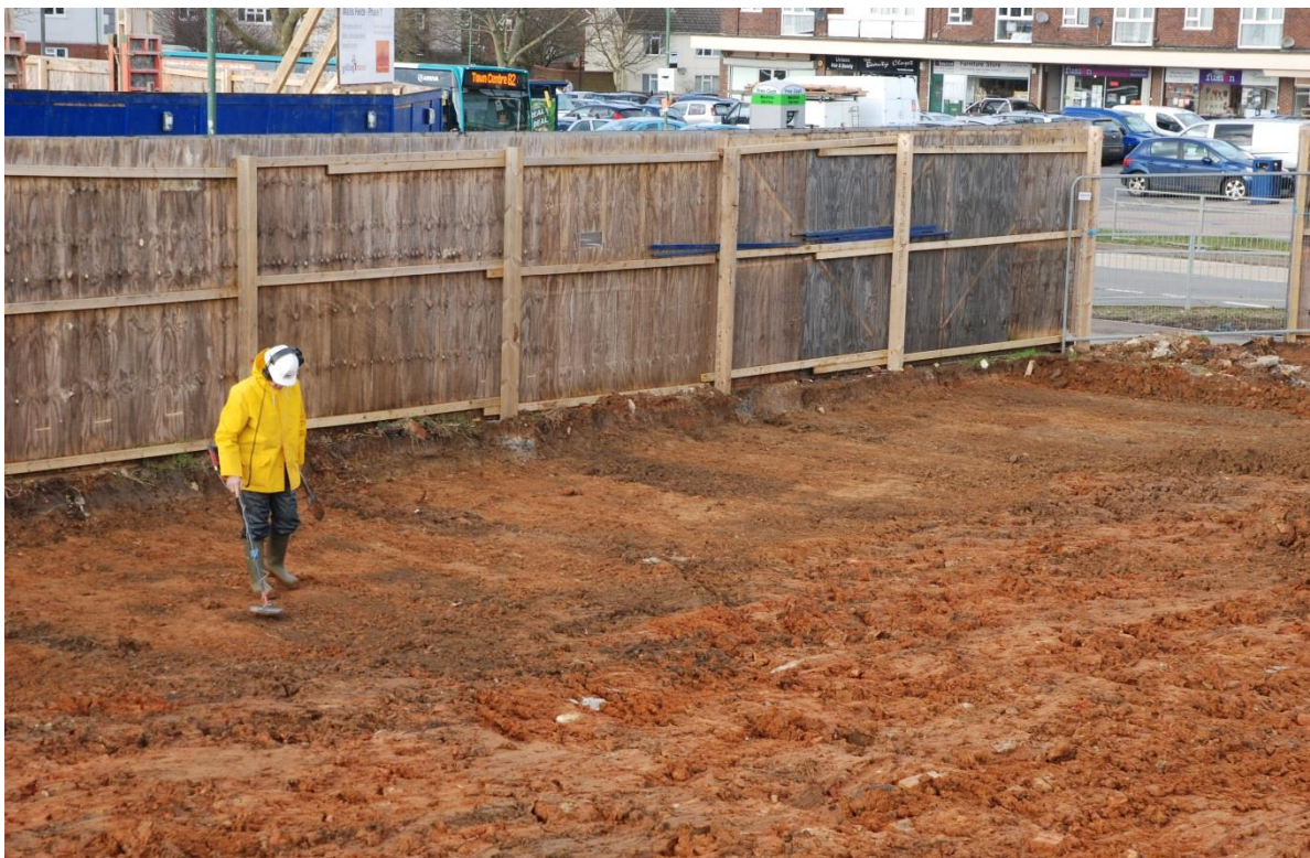
Fig. 14: The northern part of Area 1, looking northwest towards the junction of Longshaw Road and Wallis Avenue. Note the distinction between the disturbed area in the foreground (from the demolished buildings), and the former front gardens adjoining the site boundary where exposed natural is cut by a series of darker lines representing infilled service trenches
