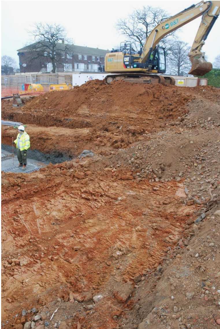
Fig. 21: View of Area 3 during machine stripping, looking north towards Wallis Avenue.
