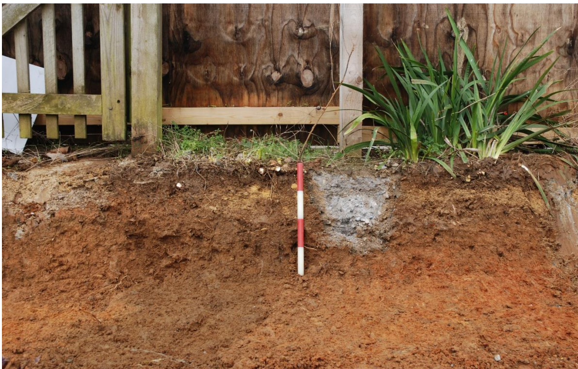
Fig. 16: Exposed section on the western boundary of the site, c 3m north of the southwest corner of Area 1 (0.4m scale). A shallow soil profile ( \leq 100\text{mm} ) overlies lighter yellow-brown made ground and thence either clean natural or – immediately left of the scale – a slightly darker band some 600mm wide representing an infilled service trench
