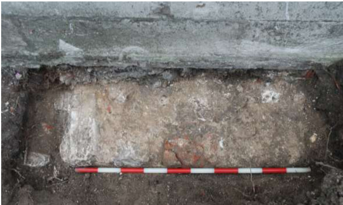
Fig.28: Wall 2 facing south. The extant northern wall of the church is at the top of frame. The stone at the left end of the scale showed signs of having once been part of a window, (1m scale)
