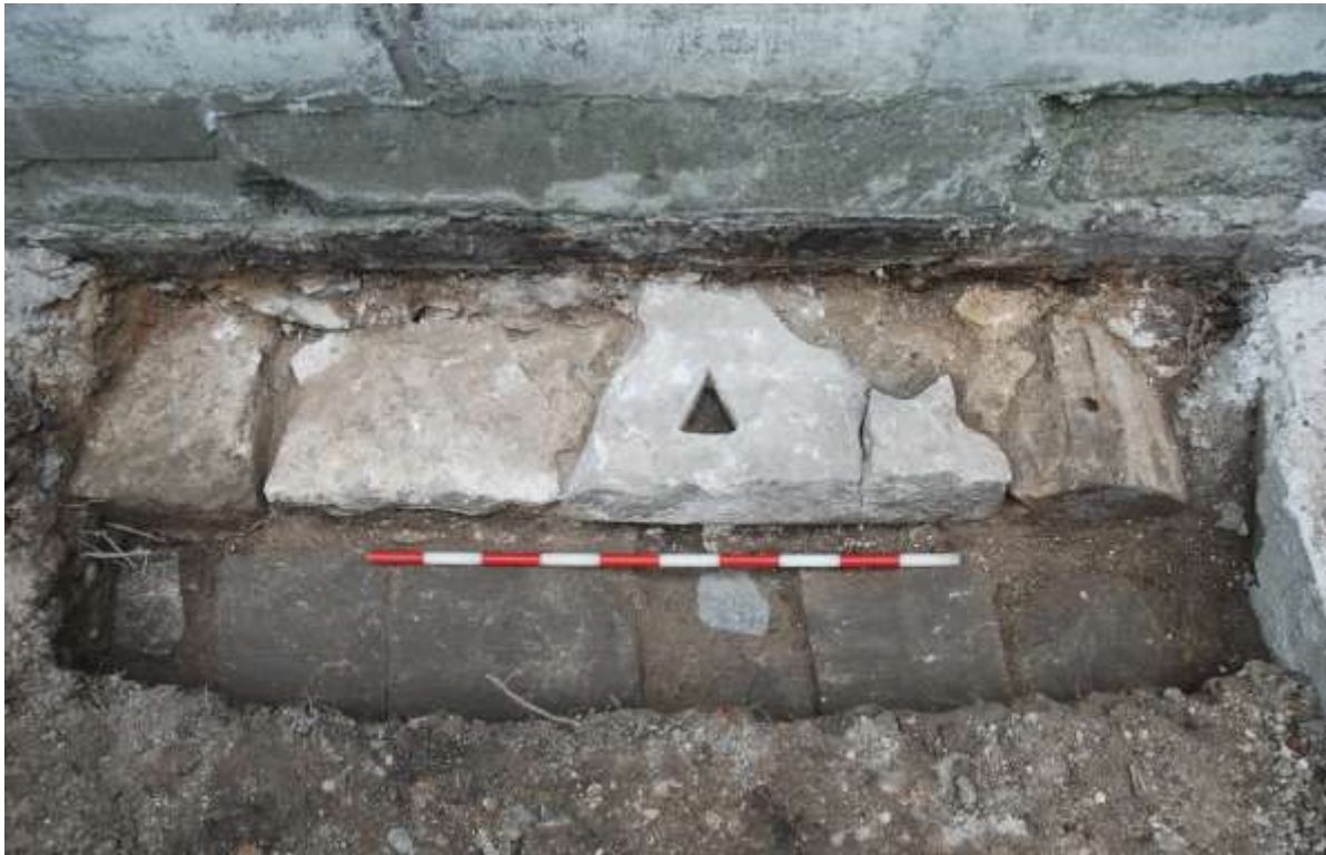
Fig.30: Wall 3, facing south, with at least two re-used architectural fragments including part of a window mullion at the far right end, and a larger piece of tracery above the 1m scale. Note the stone slabs below the scale, apparently representing a former paved surface
