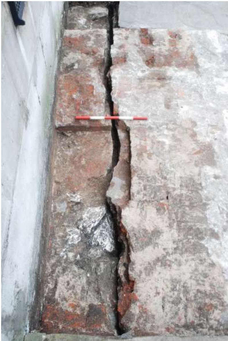
Fig.22: The eastern end of Wall 1 as exposed, showing the mixture of materials used in its construction. Vault v/003 is to the right of frame, built up against and slightly over the wall, (0.5m scale)
