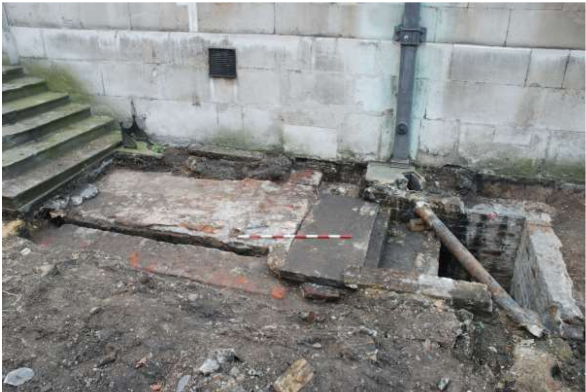
Fig.14: The two vaults, looking towards the north wall of the Church: the brick-roofed v/003 on the left of the frame and the partly-open v/004 to the right (1m scale)
