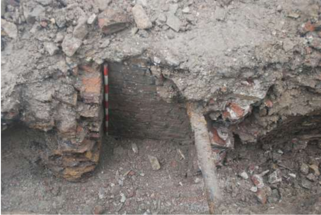
Fig.24: Former drainage box at the northern end of Trench 8, facing ESE, (1m scale)
