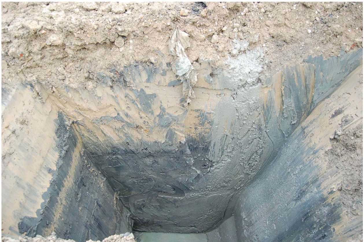
Fig 5 View of Trial Pit 1 looking south
