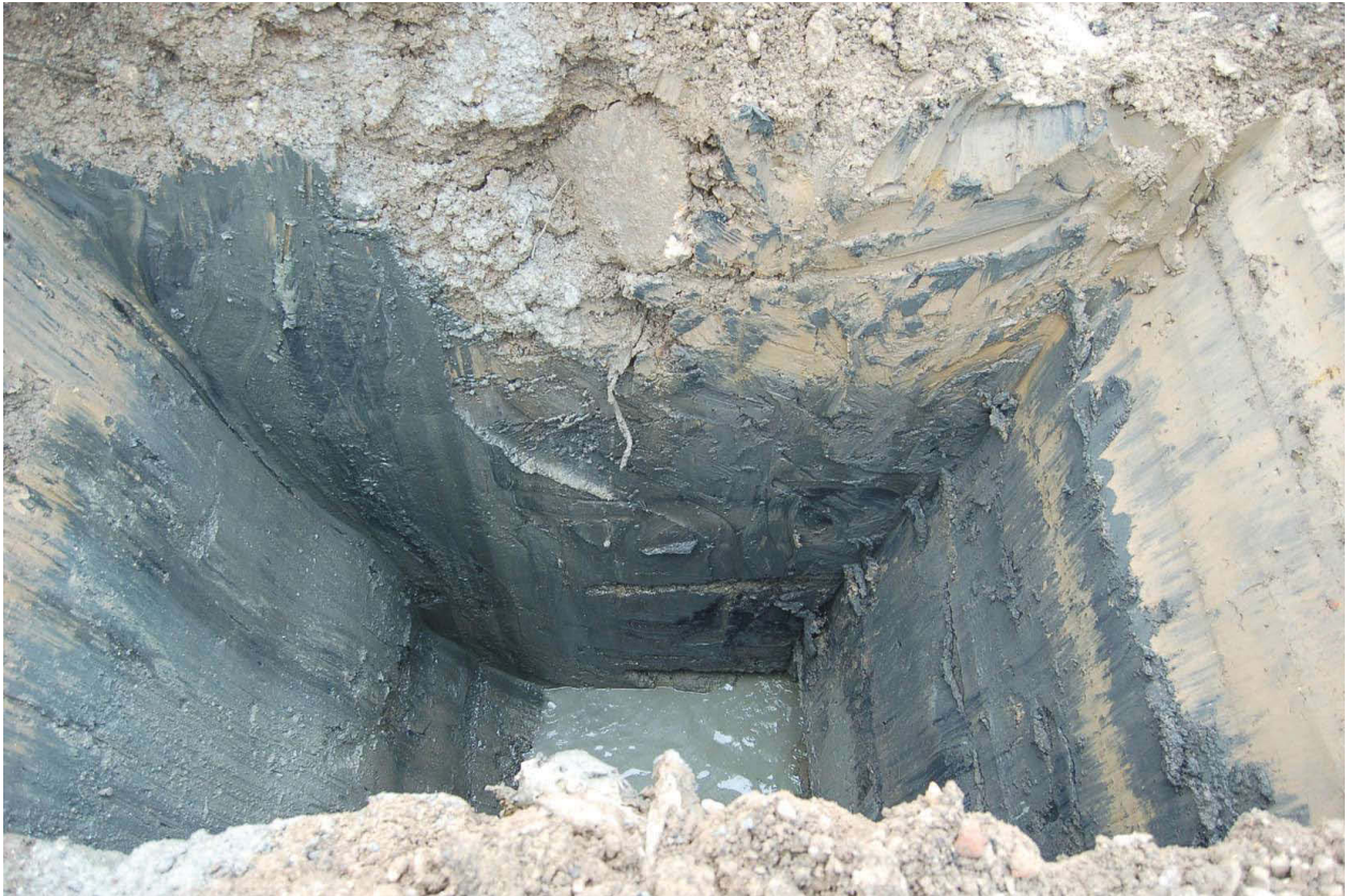
Fig 4 View of Trial Pit 1 looking north
