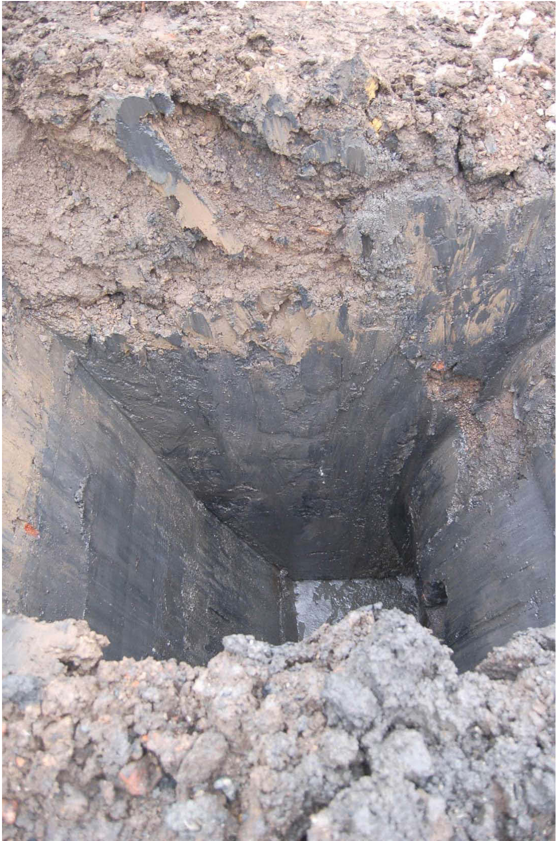
Fig 8 View of Trial Pit 2 looking south
