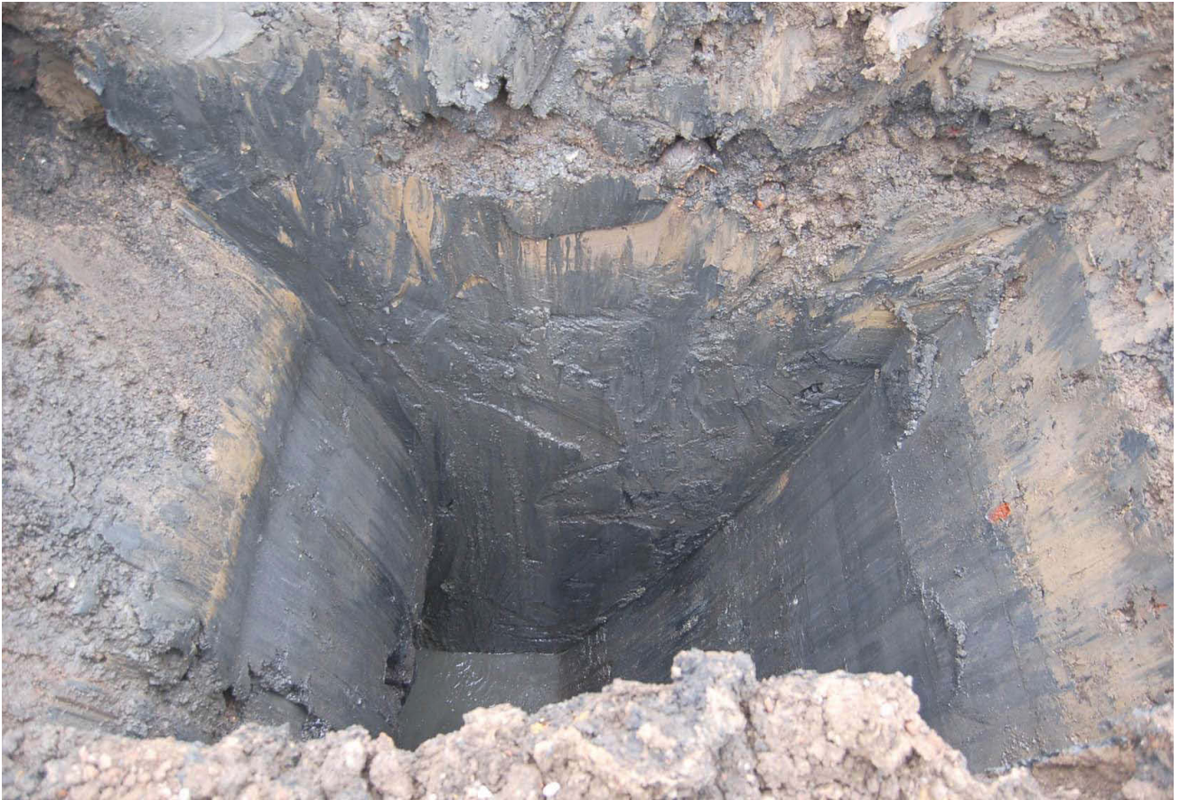
Fig 7 View of Trial Pit 2 looking north
