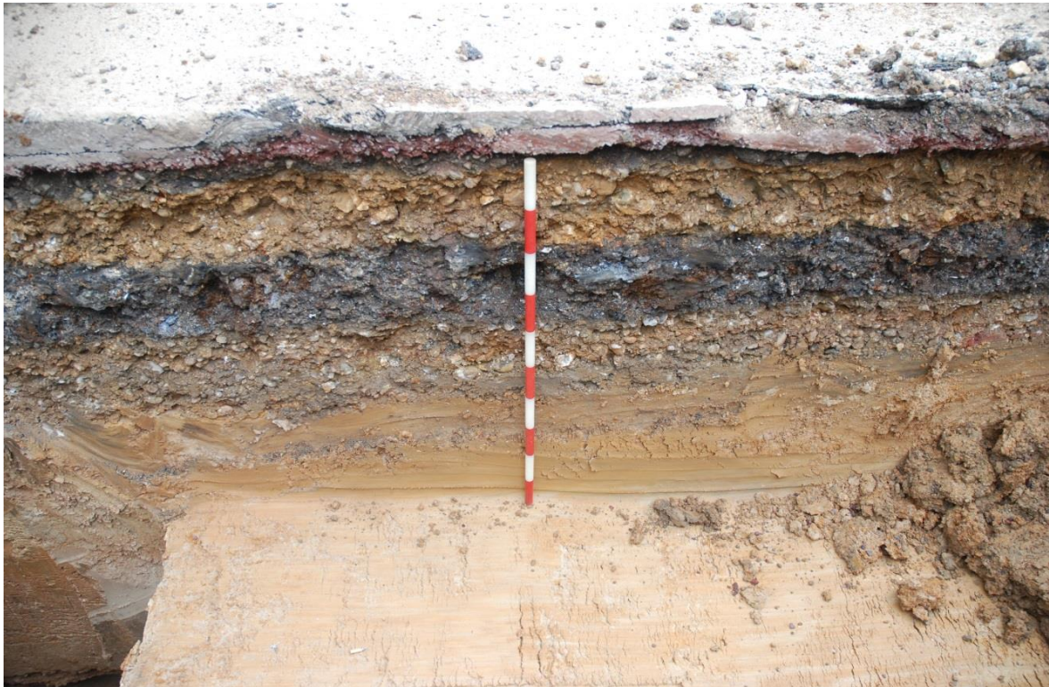
Fig.9: Trench 2, section facing NW showing road makeup and natural brickearth beneath (1m scale)
