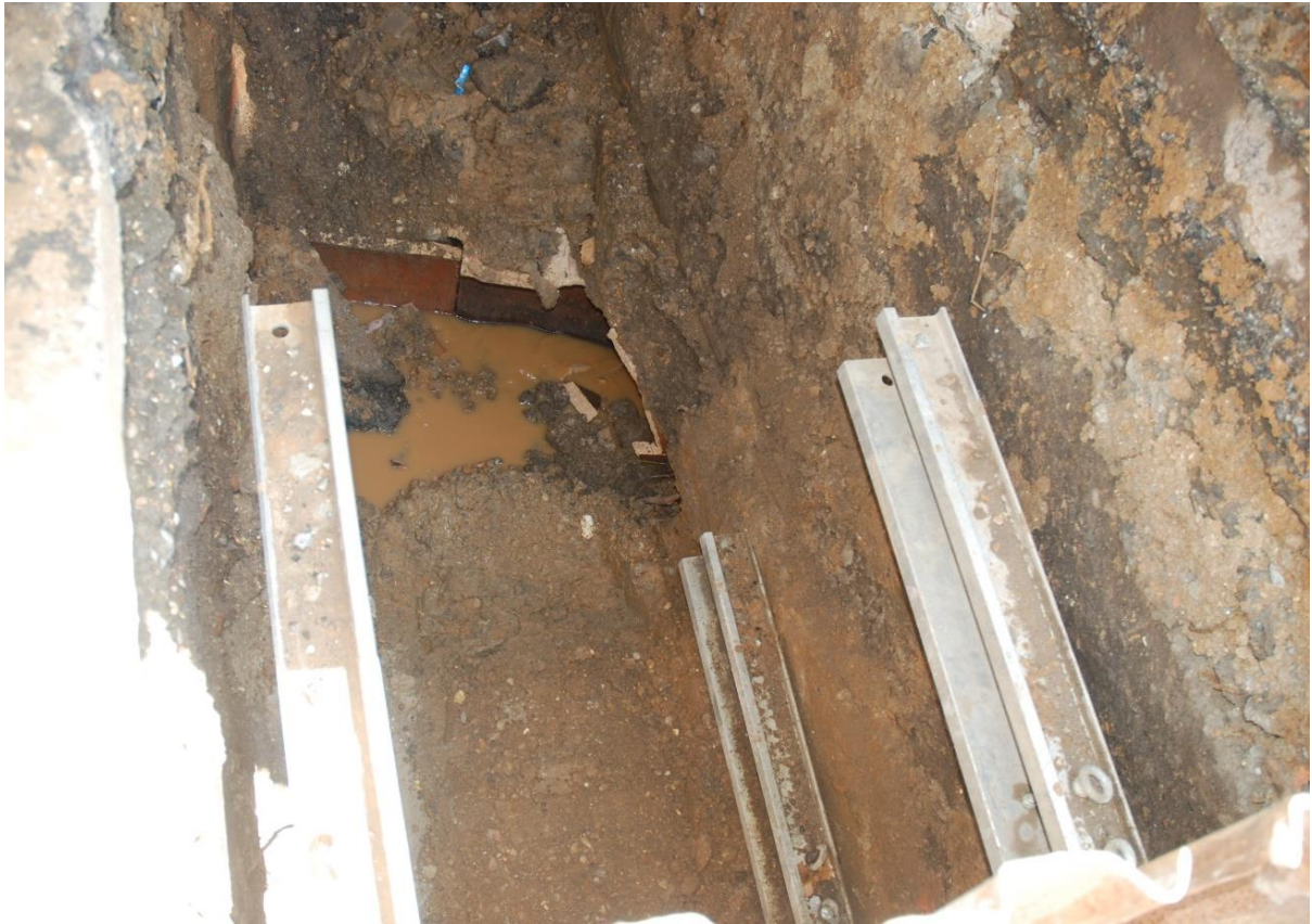
Fig.13: Trench 3, showing the modern fill of the trench
