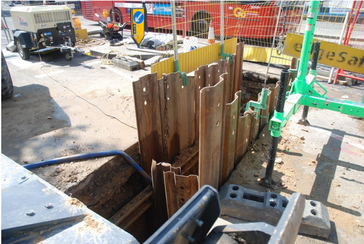
Fig.12: Trench 3, showing safety box and extension of the trench, facing W
