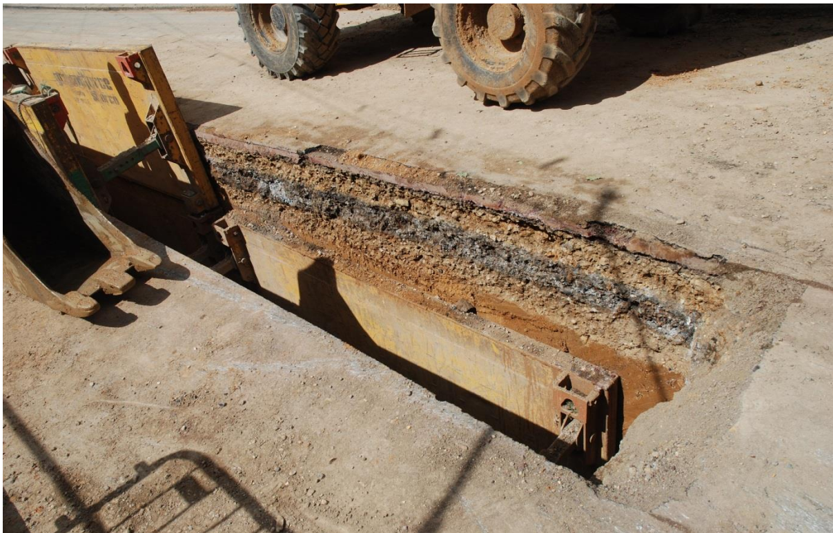
Fig.15: Trench 4, section, facing NW
