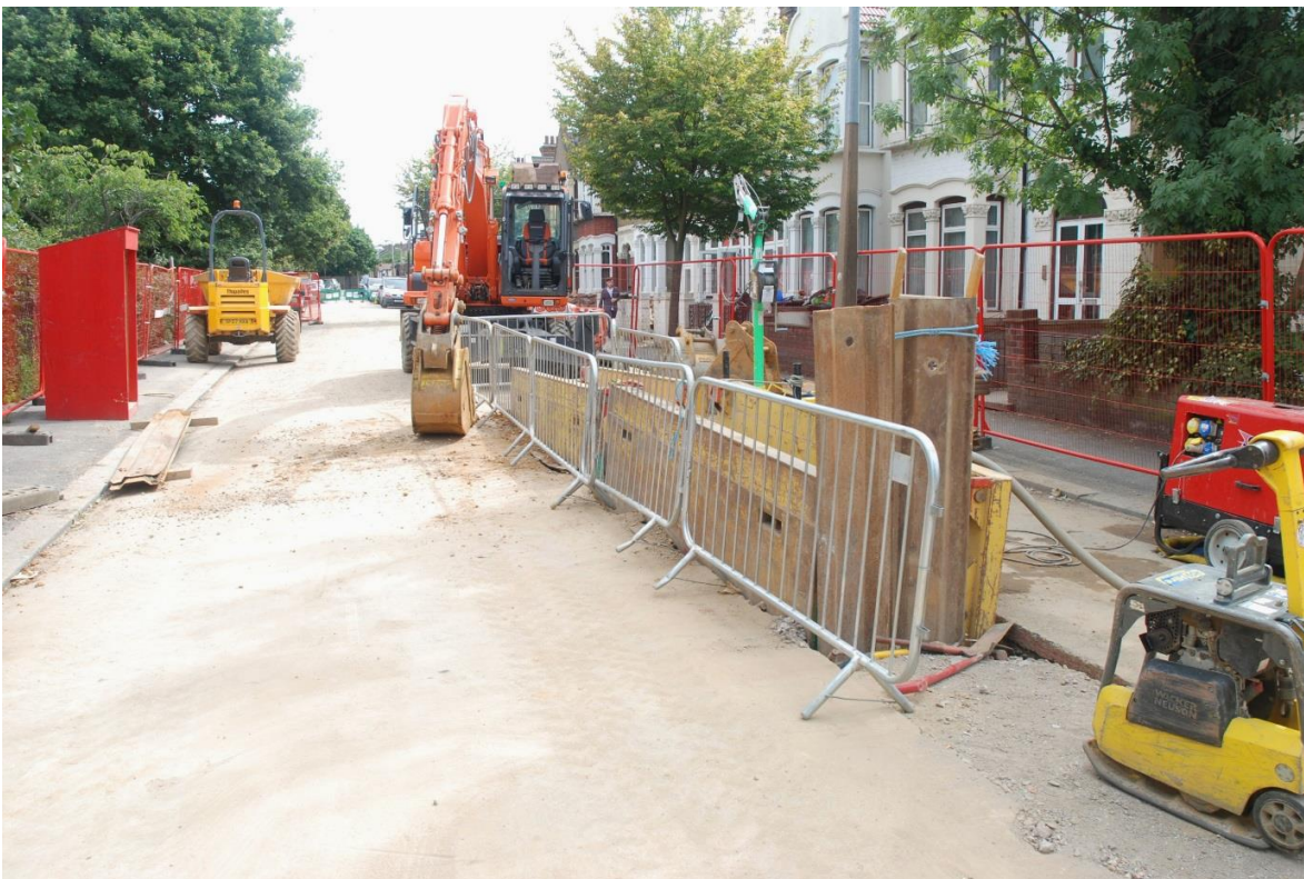
Fig.11: Trench 2, safety box
