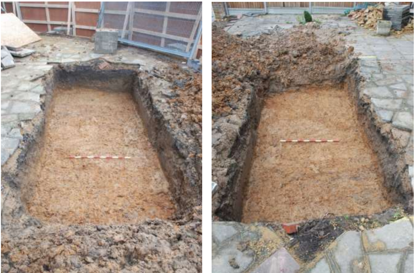
Fig.6: Trench 1 in the front garden of the property facing SSE, (left), and NNW, (right). 1m scale
