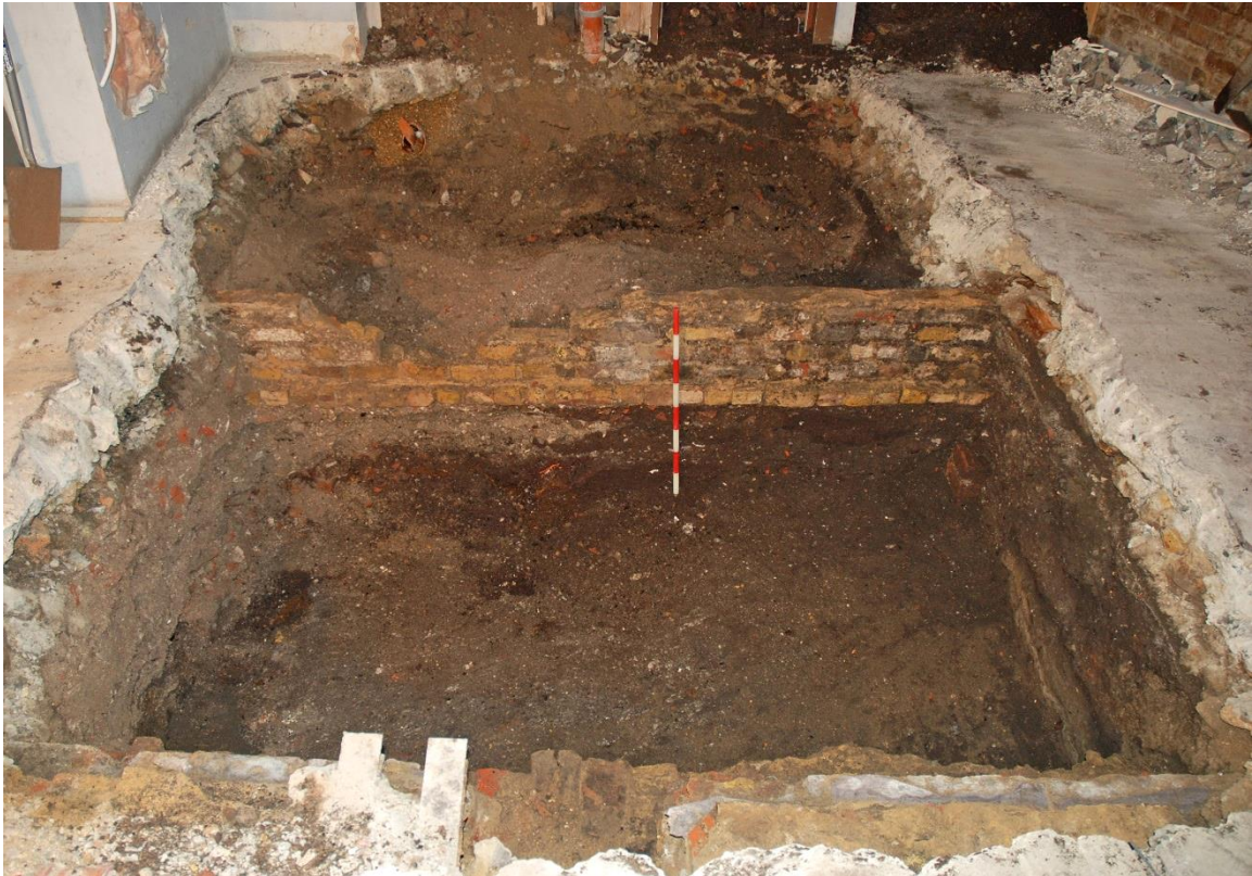
Fig.19: View of the trench after initial excavation and looking south, the 1m scale resting against the central cross-wall (4) and the top of wall base (2) in the foreground
