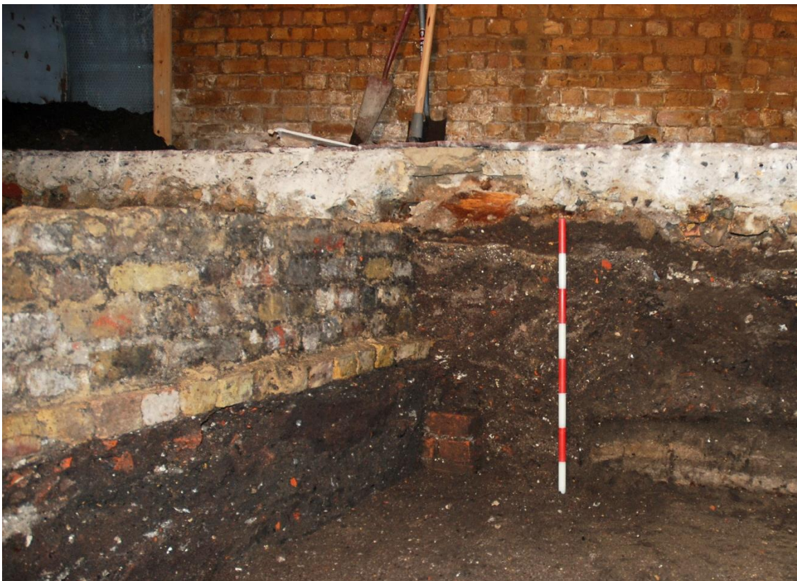
Fig.20: Detail of the western end /north side of wall base (4), cut into and built over the made ground (8)
