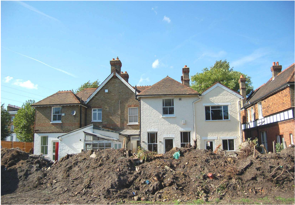
Fig 33 View of rear elevations of numbers 393 and 391
