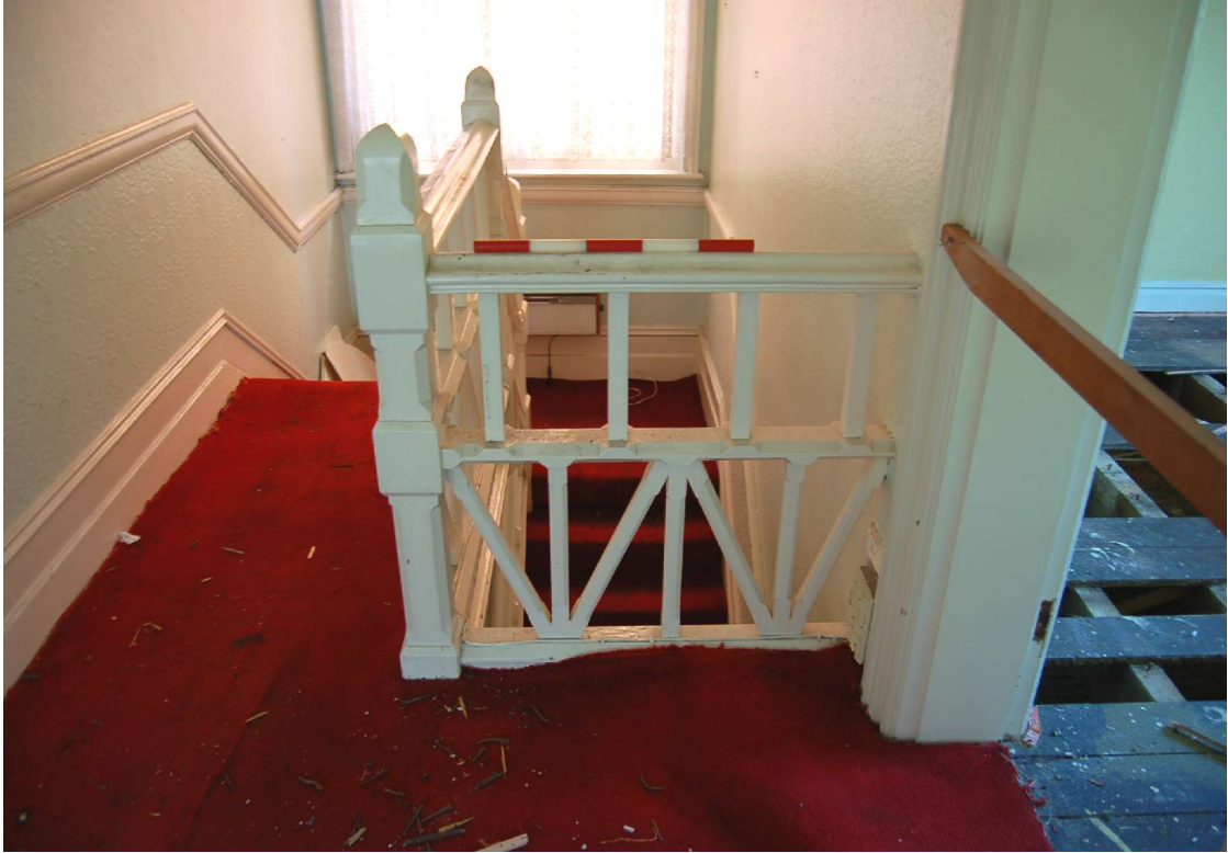
Fig 27 View of staircase design in number 389 taken from first floor
