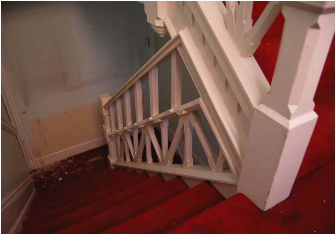
Fig 28 View of staircase design in number 389 looking toward ground floor
