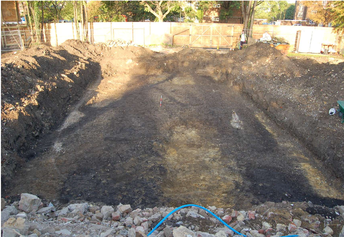
Fig 15 Pre-excavation view of features in the extended area of Trench 2
