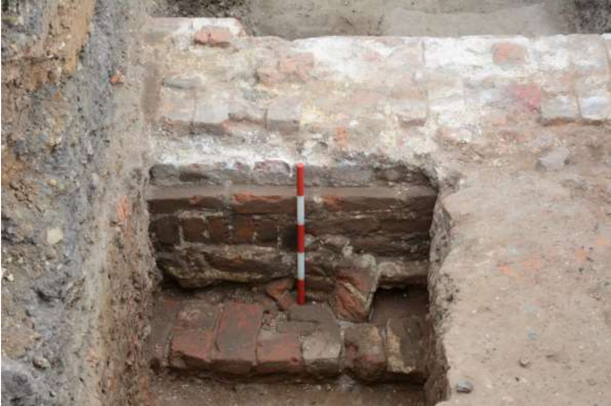
Fig.19: Detail of the rear (north) face and base of the retaining wall (7), after partial excavation of the retained deposit (4)
