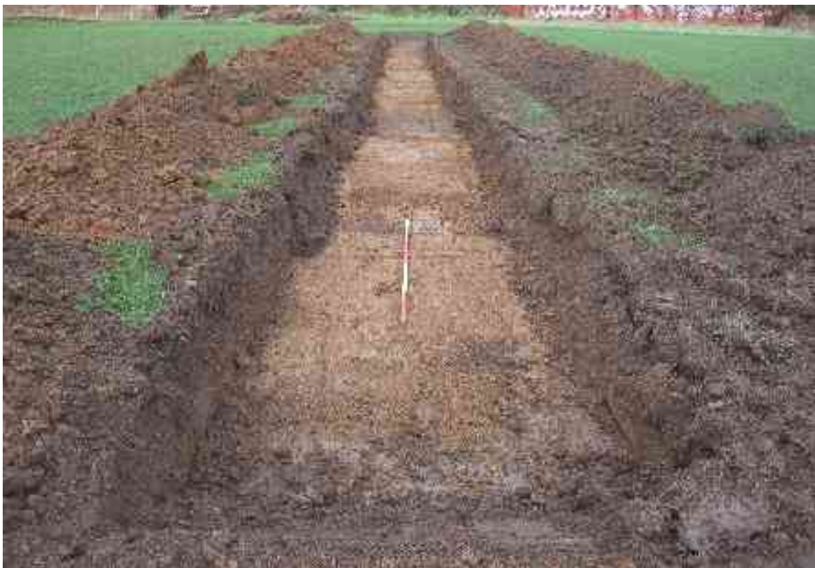
Fig 13 View of Trench 4 looking northwest
