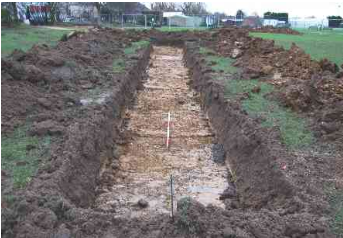
Fig 29 View of Trench 8 looking southeast
