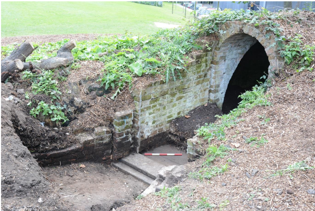
Fig.17: Southern wall (0.5m scale)
