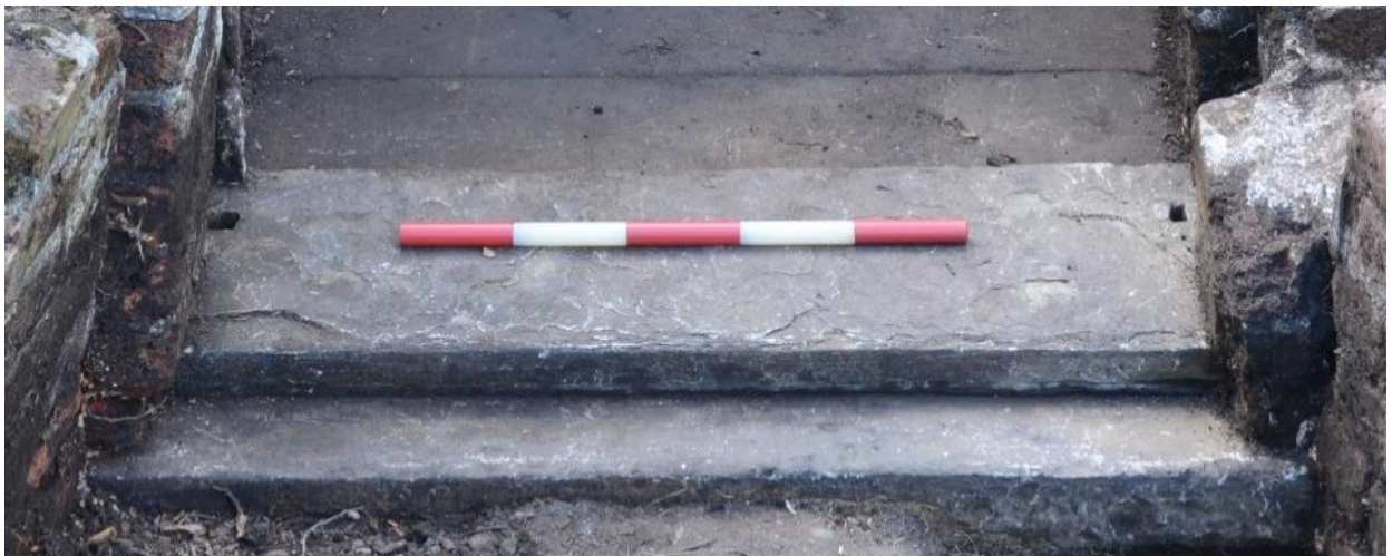
Fig.23: Stone threshold with mortises on either side, for door jambs (0.5m scale)
