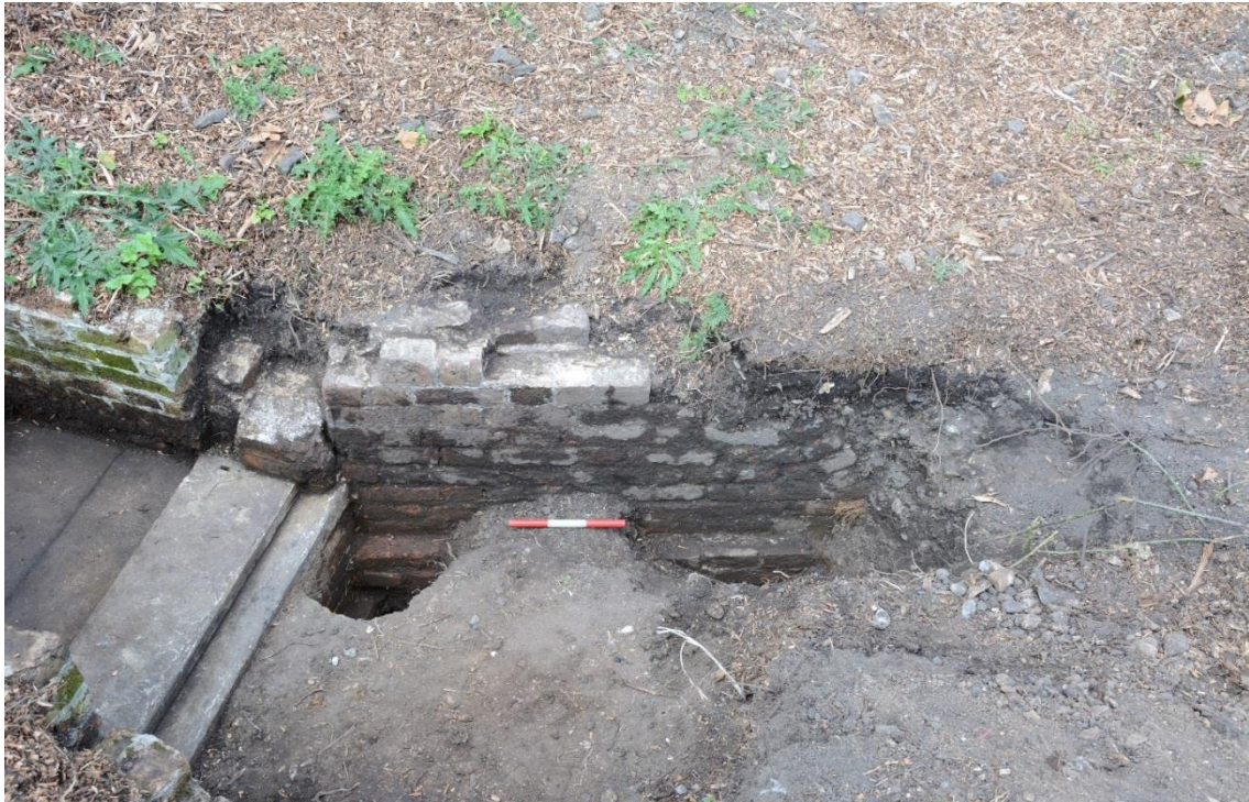
Fig.20: Test holes at the northern wall, outer part (0.3m scale)
