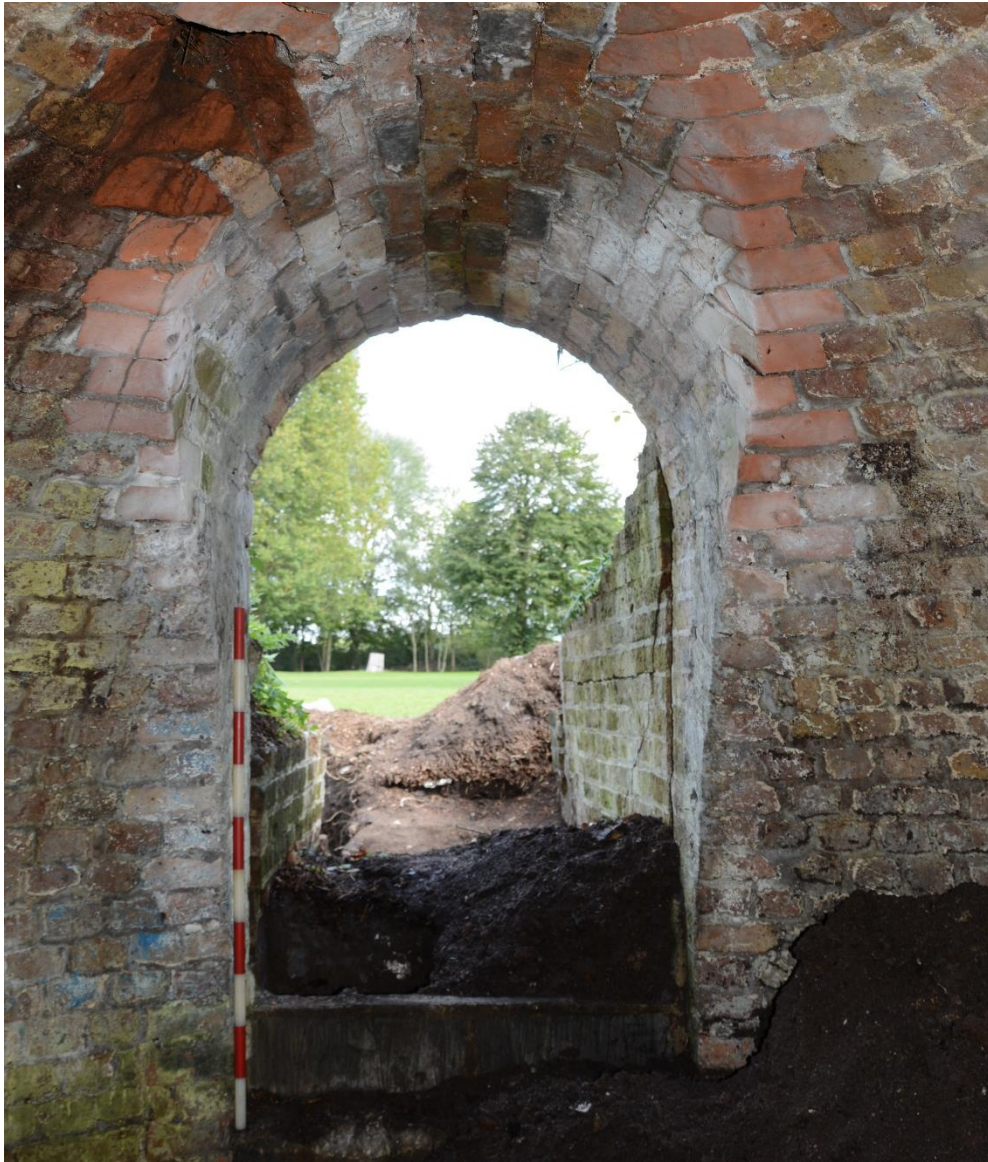
Fig.24: Base of a modern blocking wall and concrete foundation within the doorway (view from the ice house's interior, 1m scale).
