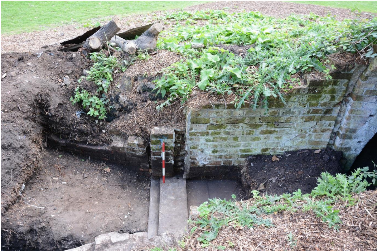
Fig.18:Southern wall (0.5m scale)
