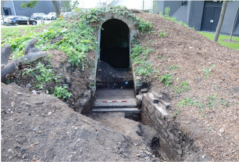
Fig.15: Exterior walls and pathway (0.5m scale)
