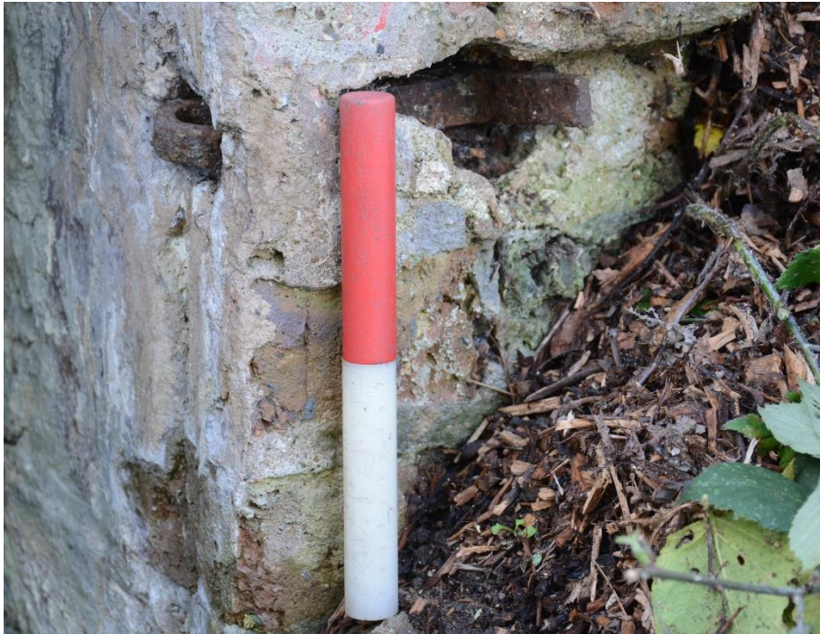
Fig.25: An iron hinge on upper right hand side of the entrance (0.2m scale)
