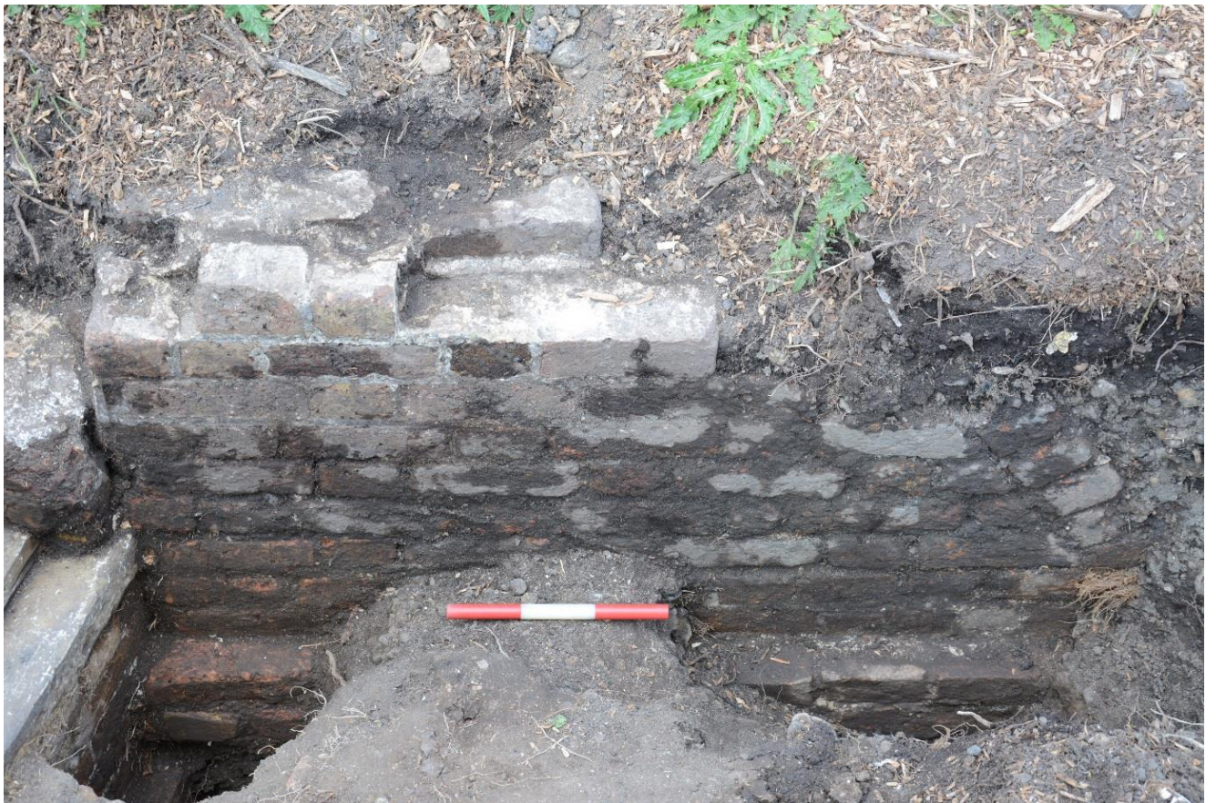
Fig.21: Test holes at the northern wall- detail (0.3m scale)
