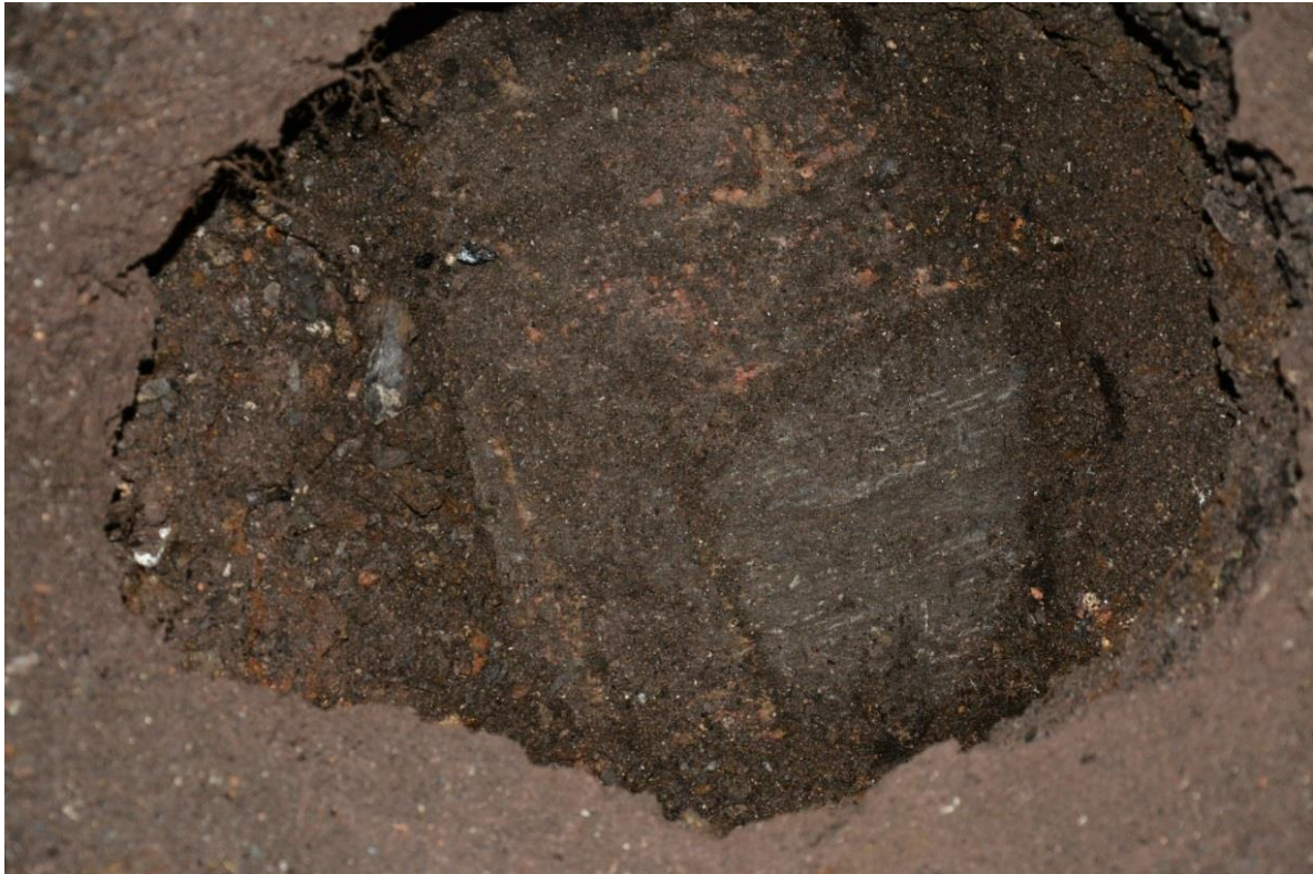
Fig.12: A test pit exposing the brick floor inside the ice house
