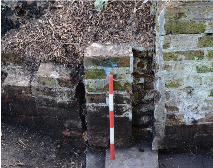
Fig.22: Rebate for a door jamb in the southern wall- close up (0.5m scale)
