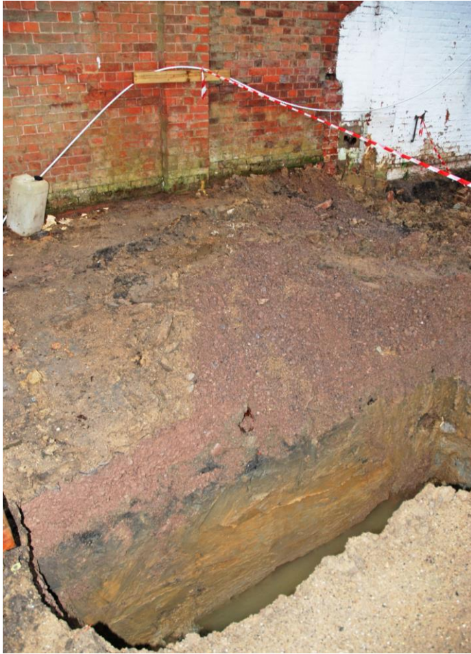
Fig.27: A section of E-W foundation trench adjoining the gardeners' bothy (to the left), with truncated subsoil overlain by modern crushed stone (MOT Type 1)
