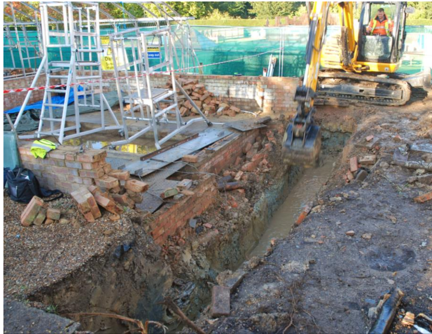
Fig.18: Excavation for the southern wall of the new cafe, facing SW
