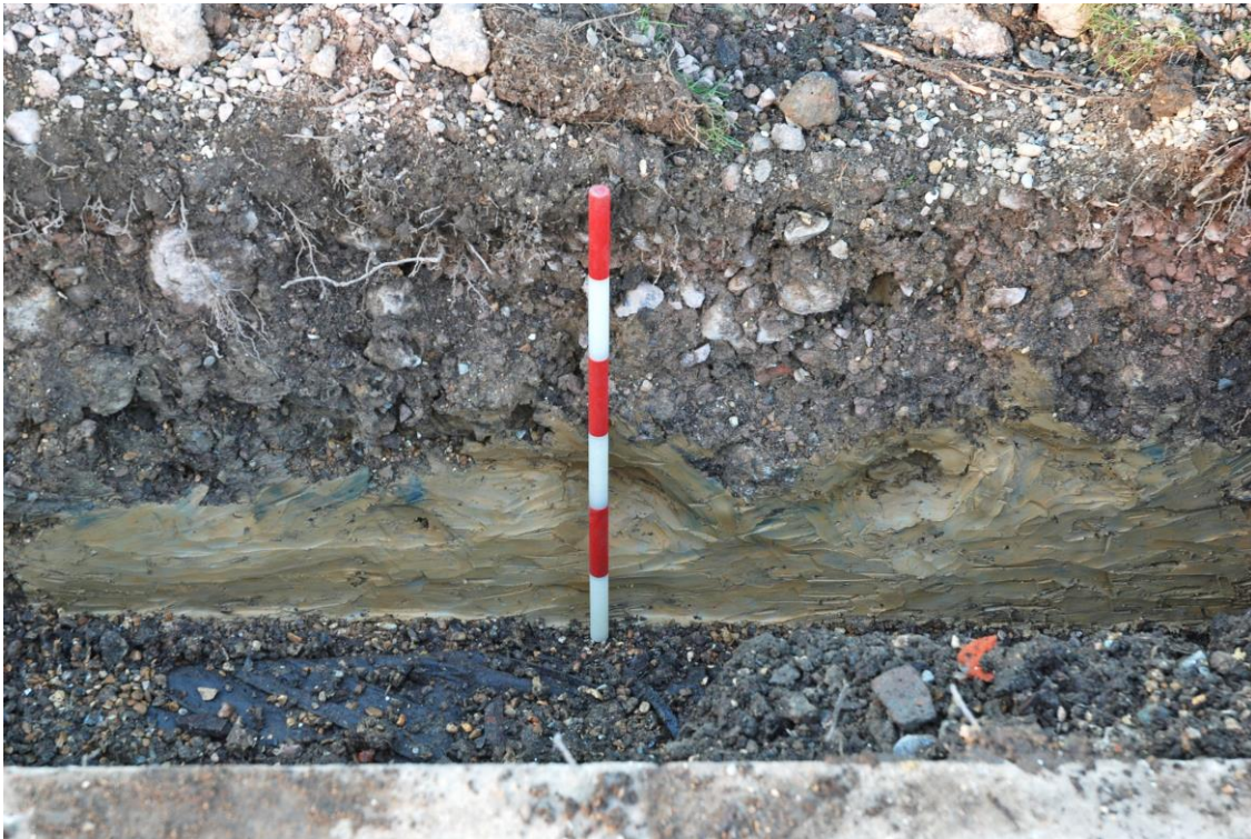
Fig.35: Part of the east-facing section of a new soakaway to the west of the Hardy House, and showing recent made ground directly over clean natural clay
