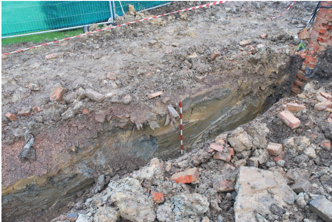
Fig.15: General view of the western foundation trench, looking northwest (1.0m scale). Previous soil horizons have been wholly removed, and the truncated surface overlain with a mixture of modern building rubble, gravel and crushed stone (MOT Type 1)
