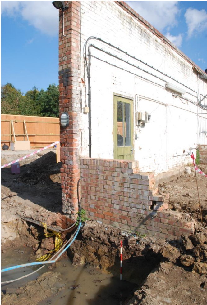
Fig.16: The western end of the spine wall, following demolition of the glasshouses to north and south and prior to excavation of the new foundations
