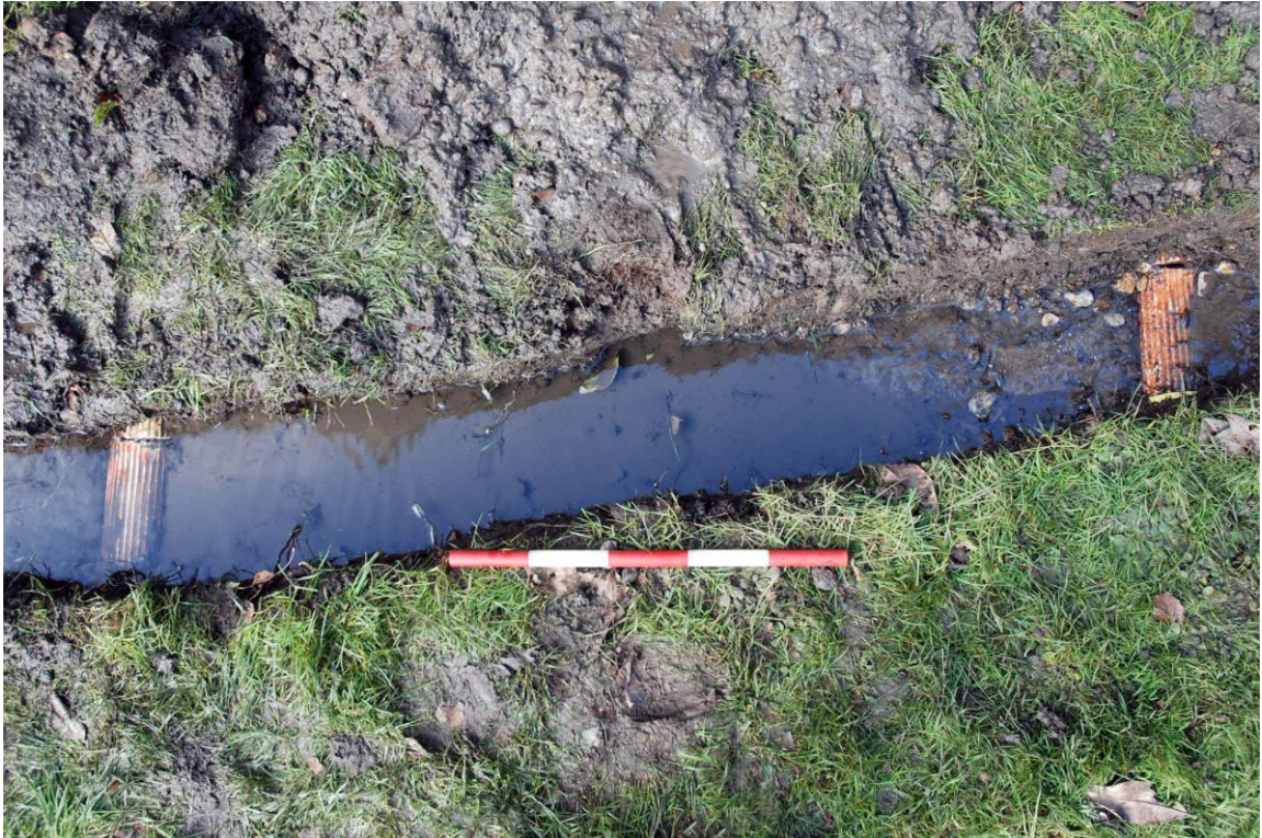
Fig.66: Parallel ceramic land drains running alongside the moat: view from above with NW to top of the frame (0.50m scale)
