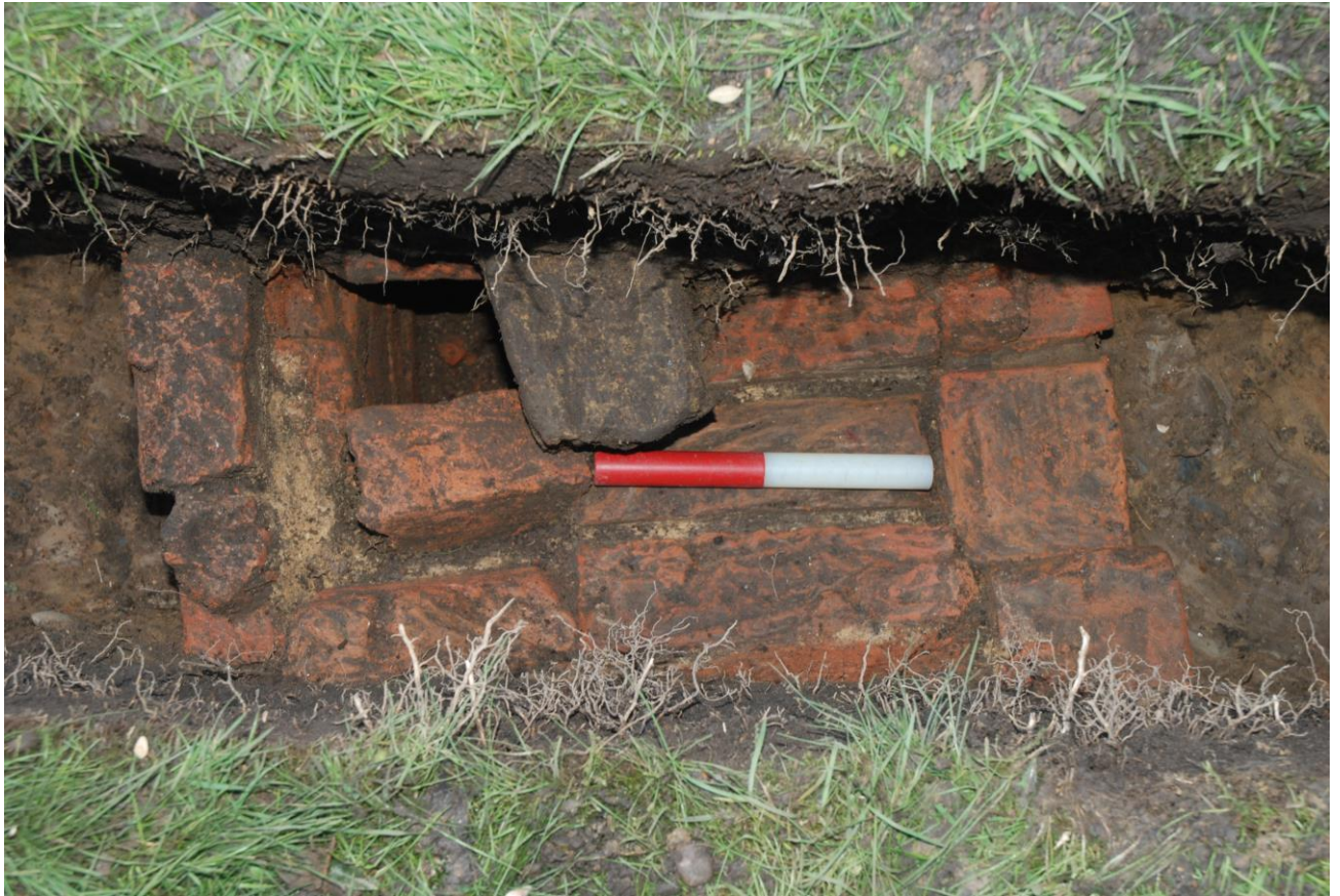
Fig.56: Brick-lined drain [14], overhead view with SW to top of frame, (0.20m scale)
