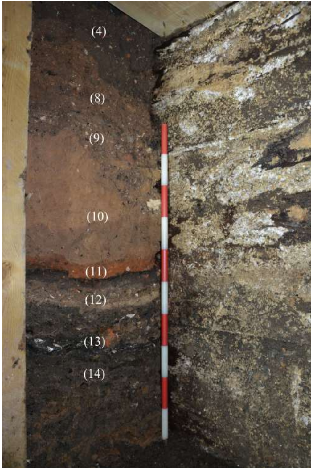
Fig.27: View of extension at base of the NW section of the shaft with context numbers added, facing SW. The main shaft is on the left, and modern concrete immediately to the right of the 1m scale
