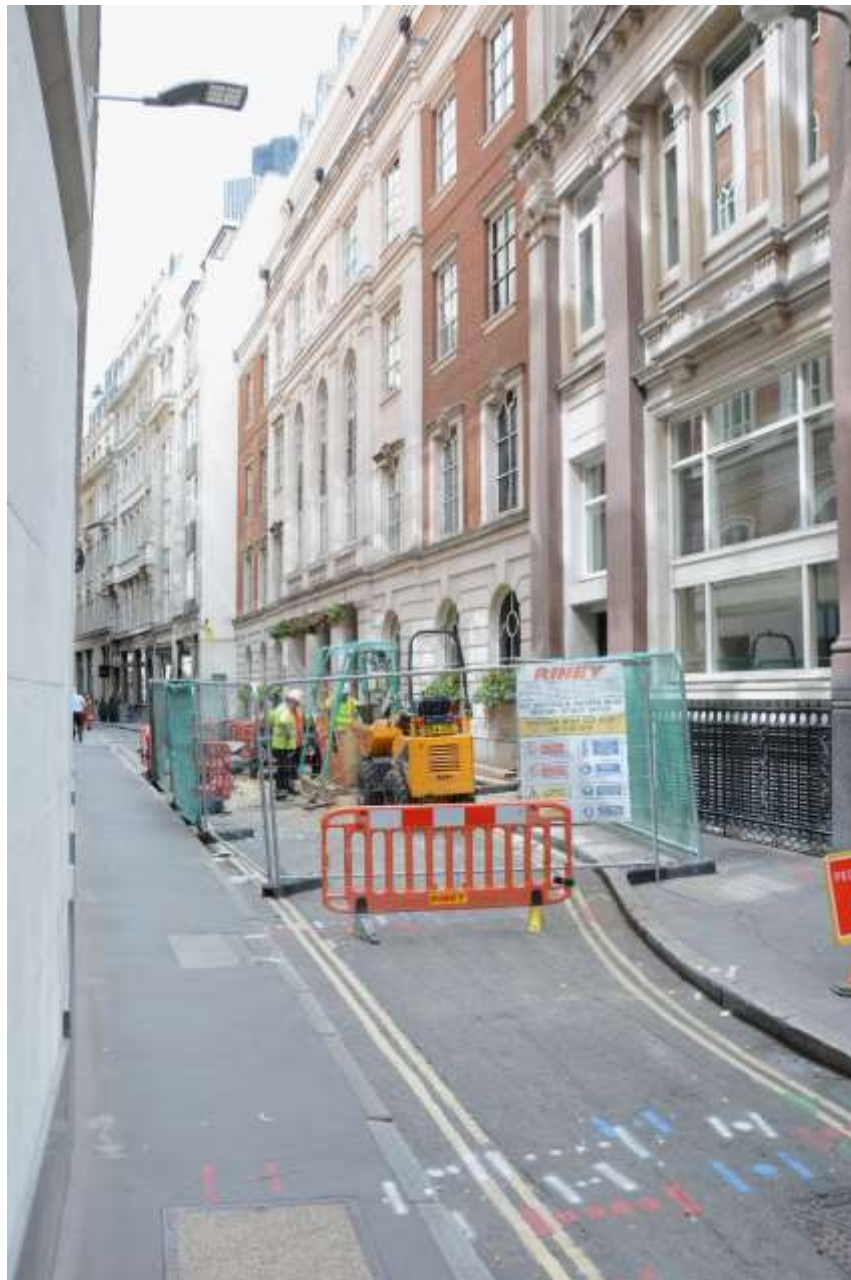
Fig. 11: View of site location on Birchin Lane, facing N
