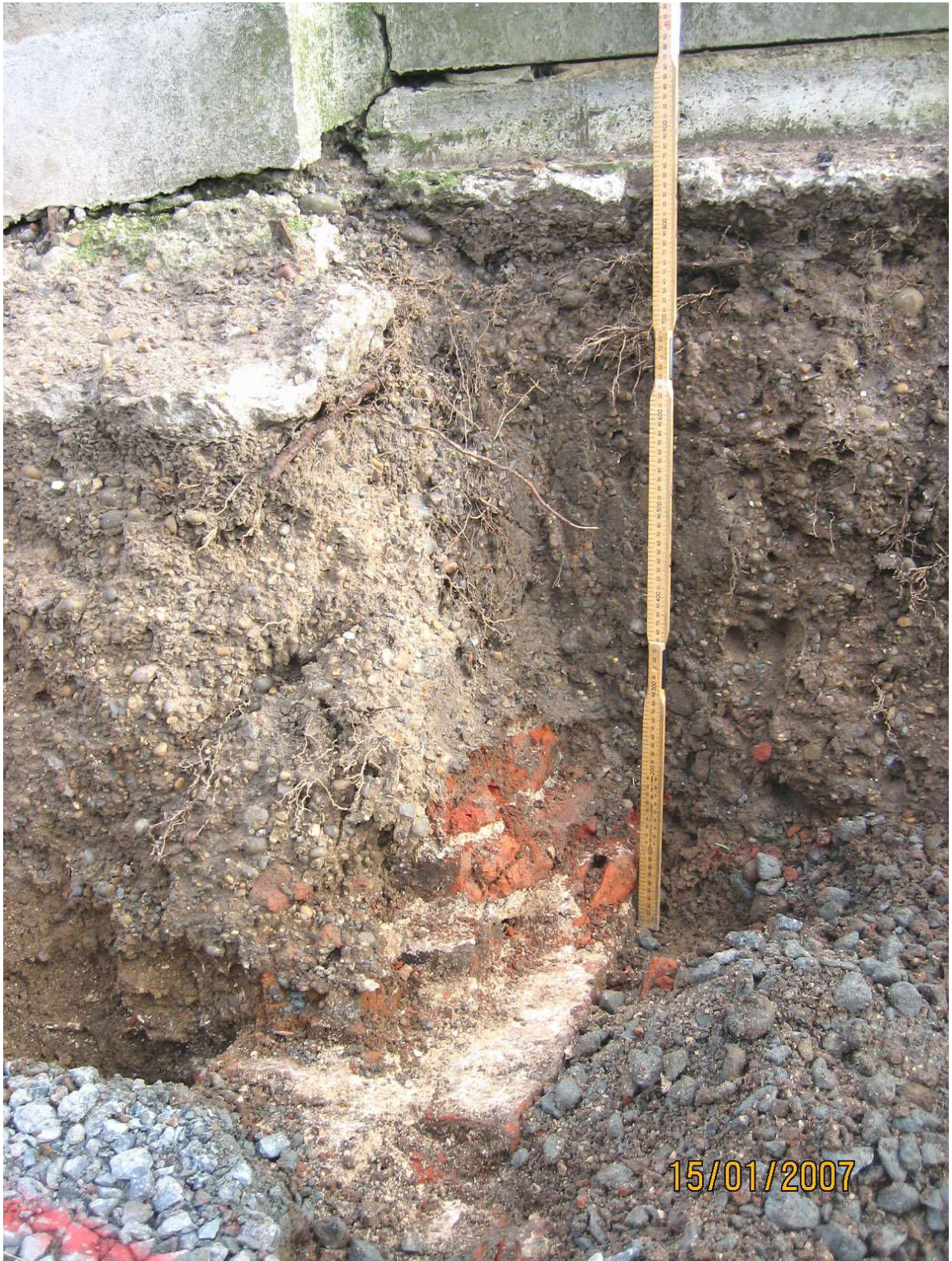
Fig 4 Detailed view of the brick wall base and adjacent deposits
