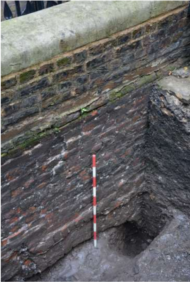
Figure 19: Detail of arch. The division between the two phases can be seen. There is a small scar to the left of the scale - purpose unknown. Facing north-east.
