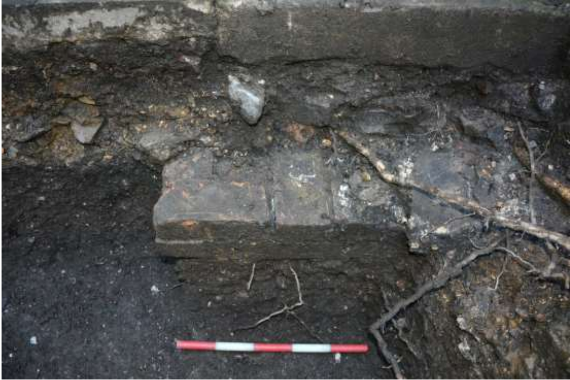
Figure 22: post-medieval brick drain structure at west end of pit. Facing west.
