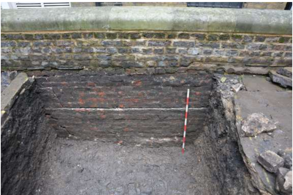
Figure 16: Existing churchyard wall. Facing north.
